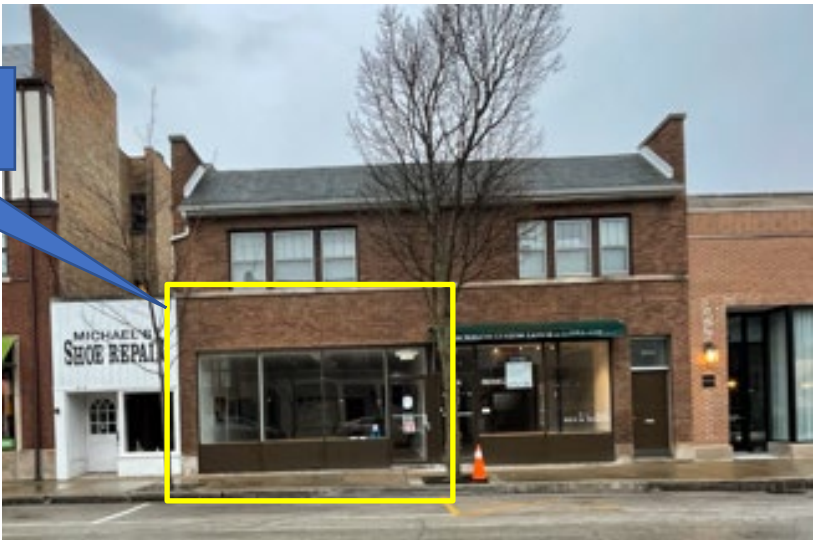
Figure 2 – Subject Property Lunk + Hancy – Storefront Location
