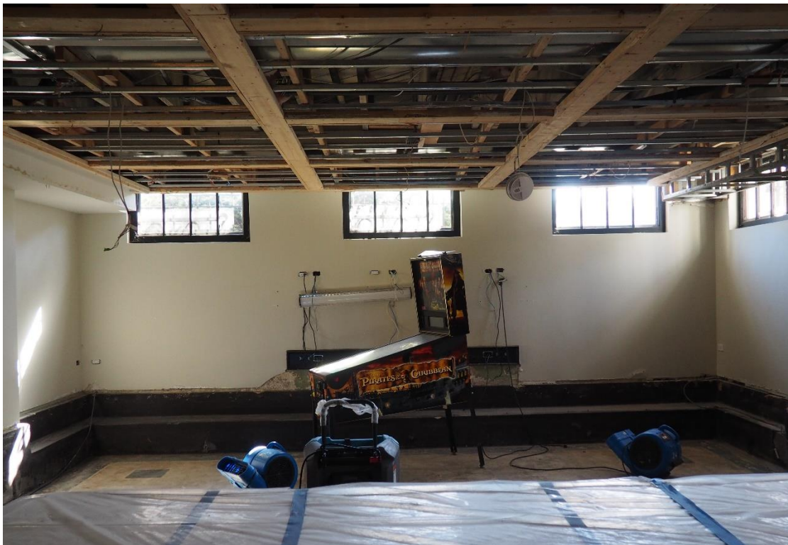
Photograph 14: View of the sunken recreation room, 2024. Source: McGuire Igleski & Associates, Inc
