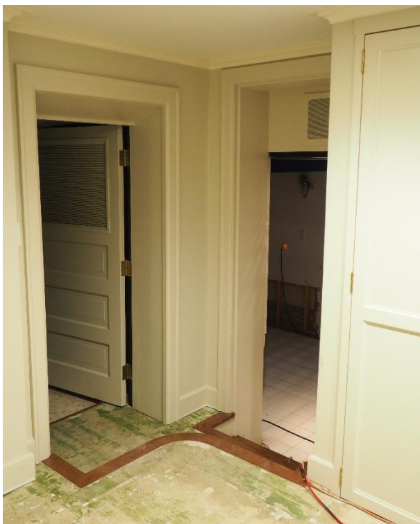
Photograph 25: View of the access to the basement storage areas, 2024. Source: McGuire Igleski & Associates, Inc. Note the storage rooms are sunken.
