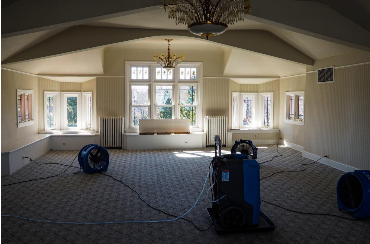
Photograph 70: Views of the former attic ballroom looking west, 2024. Source: McGuire Iglesias & Associates, Inc.
