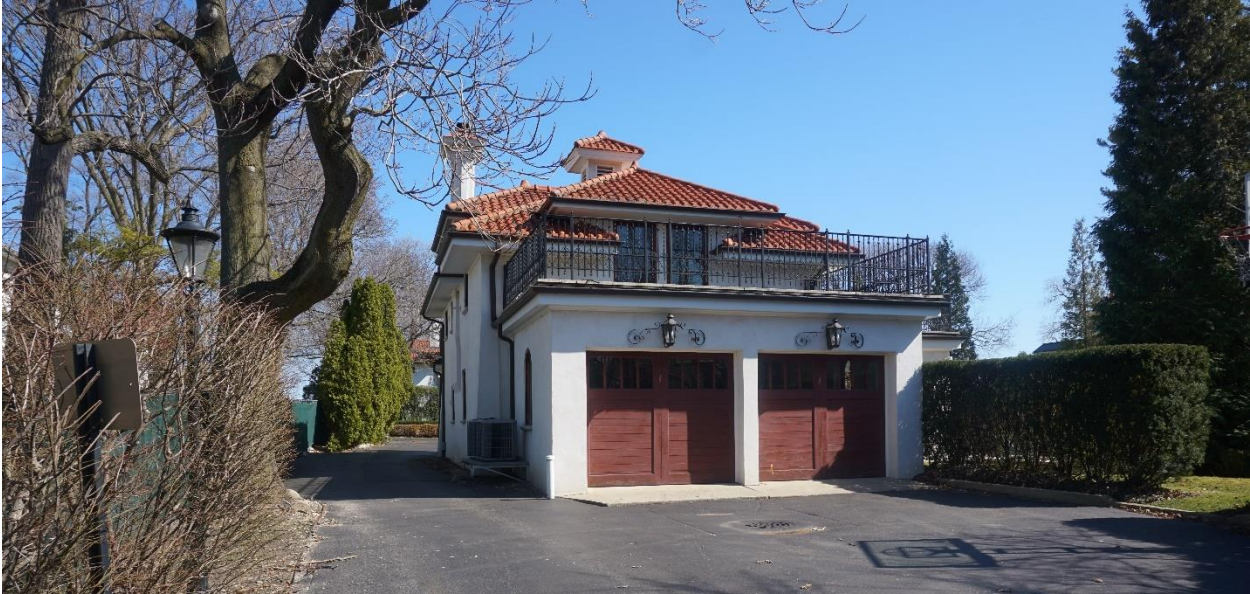
Photograph 79: View of the west and north elevations of the garage and pool house, 2024. Source: McGuire Iglesias & Associates, Inc.
