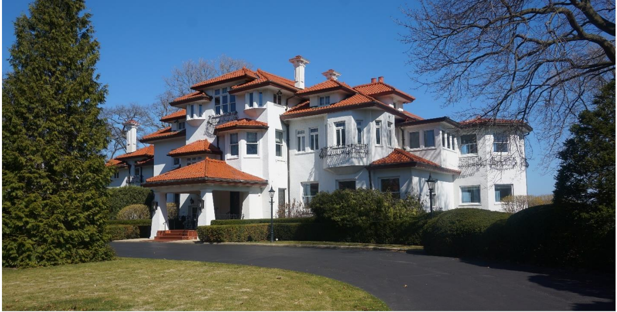
Photograph 3: View of the west façade looking north, 2024. Source: McGuire Igleski & Associates, Inc.
