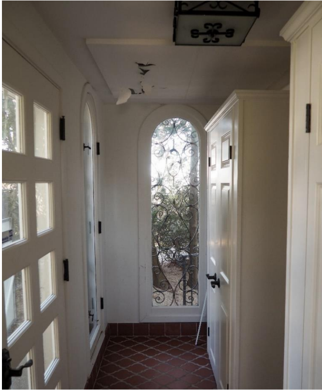
Photograph 56: View of the north entrance vestibule, 2024. Source: McGuire Igleski & Associates, Inc.
