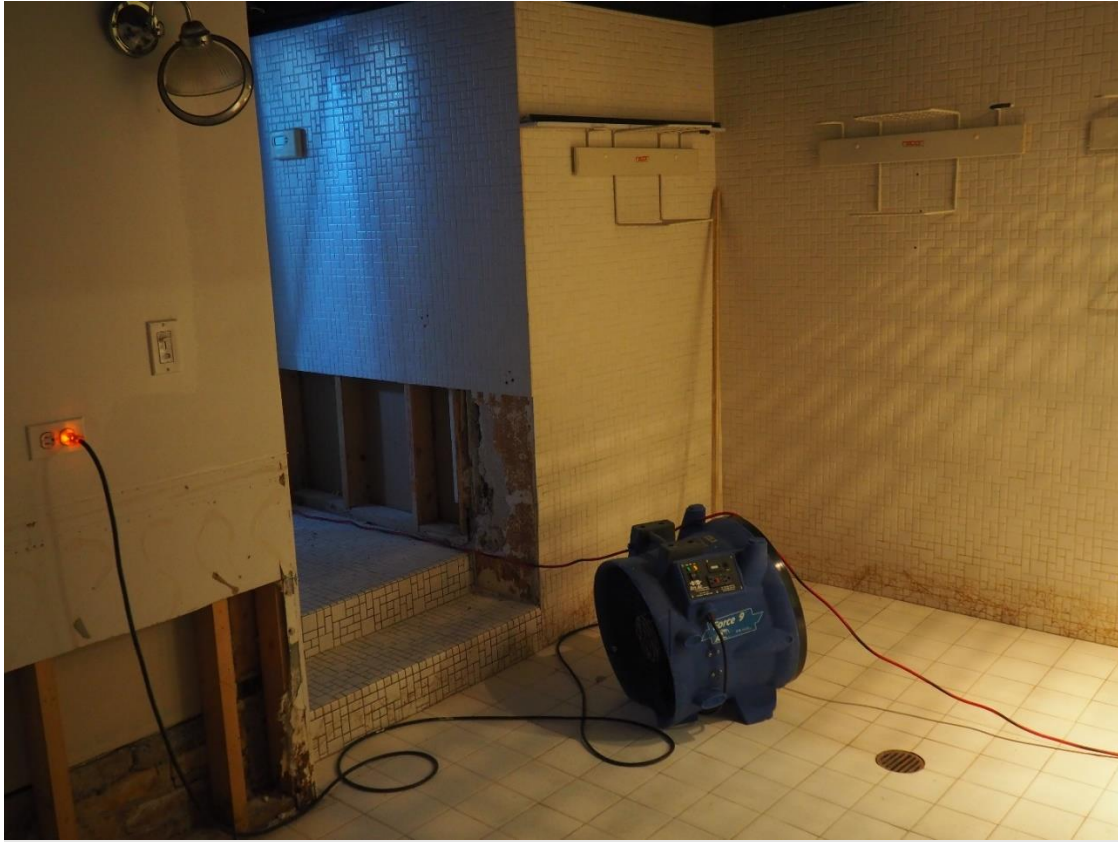
Photograph 26: View of the basement storage, 2024. Source: McGuire Igleski & Associates, Inc. This room was likely a “beach room” according to archival materials.
