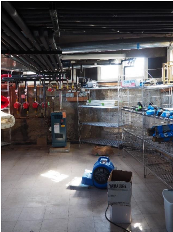
Photograph 27: View of the basement storage, 2024. Source: McGuire Igleski & Associates, Inc.
