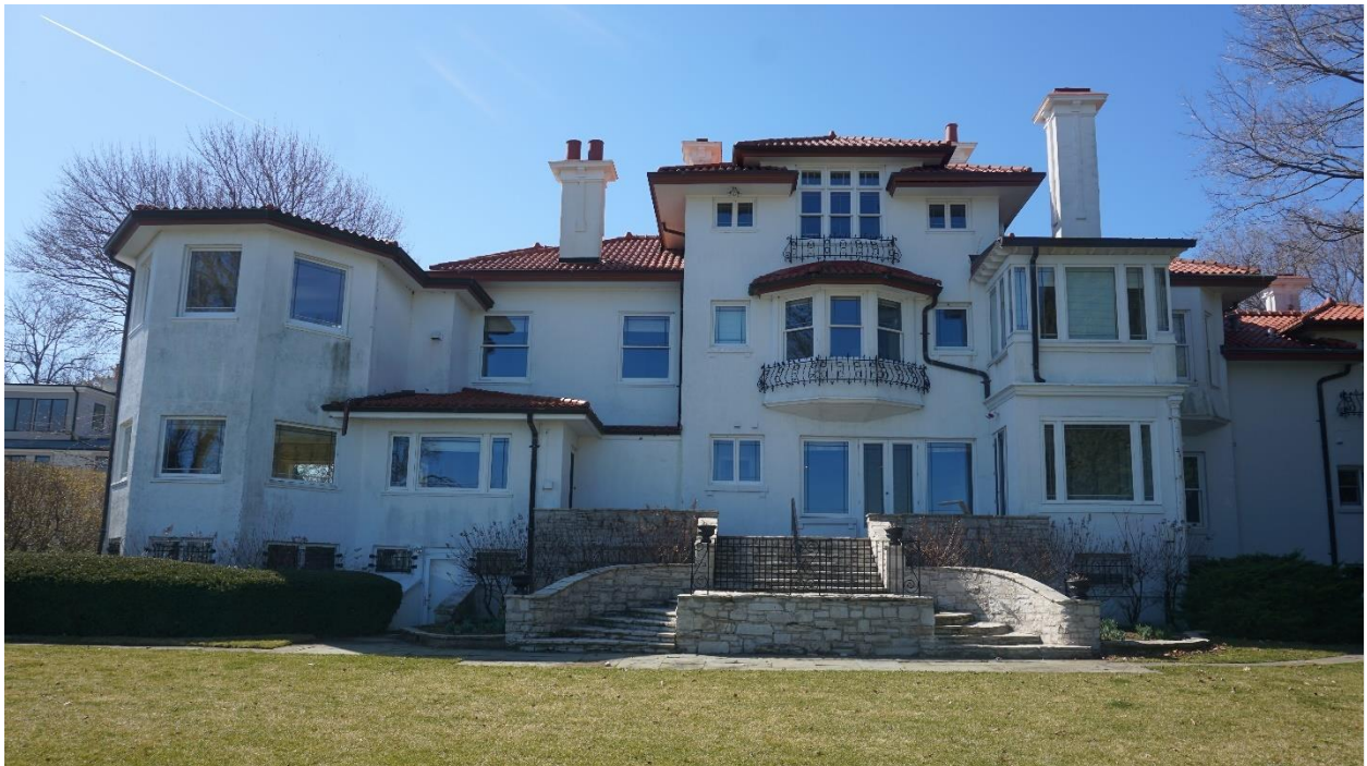
Photograph 8: View of the east façade looking west, 2024. Source: McGuire Igleski & Associates, Inc.
