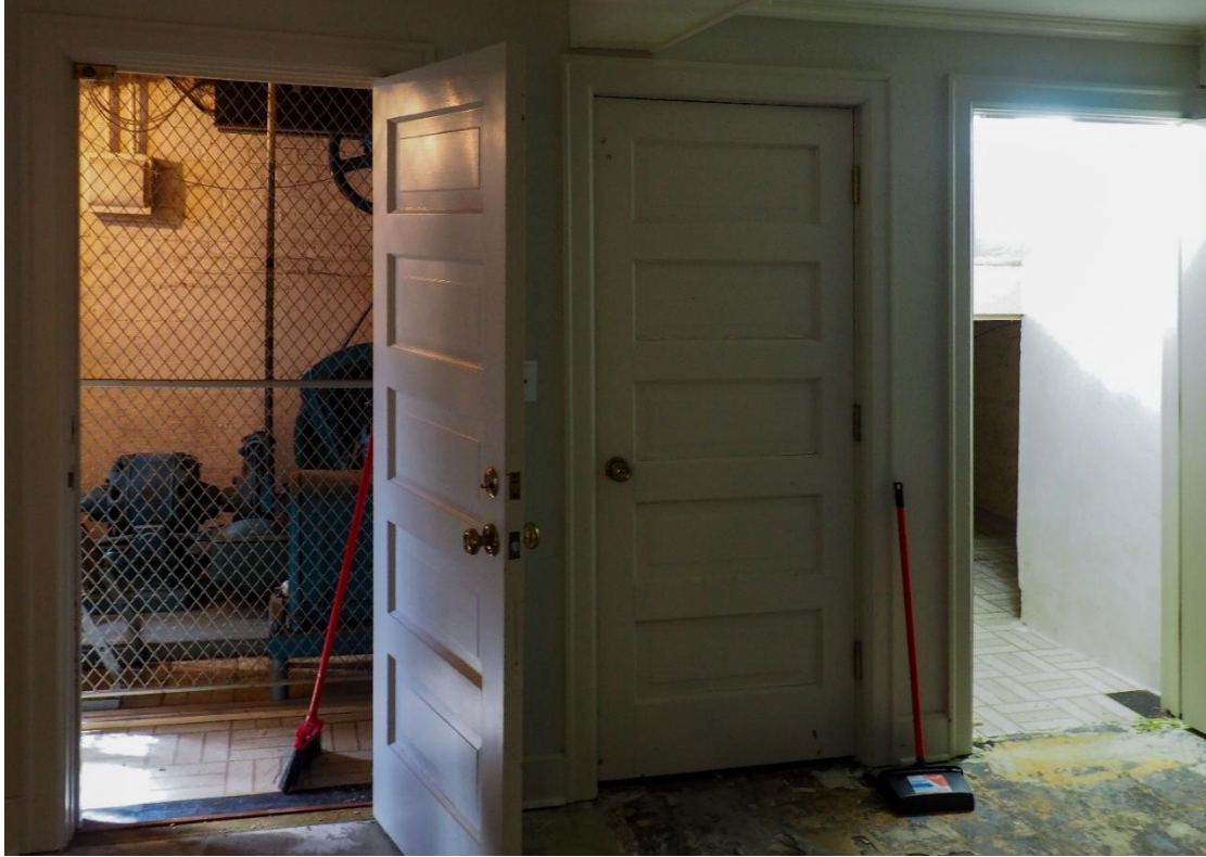
Photograph 13: View of the elevator control room and closets, 2024. Source: McGuire Igleski & Associates, Inc.
