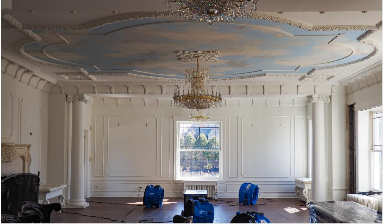
Photograph 38: View of the living room looking south, 2024. Source: McGuire Iglesias & Associates, Inc.
