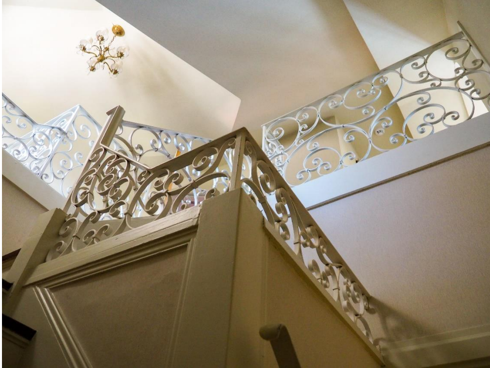
Photograph 67: View ascending the stairs to the attic level, former ballroom, 2024. Source: McGuire Igleski & Associates, Inc.
