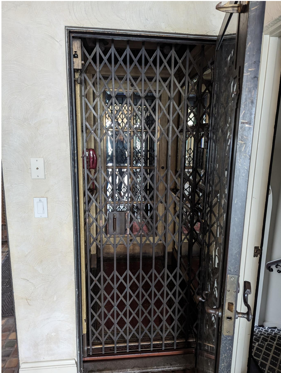
Photograph 72: Elevator Company of America entrance from the first floor entrance hall. The Oscar Bruno Bach-designed door is open, and the scissor door is closed. Source: McGuire Igleski & Associates, Inc.
