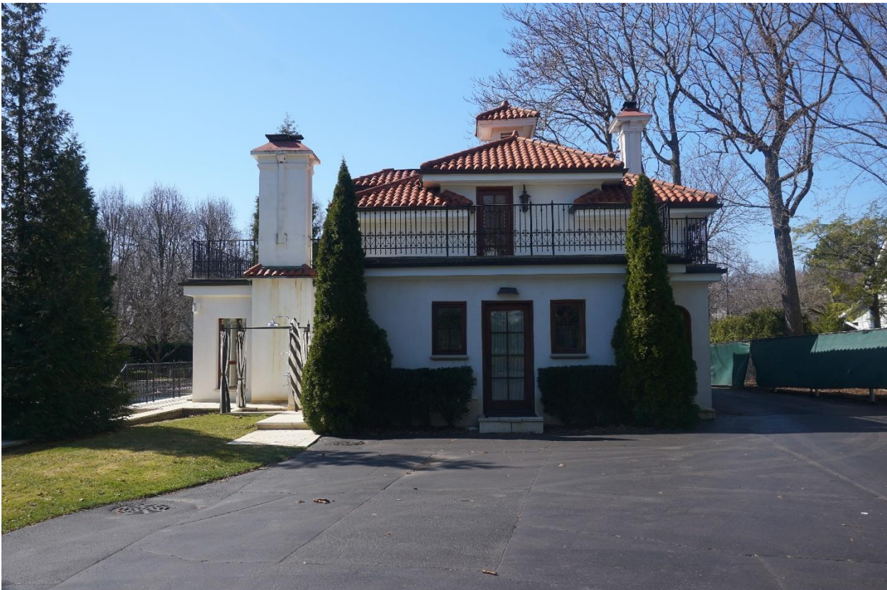
Photograph 80: View of the east elevation of the garage and pool house, 2024. Source: McGuire Iglesias & Associates, Inc.
