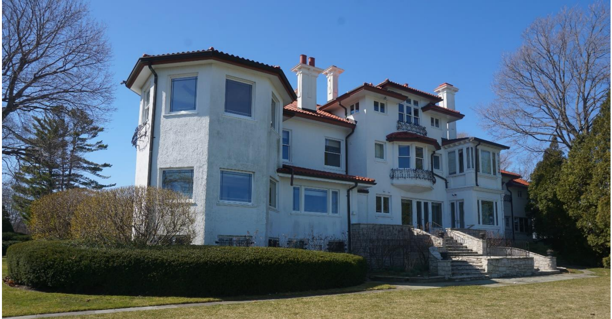
Photograph 7: View of the east façade looking northwest, 2024. Source: McGuire Igleski & Associates, Inc.
