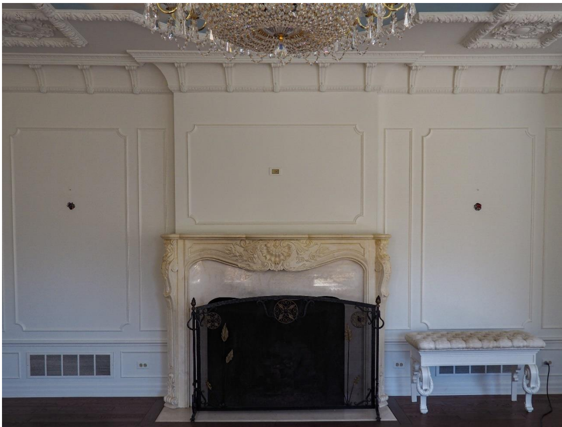
Photograph 42: View of the living room looking east, 2024. Source: McGuire Igleski & Associates, Inc.
