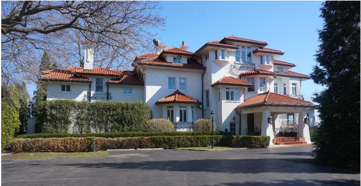
Photograph 1: View of the west façade looking east, 2024. Source: McGuire Igleski & Associates, Inc.
