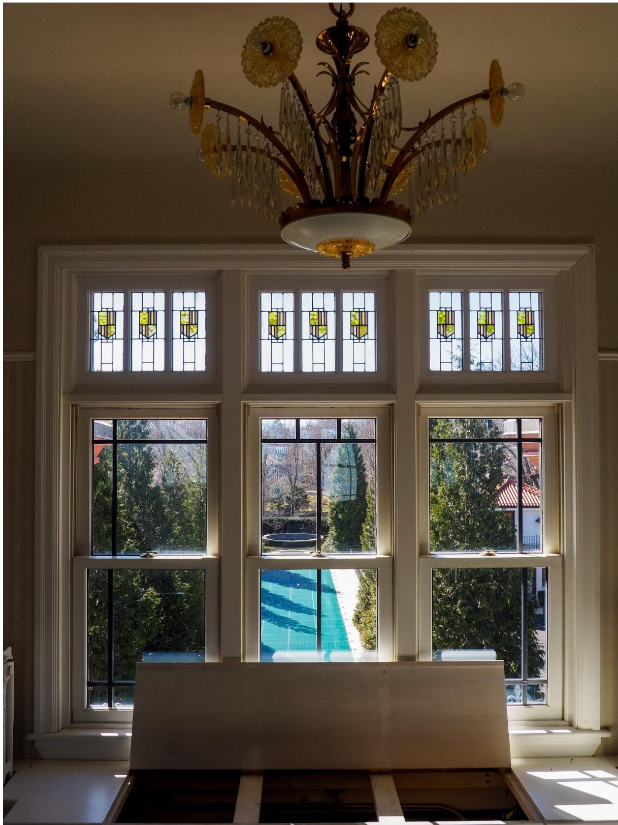
Photograph 71: Detail of the attic stained glass looking toward the pool to the west, 2024. Source: McGuire Igleski & Associates, Inc.
