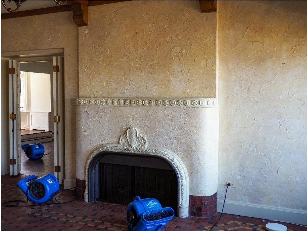
Photograph 30: View of the first floor entrance hall fireplace, 2024. Source: McGuire Igleski & Associates, Inc.
