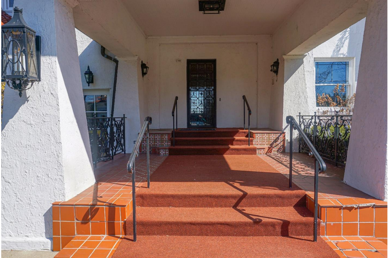
Photograph 5: Detail of the west façade entrance porch looking northeast, 2024. Source: McGuire Igleski & Associates, Inc.
