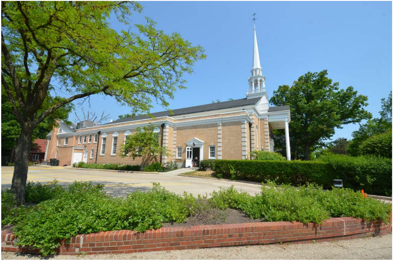
VIEW OF SOUTH FACADE
