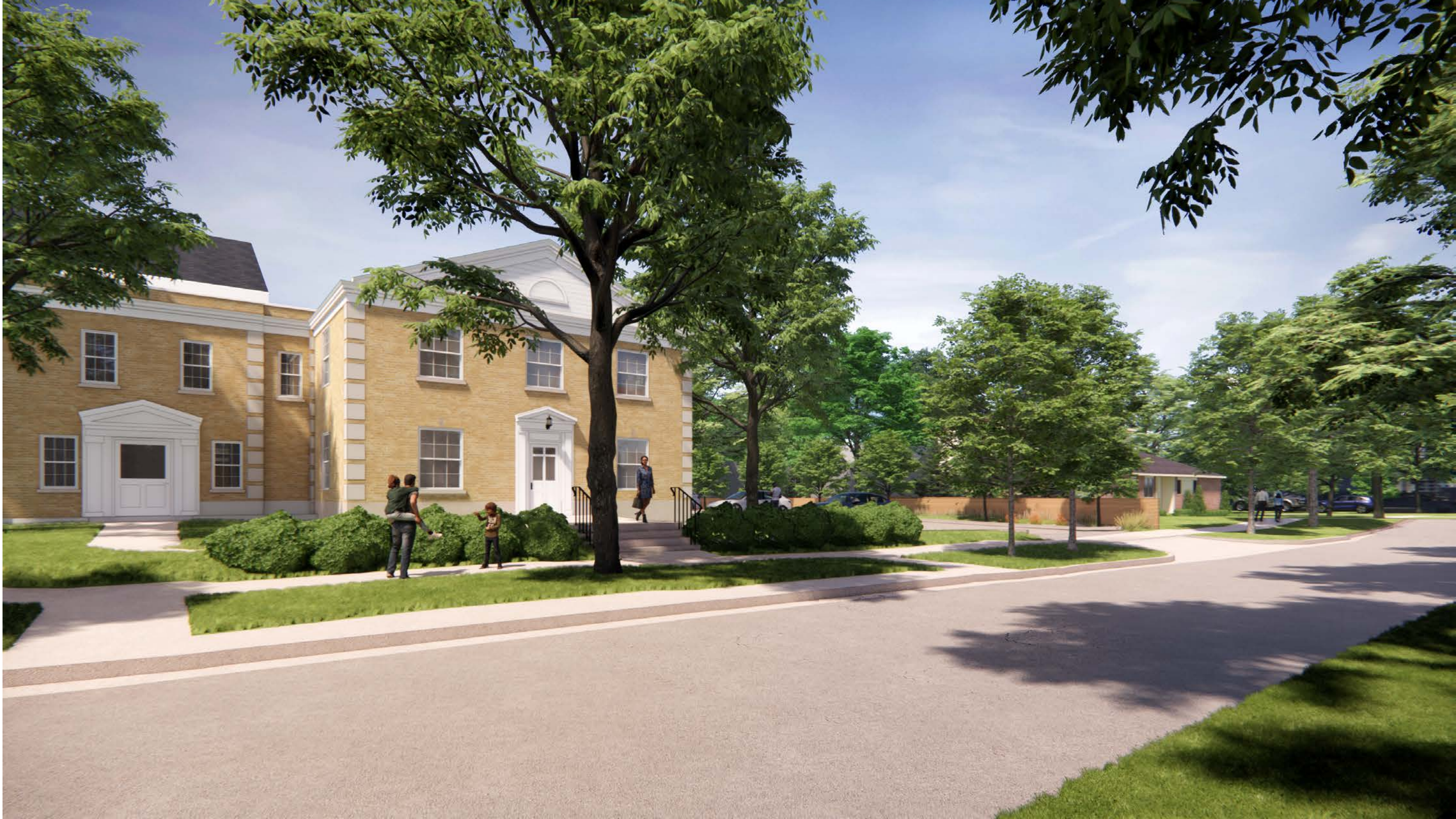
VIEW OF NORTH ADDITION FROM CHERRY STREET
