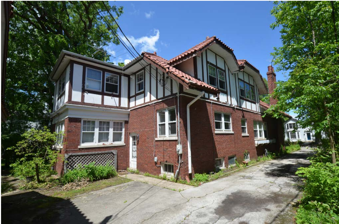
VIEW OF SOUTH & EAST FACADE
