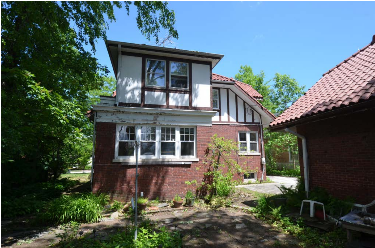
VIEW OF SOUTH FACADE
