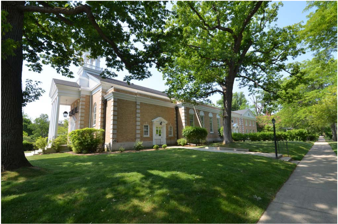
VIEW OF NORTH FACADE
