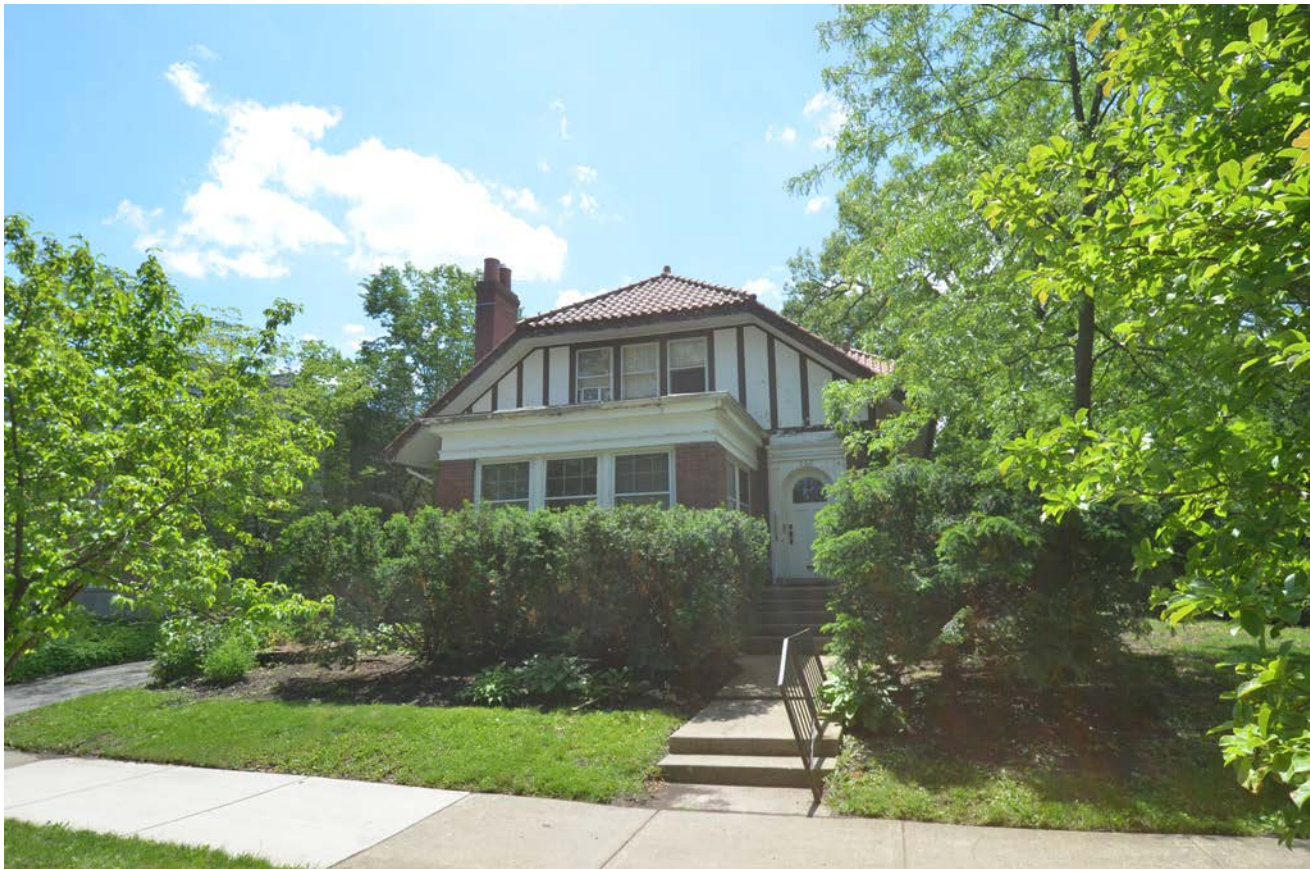
VIEW OF NORTH FACADE
