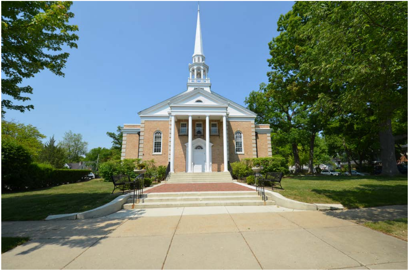
VIEW OF EAST FACADE
