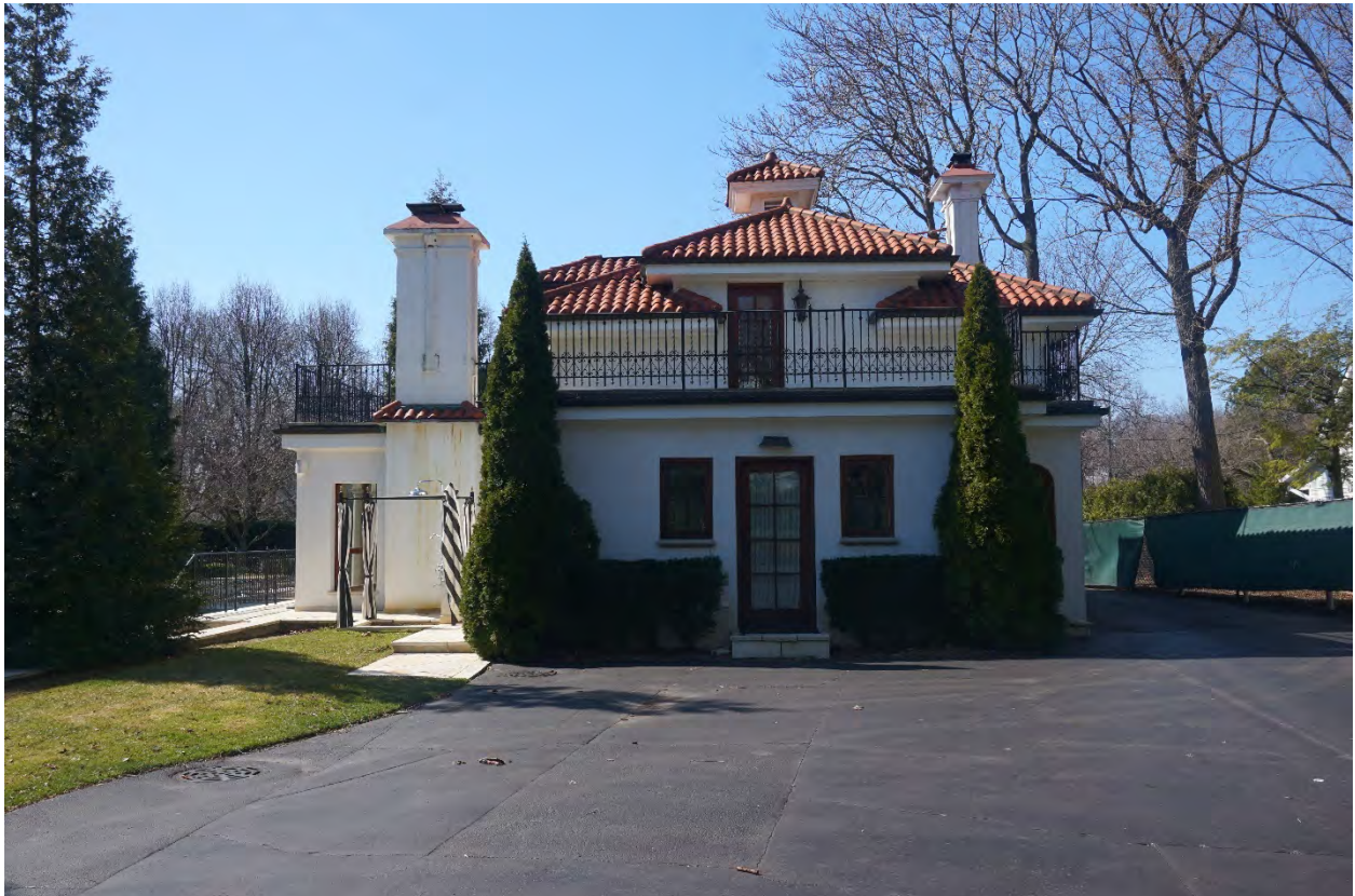
Photograph 82: View of the east elevation of the garage and pool house, 2024.
