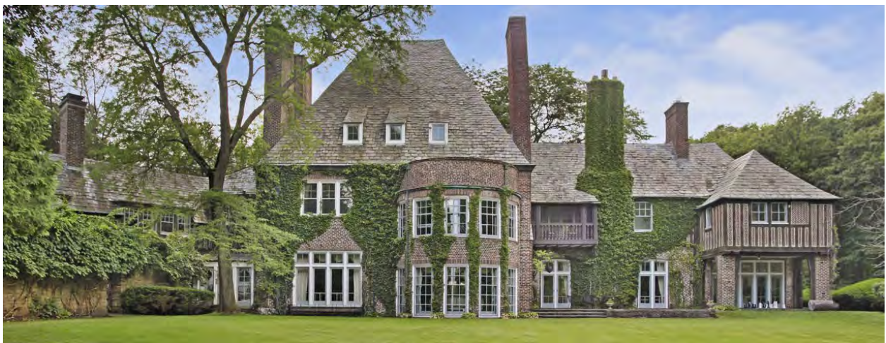
Figures 7-8: Oscar Bruno Bach designed doors on the Lake Forest, Illinois, residence Wyldwoode (architect Harrie T. Lindeberg, historic residence of Clyde Carr). Credit: VHT Studios, 2018.
