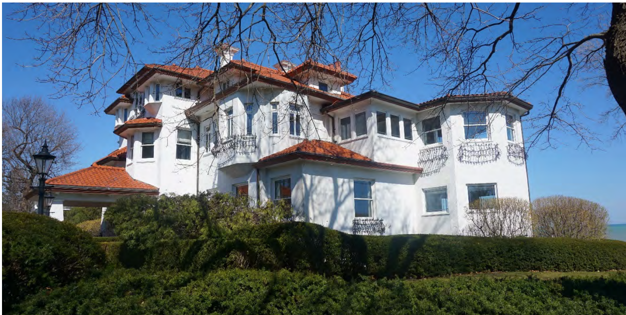
Photograph 6: View of the west and south façades looking north, 2024.
