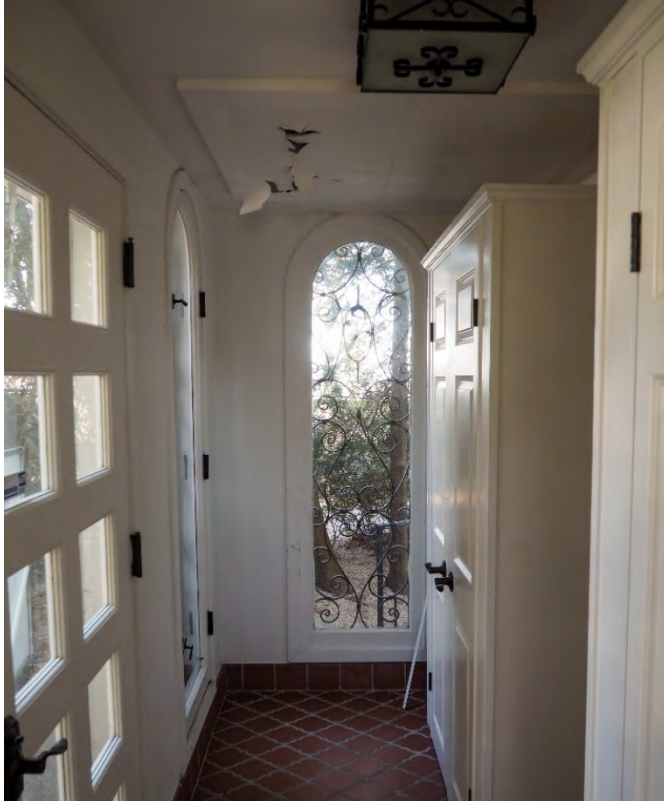
Photograph 58: View of the north entrance vestibule, 2024.
