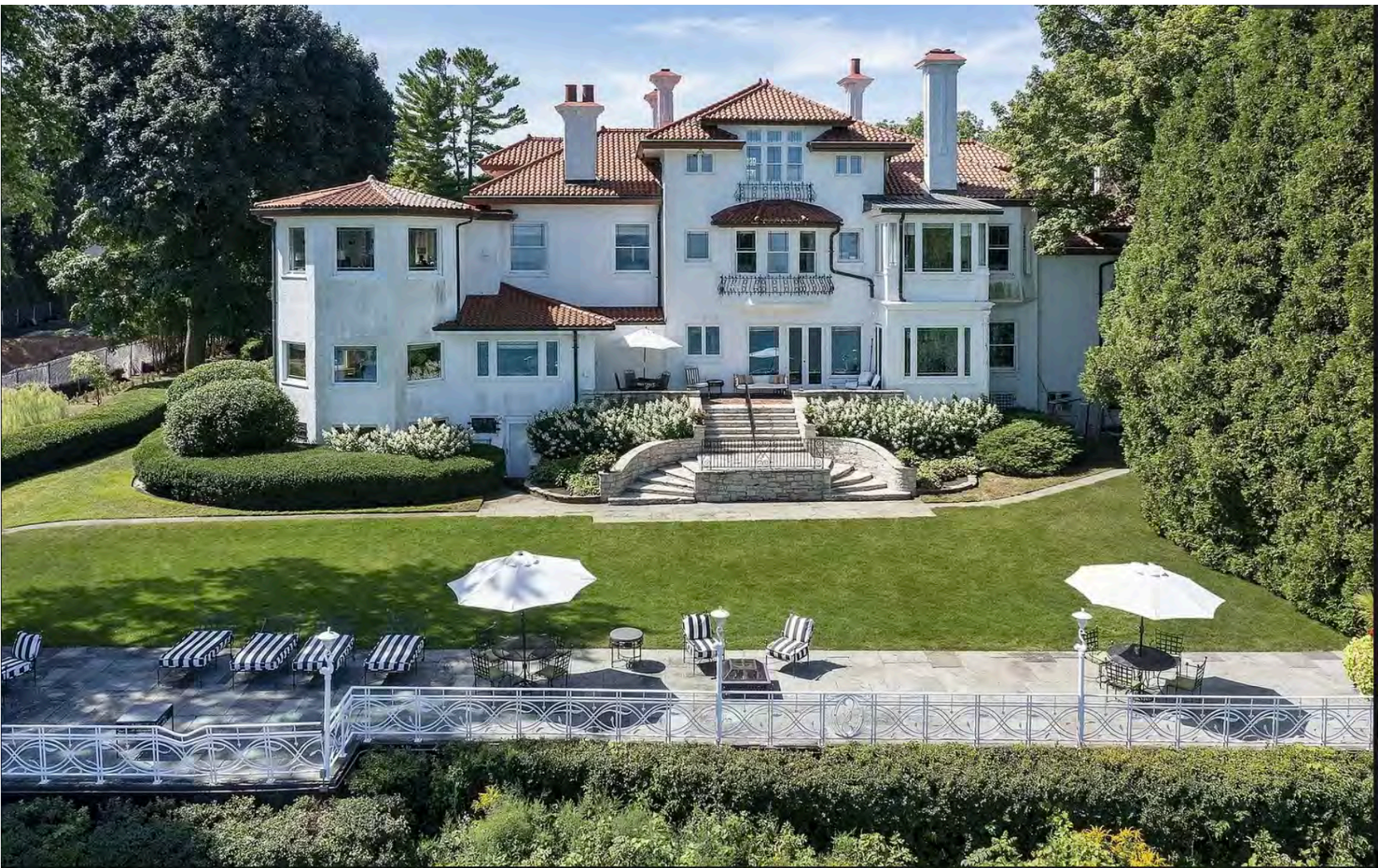
Photograph 4: View of the exterior rear façade, looking west; 2022.
