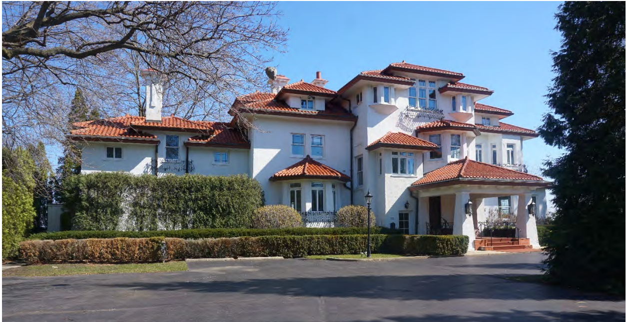
Photograph 1: View of the west façade looking east, 2024.
