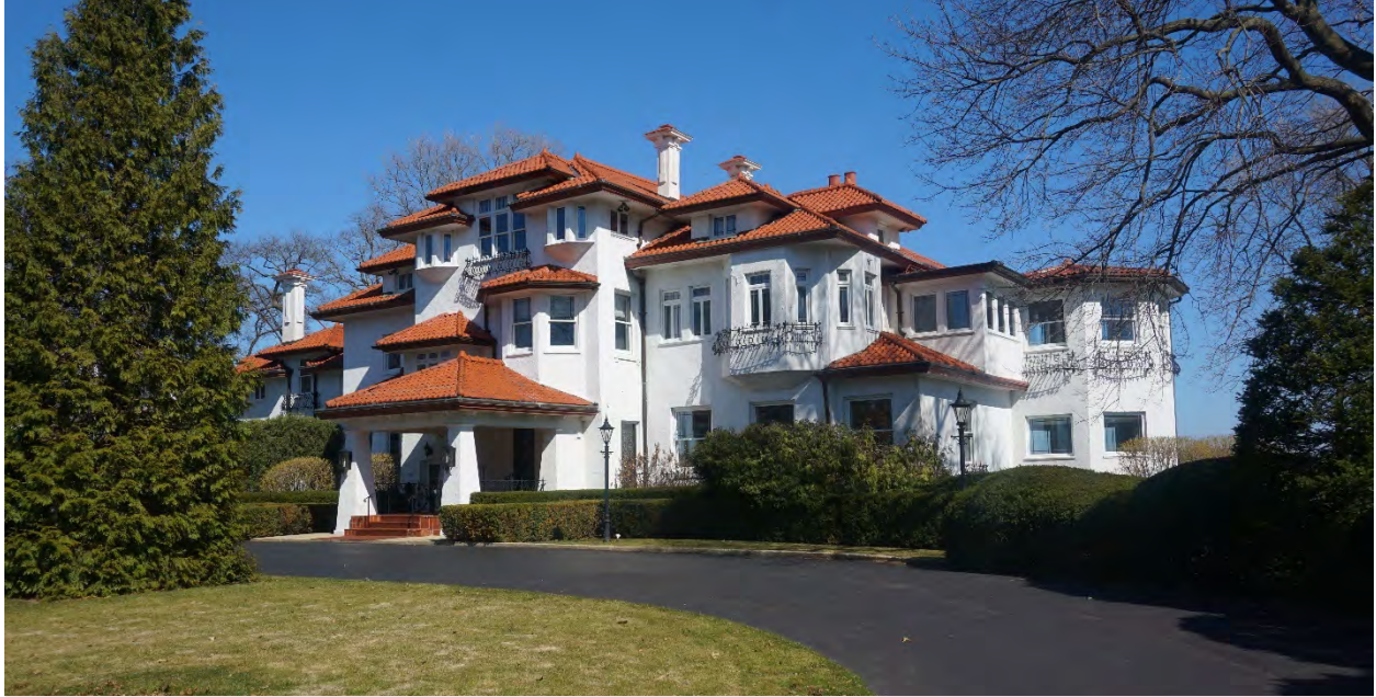
Photograph 3: View of the west façade looking north, 2024.
