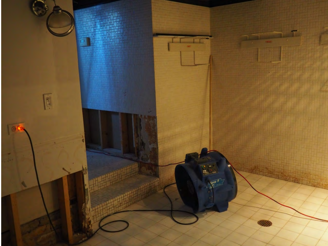
Photograph 27: View of the basement storage, 2024. This room was likely a “beach room” according to archival materials.
