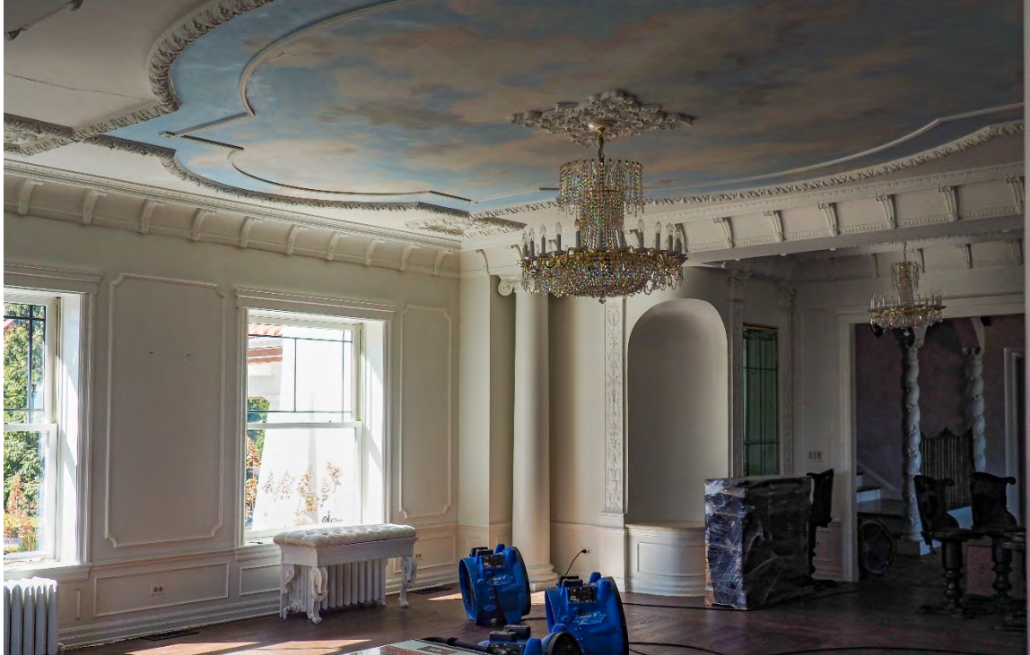
Photograph 42: View of the living room looking northwest, 2024.
