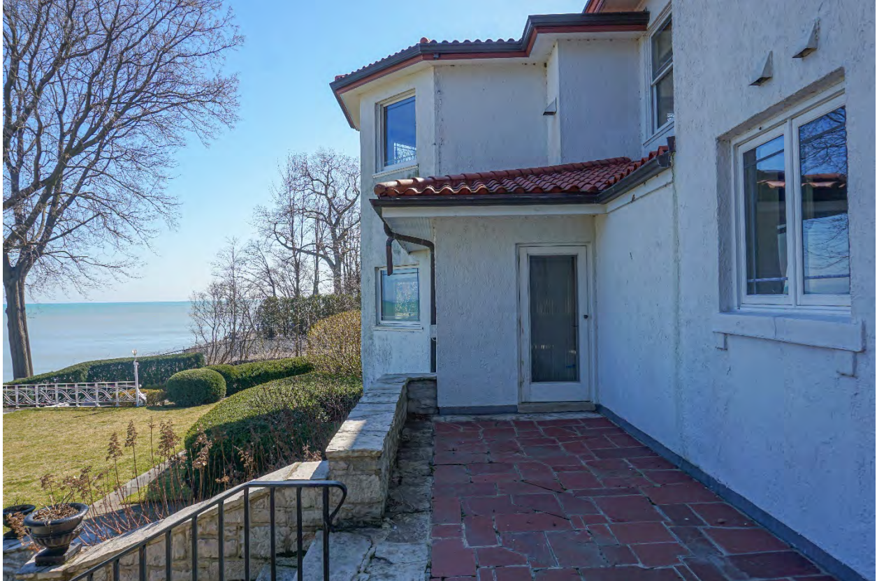
Photograph 9: Detail of the east patio and enclosed hexagonal porch looking south, 2024. Note the rear vestibule addition to the first floor, 1969.
