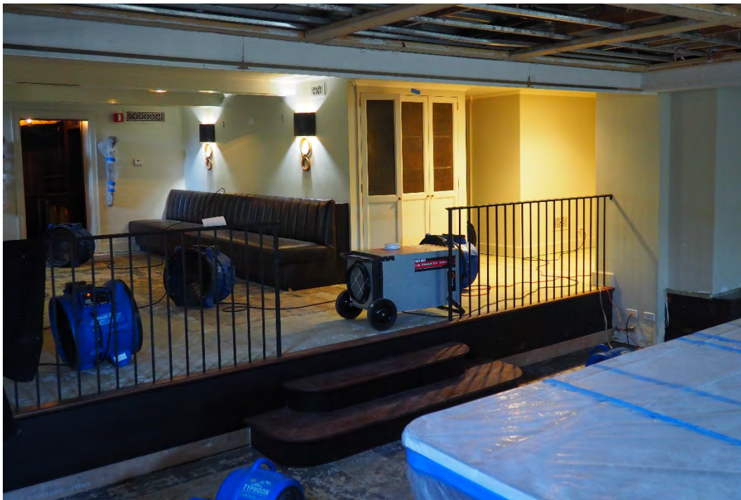
Photograph 23: View of the lounge from the sunken recreation room, looking northeast, 2024.
