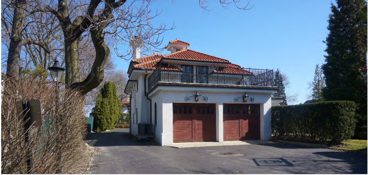
Photograph 81: View of the west and north elevations of the garage and pool house, 2024.
