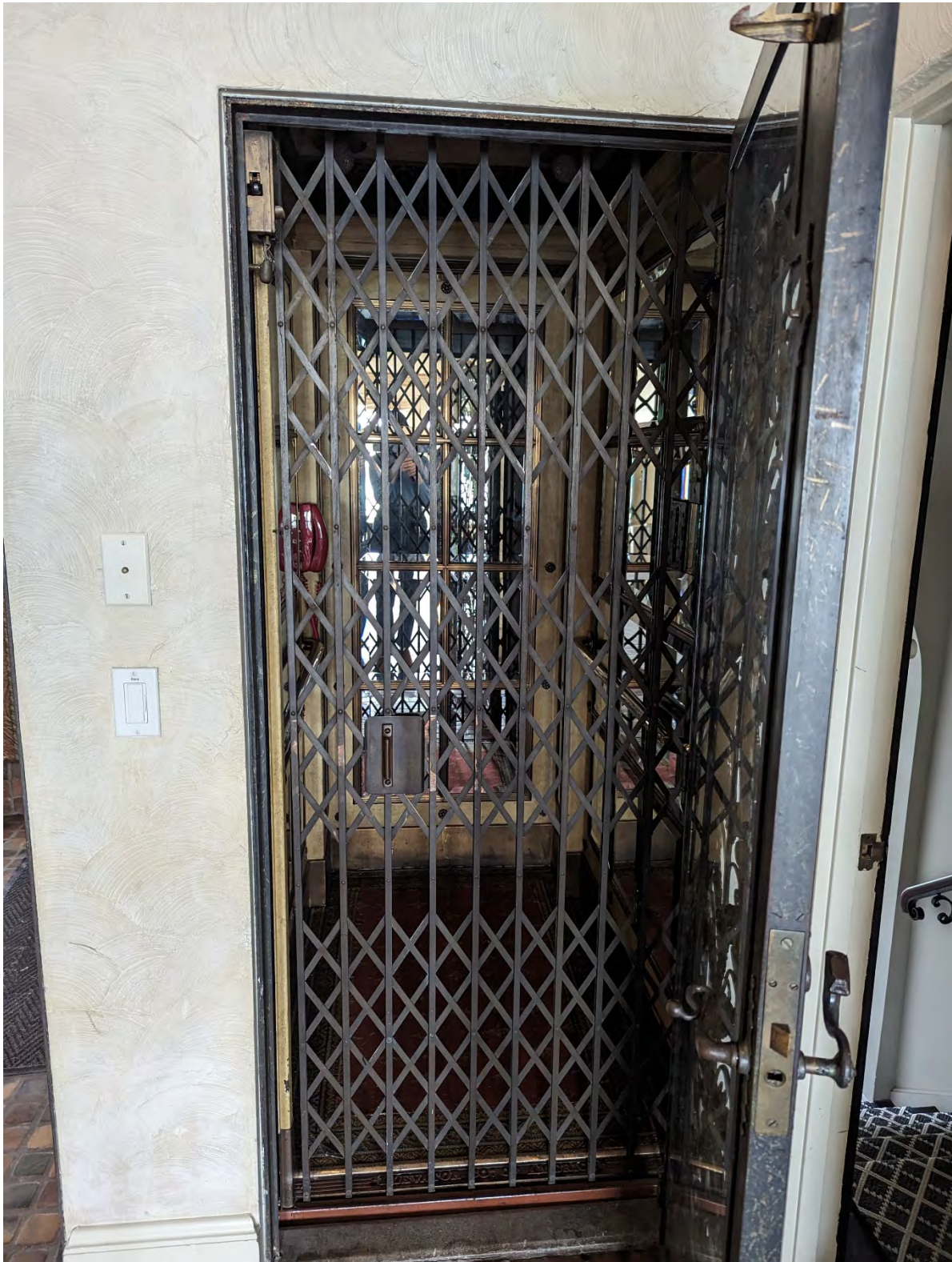
Photograph 74: Elevator Company of America entrance from the first floor entrance hall. The Oscar Bruno Bach-designed door is open, and the scissor door is closed.
