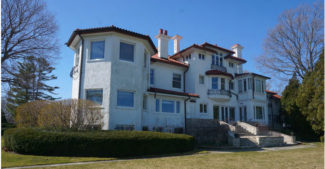
Photograph 7: View of the east façade looking northwest, 2024.
