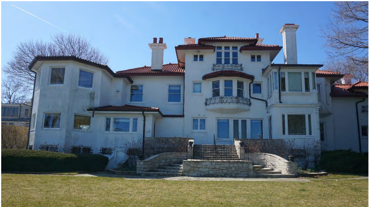
Photograph 8: View of the east façade looking west, 2024.
