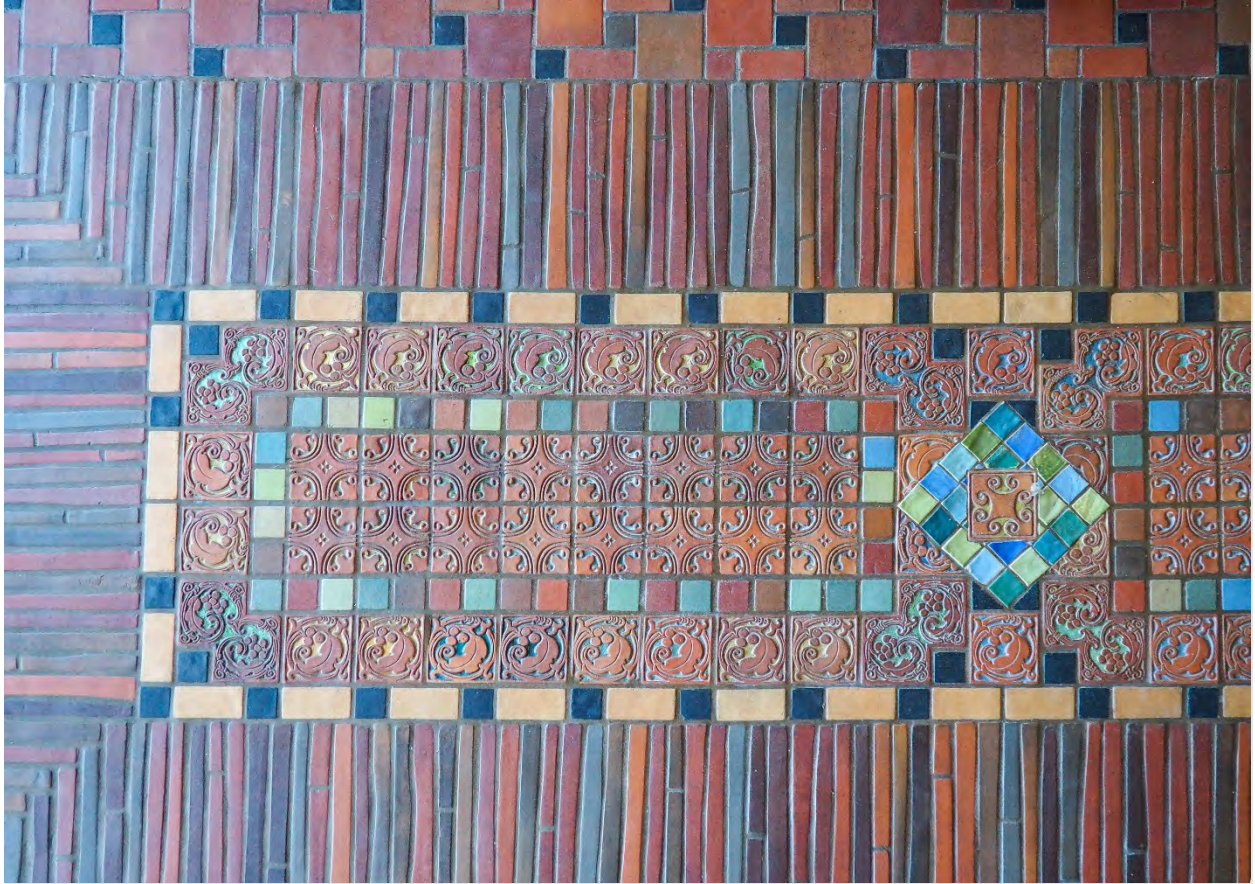
Photograph 36: Detail of the entrance hall Batchelder handmade tile floor, 2024. Source: McGuire Igleski & Associates, Inc.
