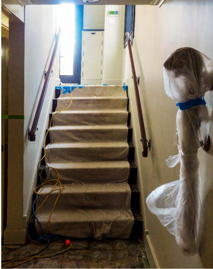
Photograph 11: View ascending the basement stair, 2024.
