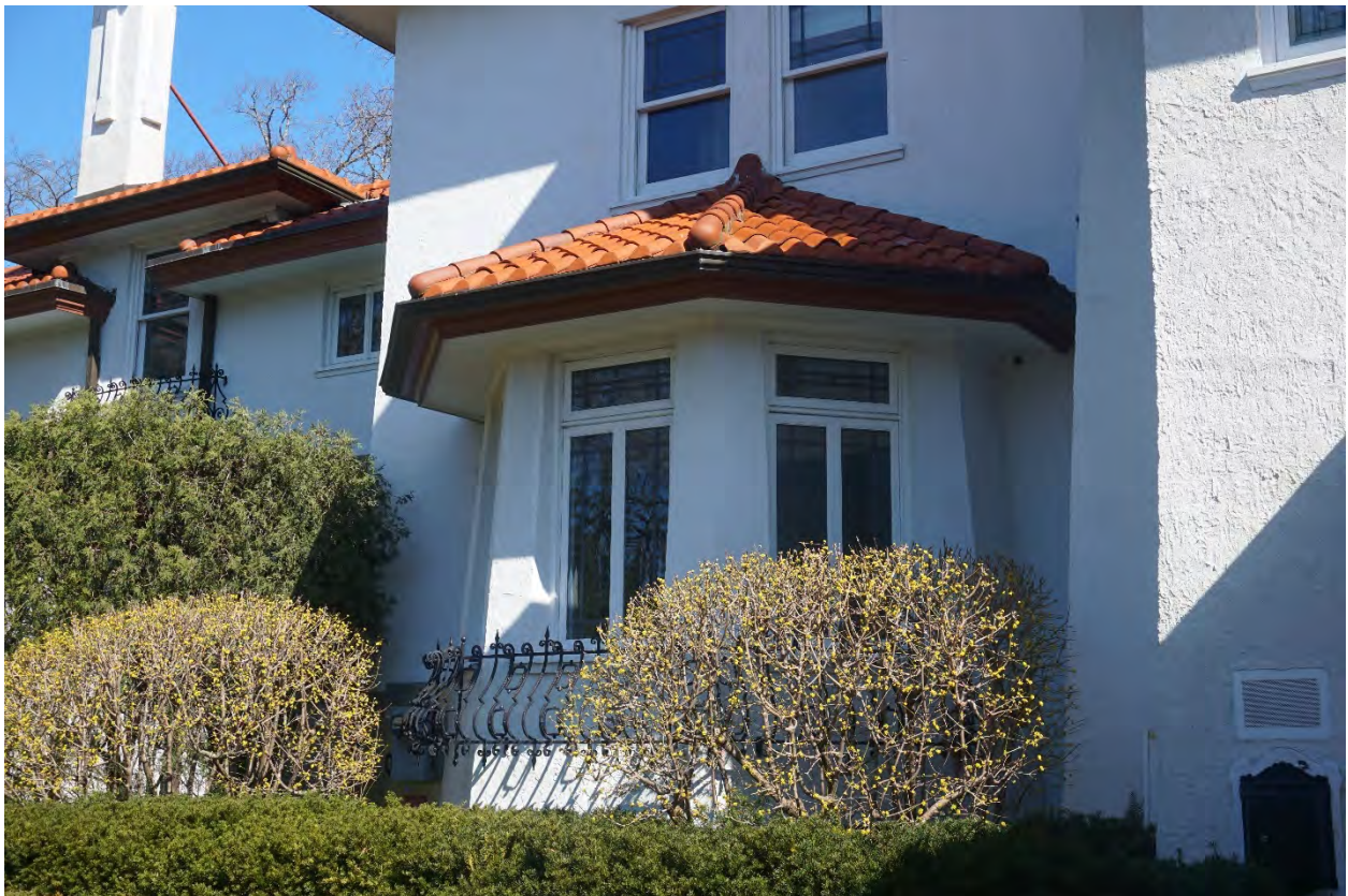
Photograph 4: Detail of the west façade first floor oriel window looking north, 2024.
