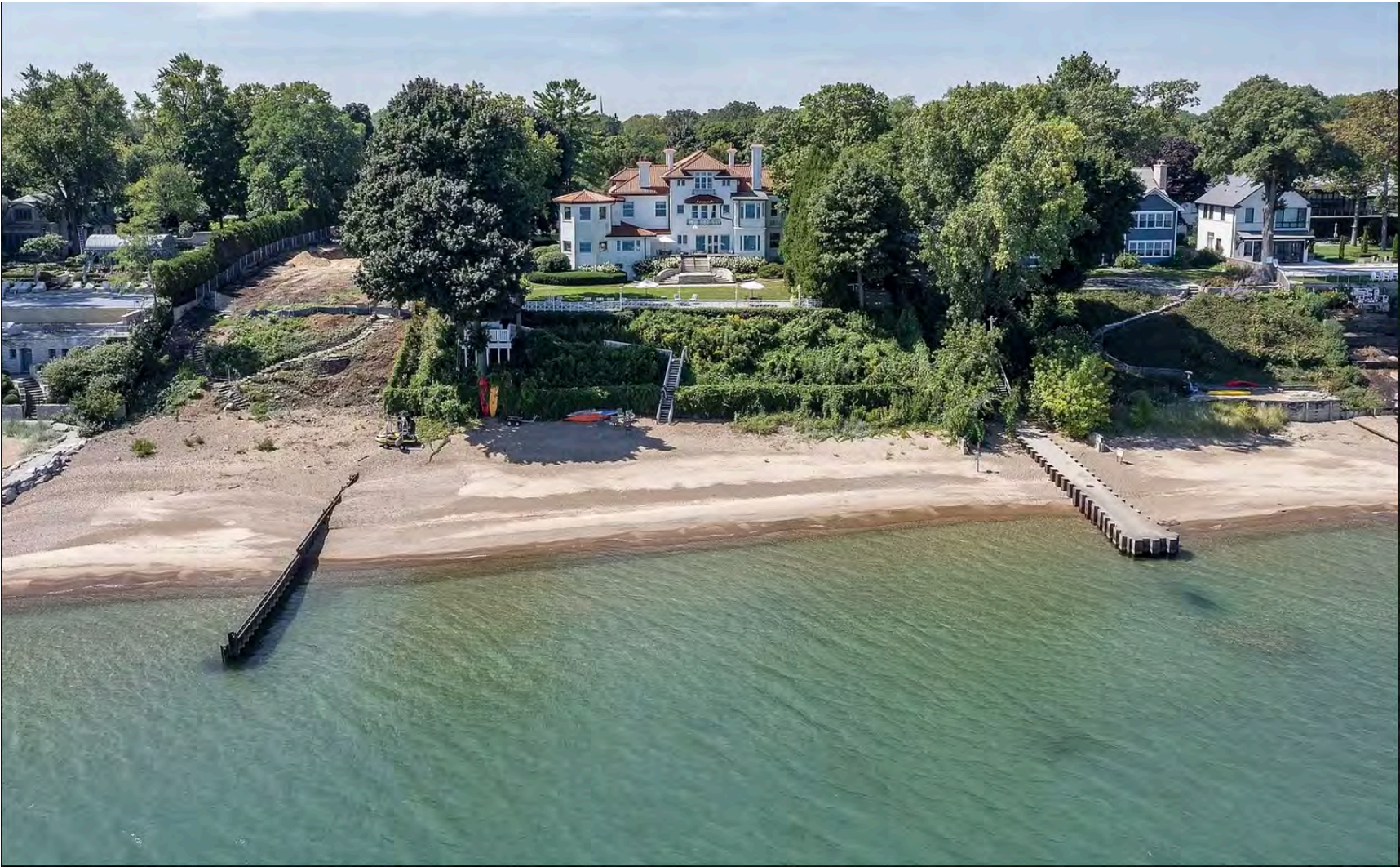
Photograph 6: View of the exterior, looking west; 2022.
