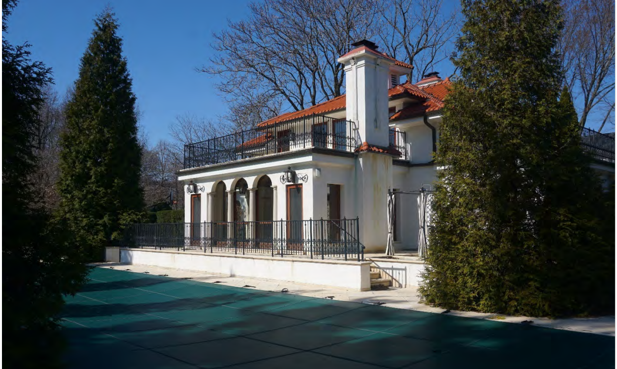
Photograph 83: View of the south elevation of the pool house and pool, 2024.
