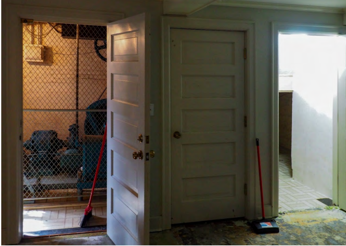
Photograph 13: View of the elevator control room and closets, 2024.
