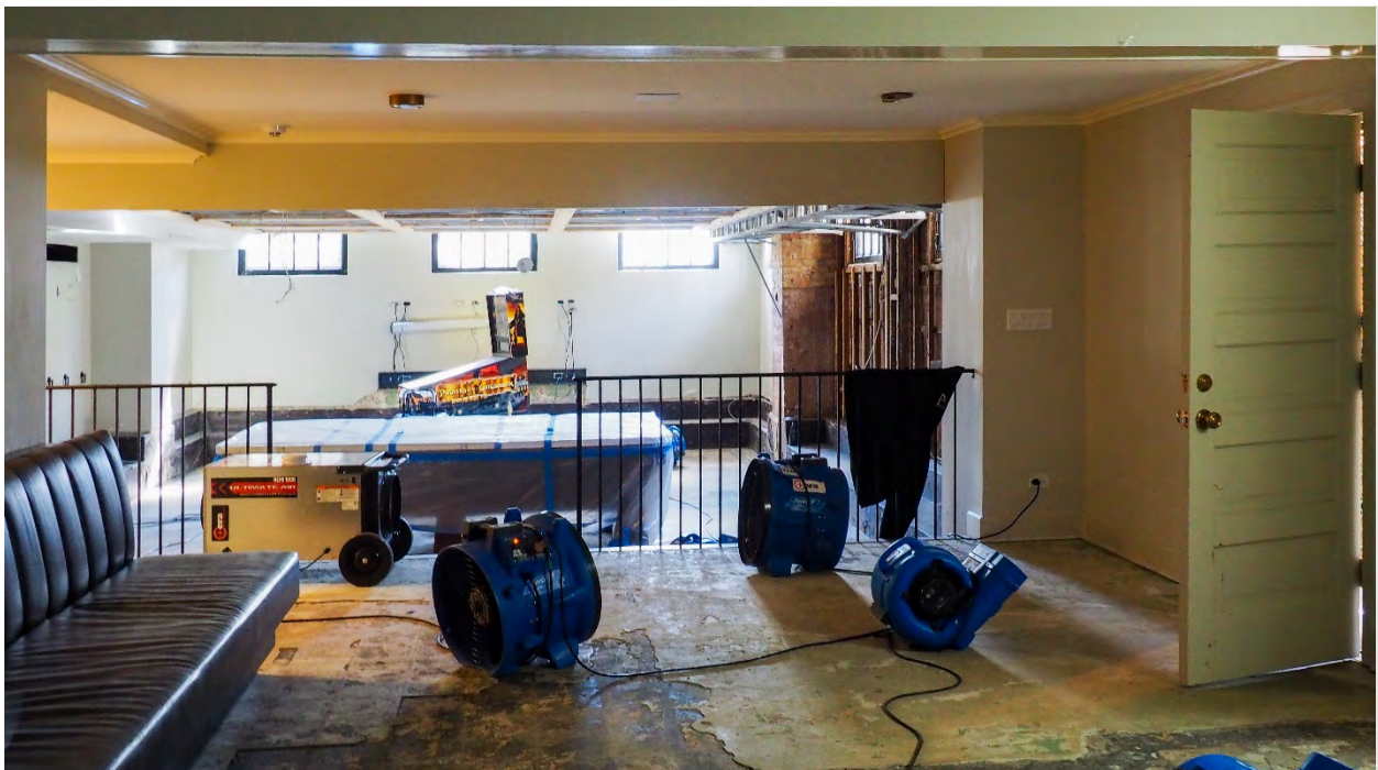
Photograph 12: View of the basement lounge and sunken recreation room looking south, 2024.
