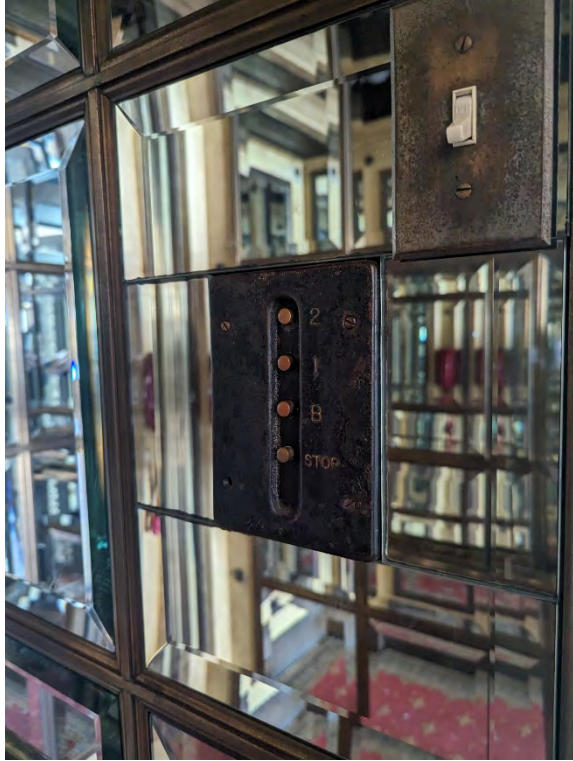
Photographs 77-78: Detail of the operatorless elevator switches, left, and the scissor door handle, right.
