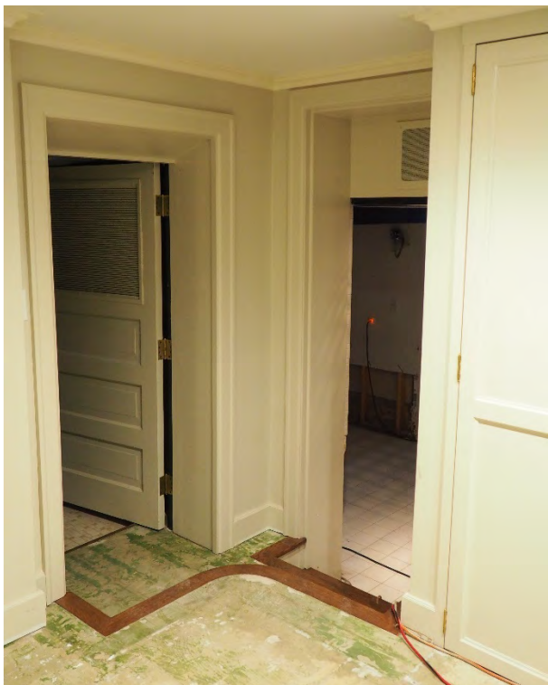
Photograph 26: View of the access to the basement storage areas, 2024.
