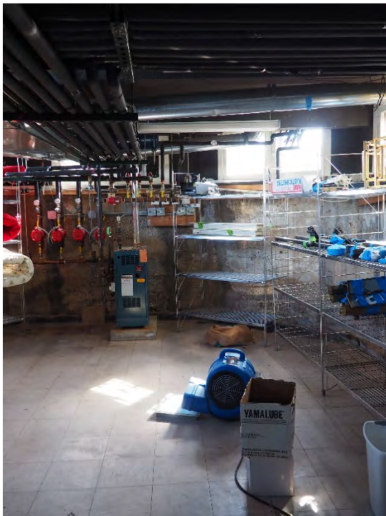
Photograph 28: View of the basement storage, 2024.
