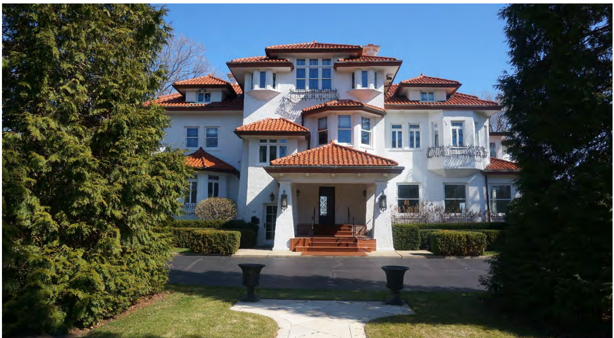
Photograph 2: View of the main/public entrance at the west façade looking northeast, 2024.
