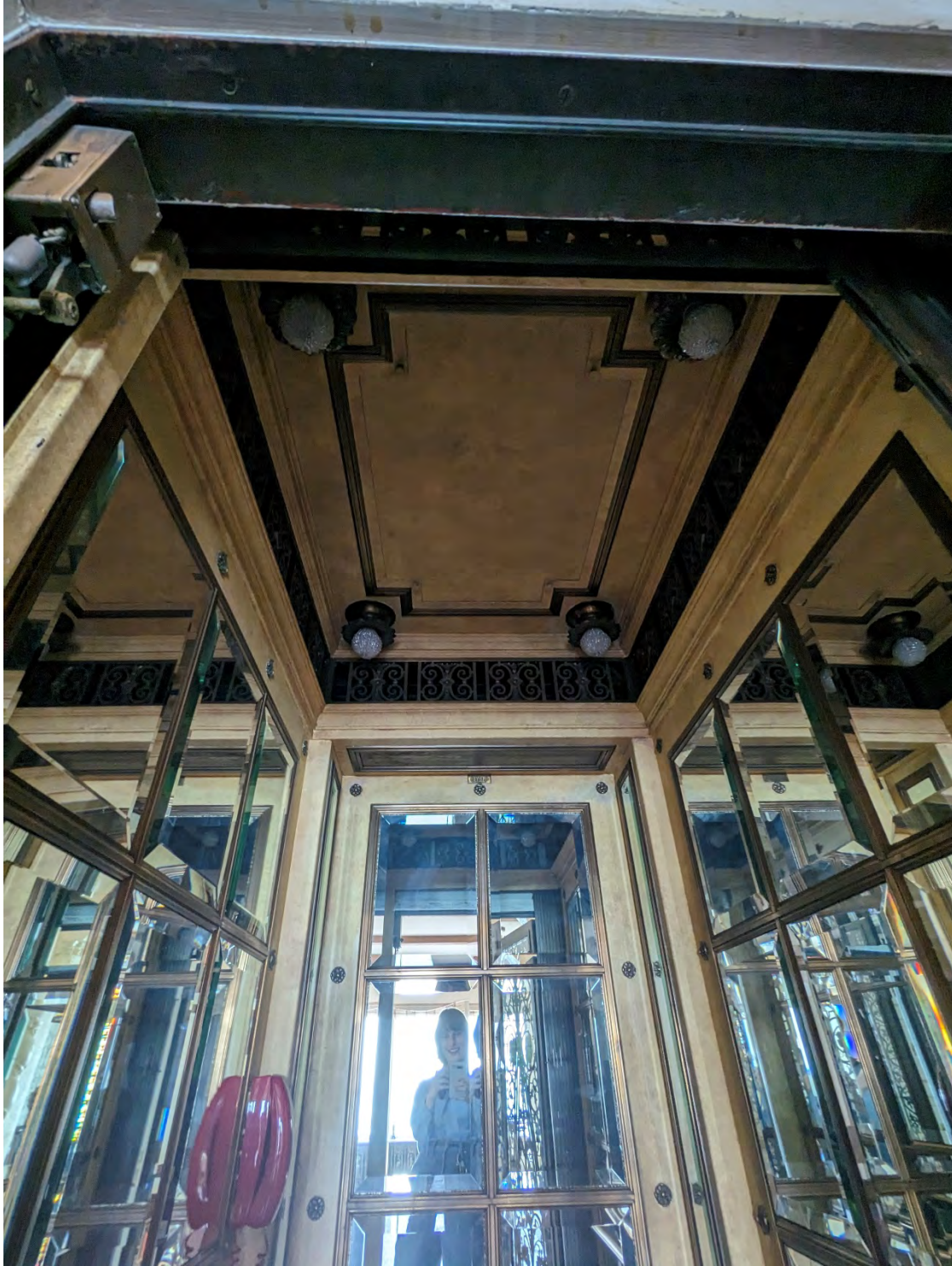
Photograph 75: Elevator Company of America Elevator interior and ceiling.
