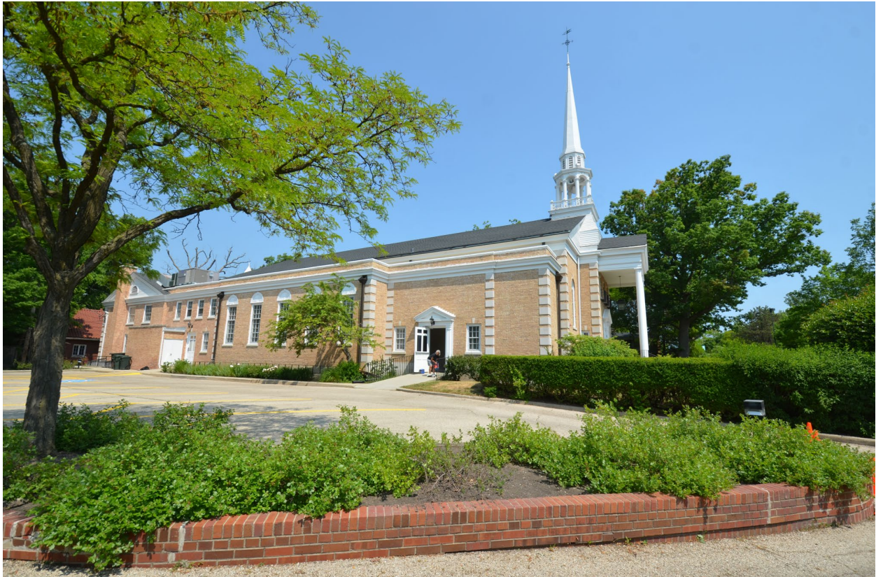
Figure 5 – Grace Presbyterian Church – South Façade
