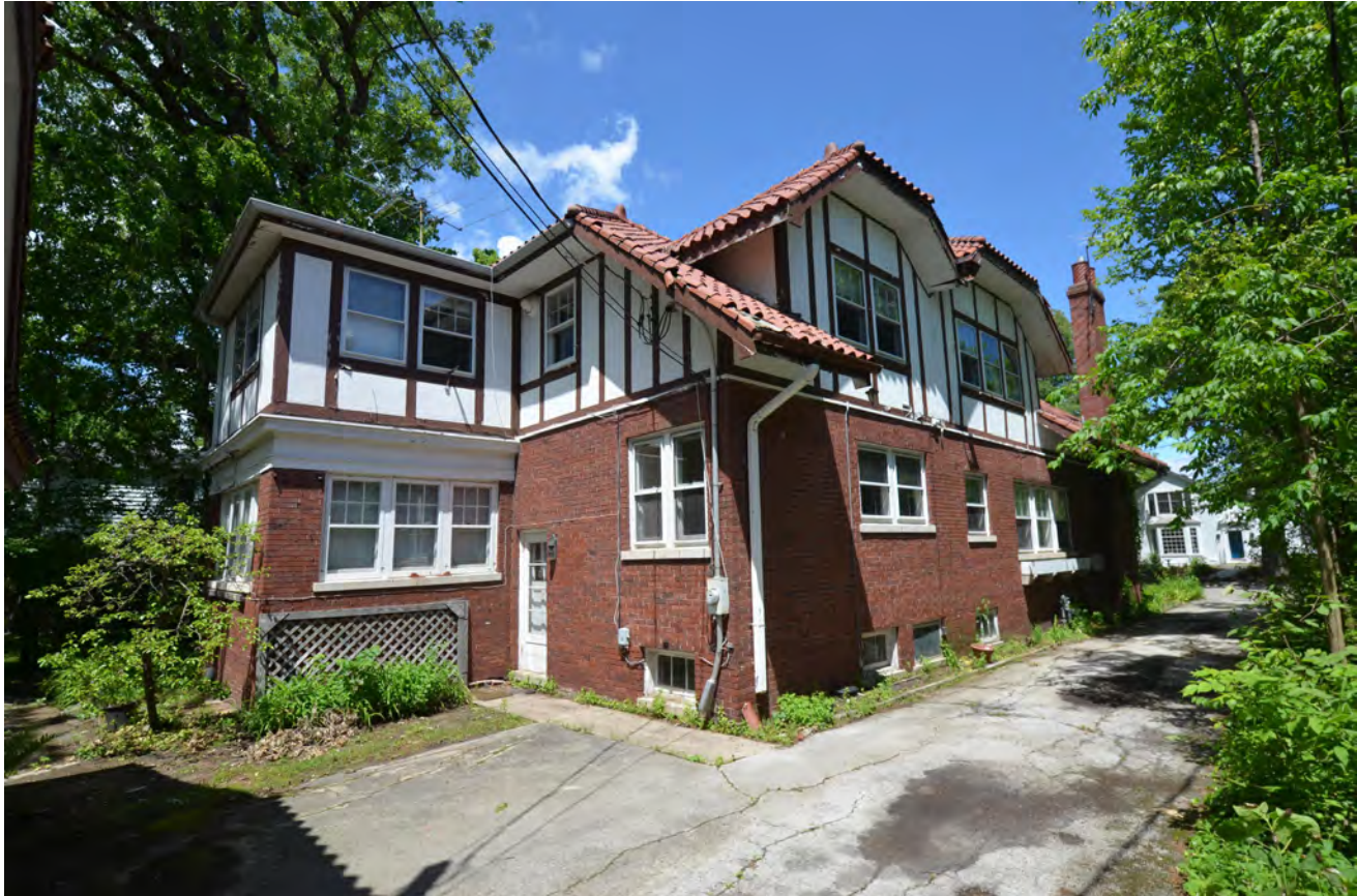
VIEW OF SOUTH & EAST FACADE
