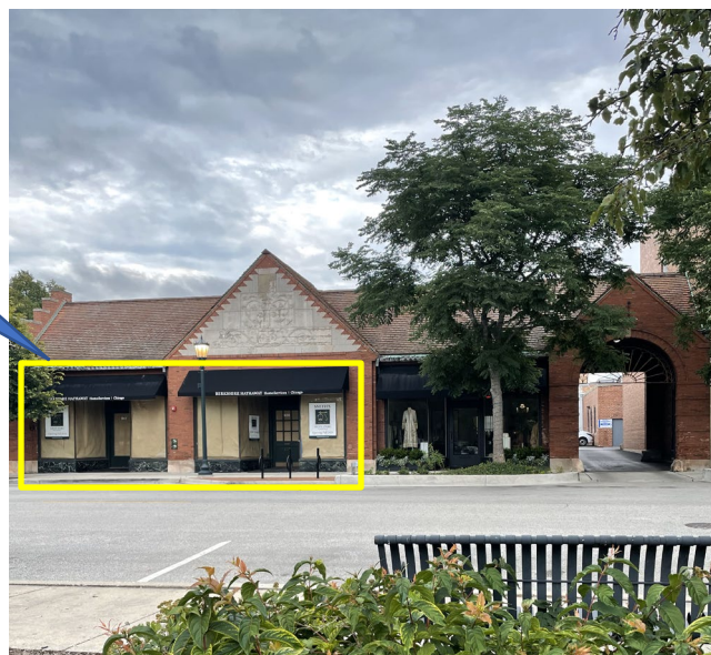
Figure 1 – Subject Property View of the Entire Building from Elm Street
