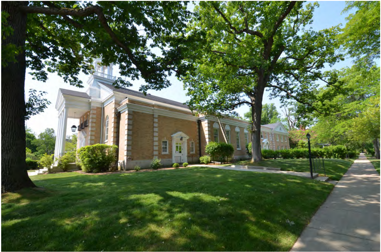
VIEW OF NORTH FACADE
