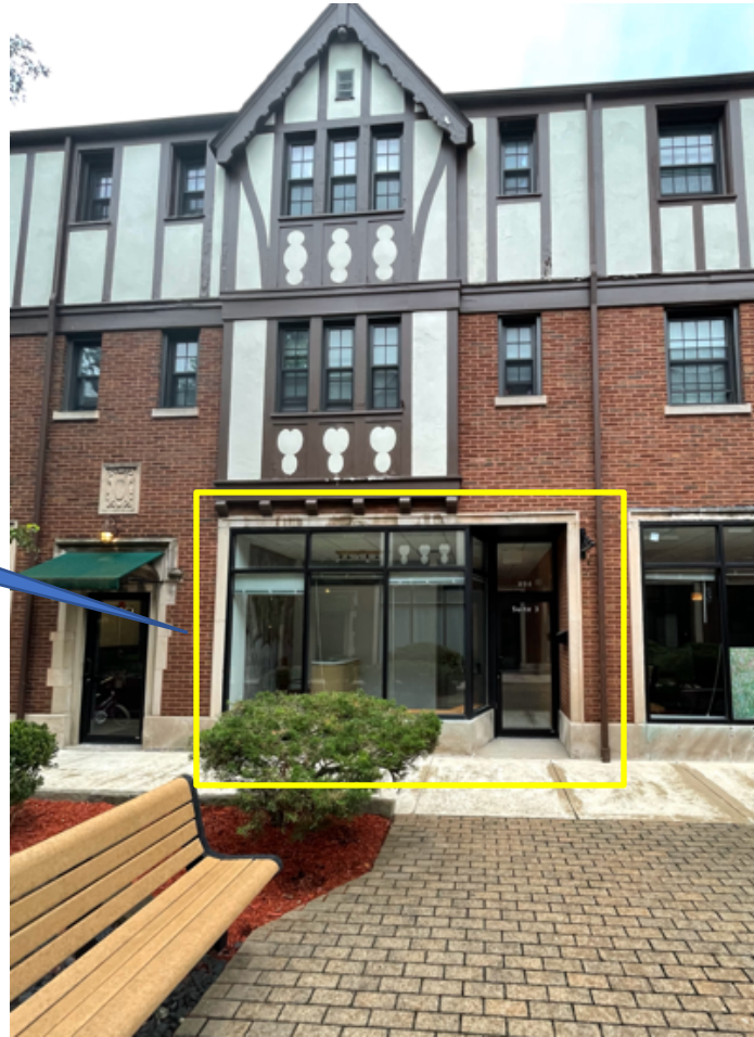
Figure 1 – Subject Property – Storefront of Pelvio LLC in building courtyard
