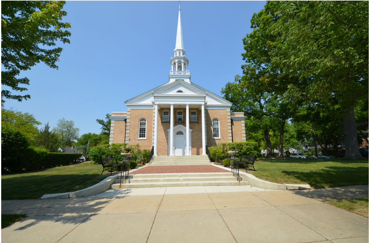
Figure 3 – Grace Presbyterian Church – East Façade
