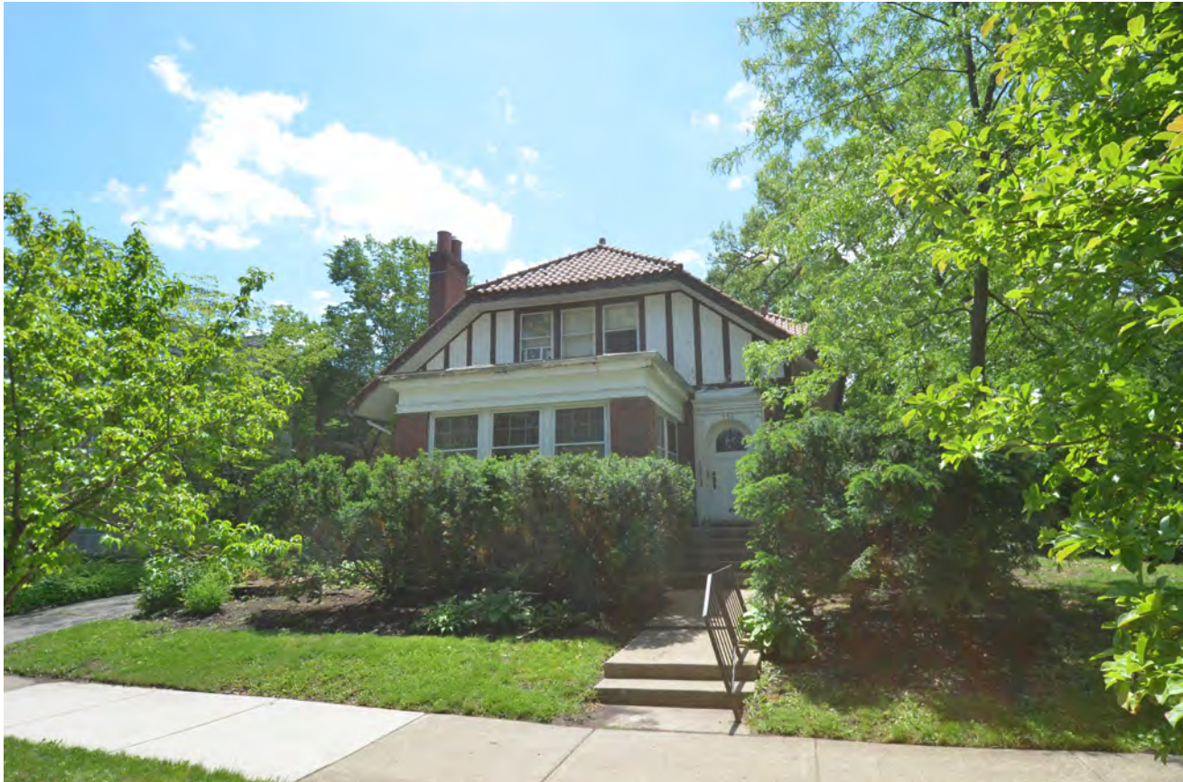
VIEW OF NORTH FACADE
