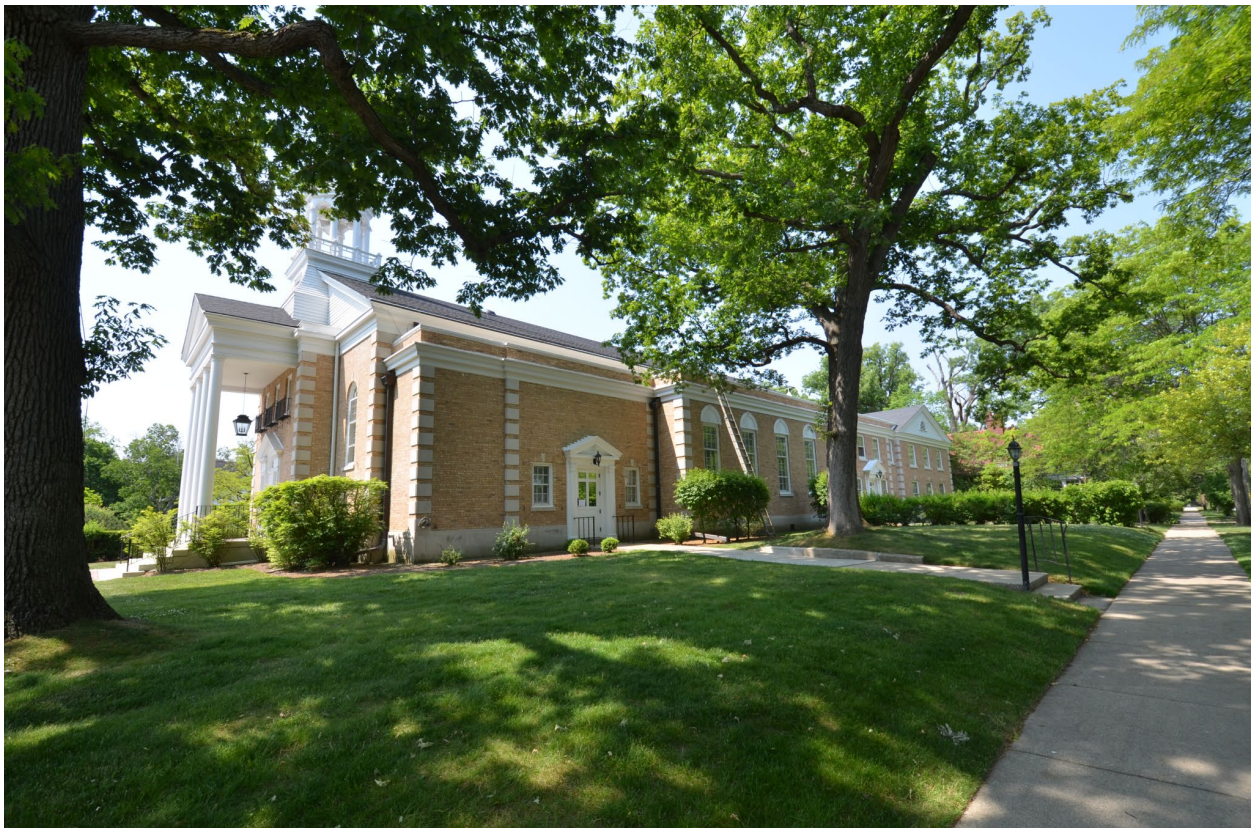
Figure 4 – Grace Presbyterian Church – North Façade
