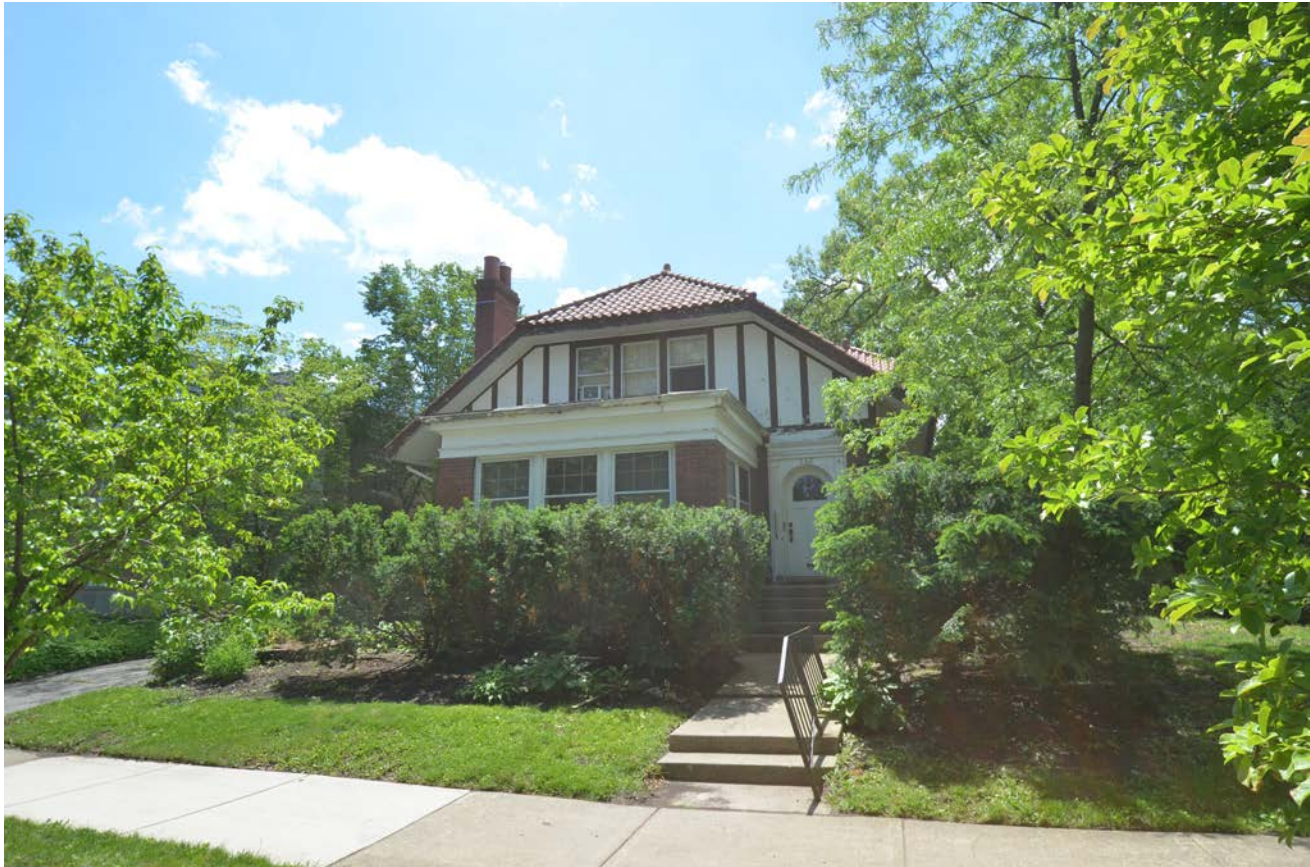
VIEW OF NORTH FACADE
