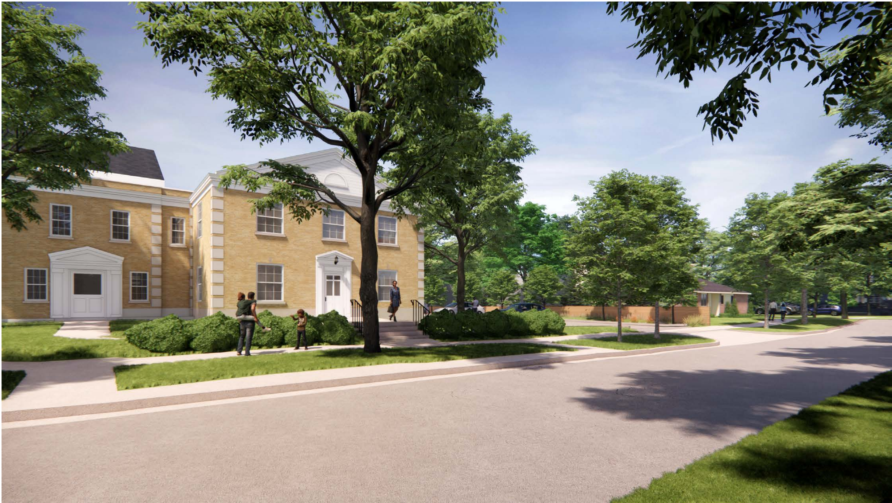
VIEW OF NORTH ADDITION FROM CHERRY STREET
