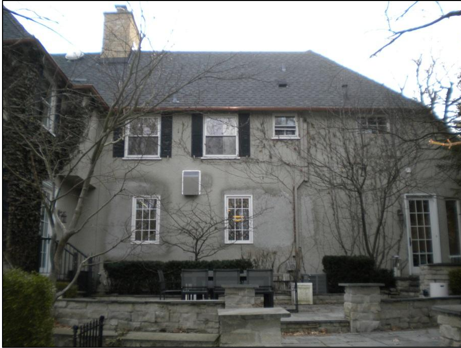
North half of rear façade, Spring 2019, looking W, Spring 2019
