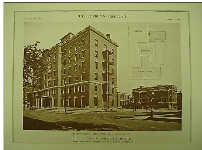
Chicago Lying In Hospital, 432 E. 51 st Street
