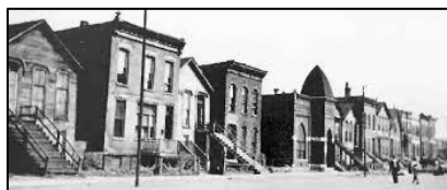
Deteriorated Housing in Chicago
