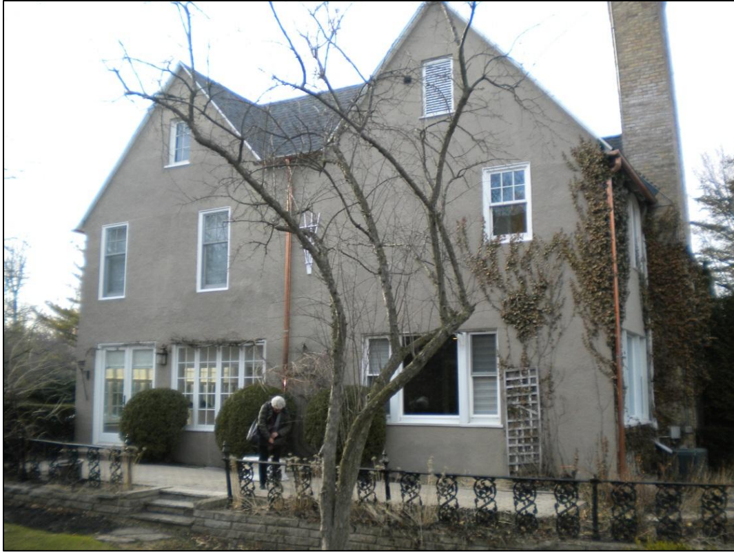
South (side) façade of main house, looking N, Spring 2019
