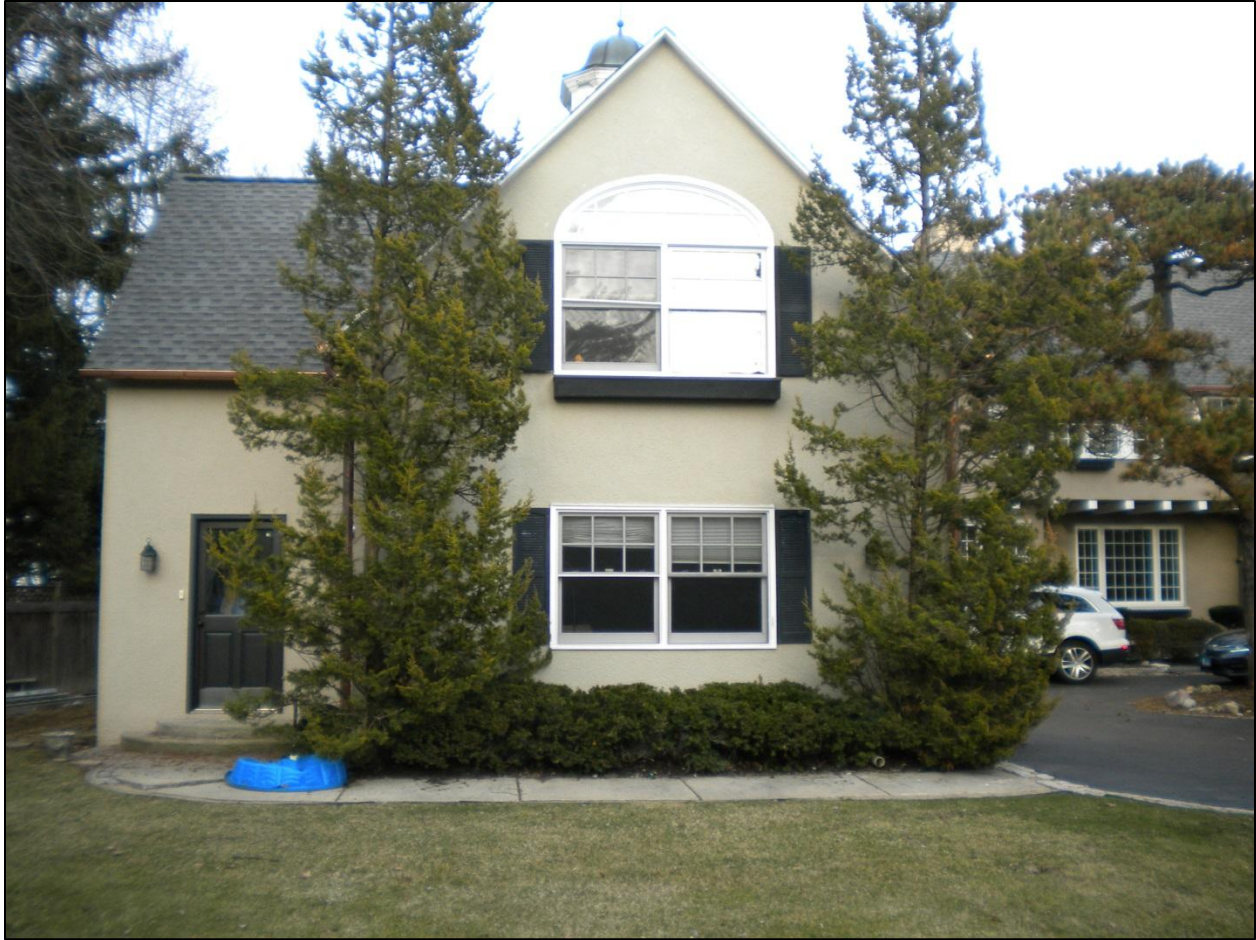
West façade of garage wing addition, looking E, Spring 2019
