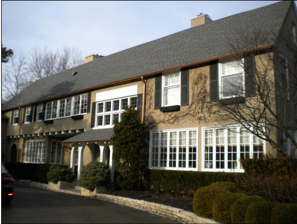
Main house, front façade, looking NE, Spring 2019
