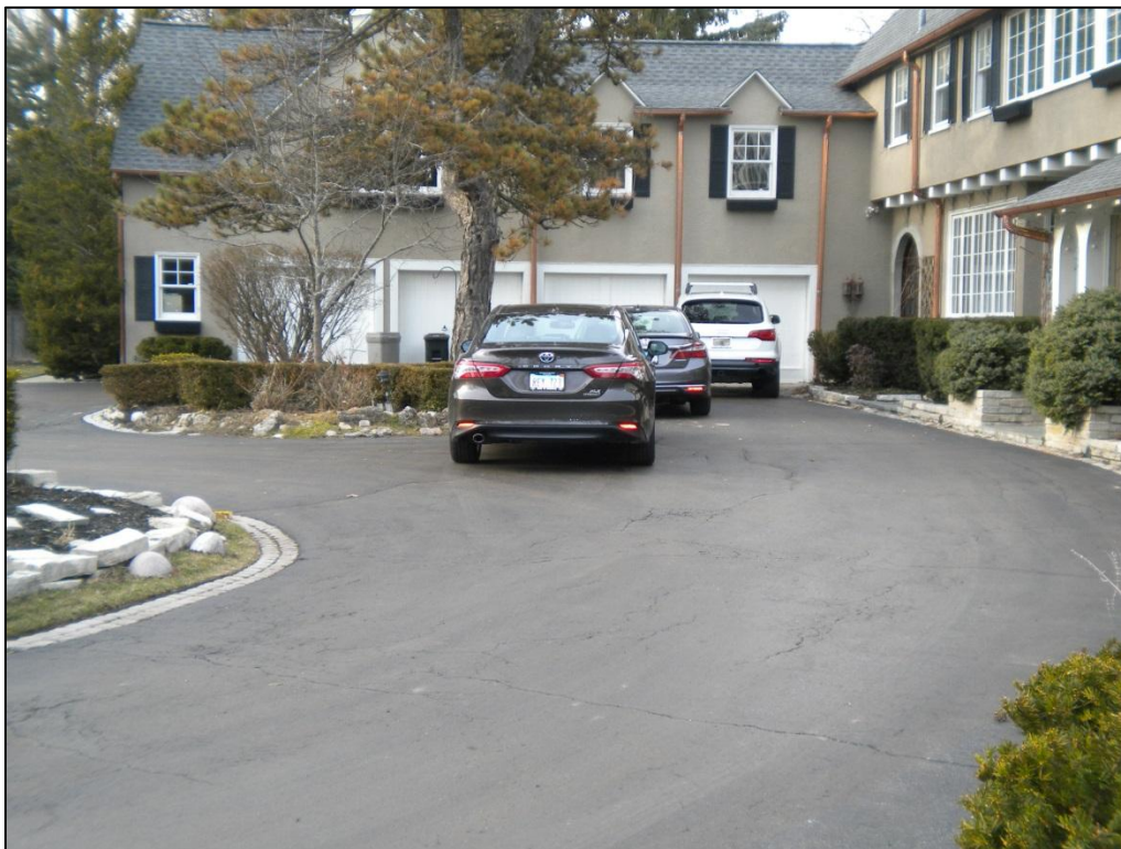
Garage wing, looking N, Spring 2019.
