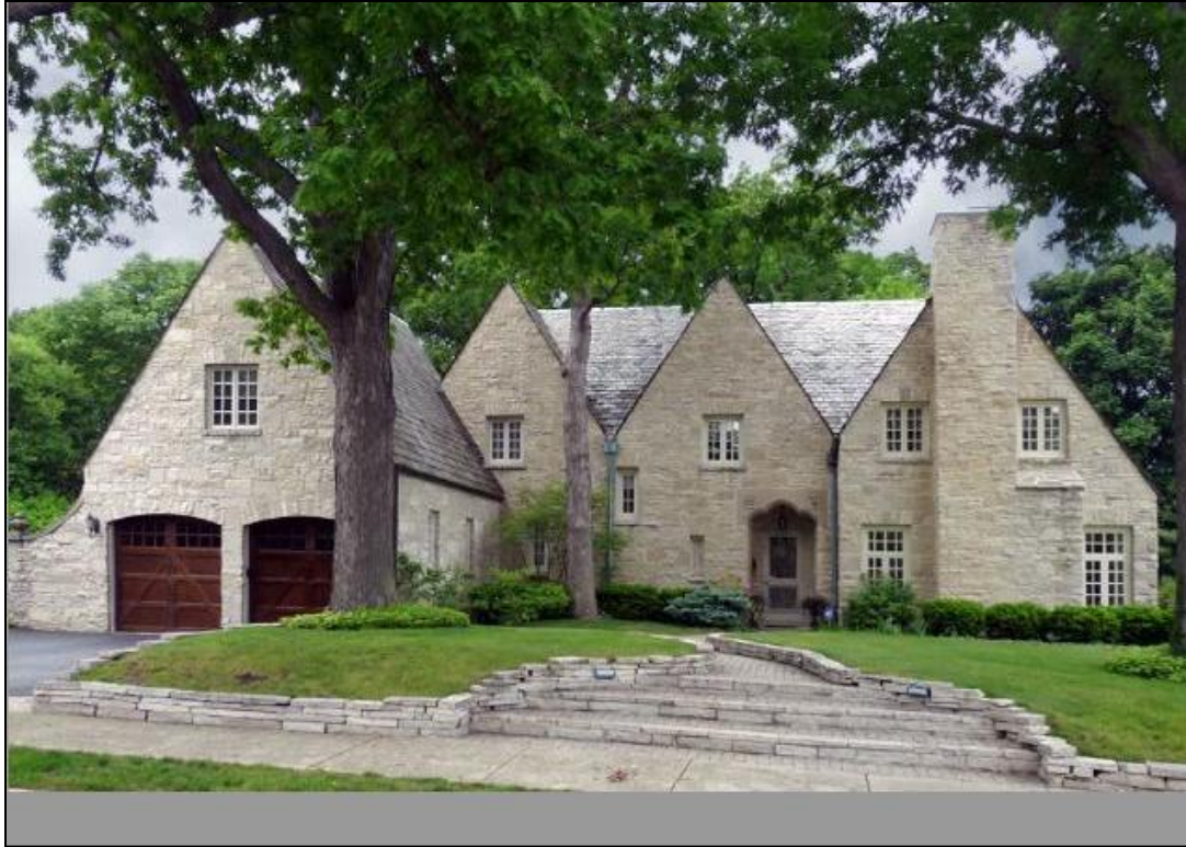
Mayfield House, ca. 1926, 145 Montgomery, Glencoe
