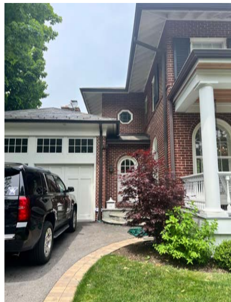
Main (south) façade, side entrance
