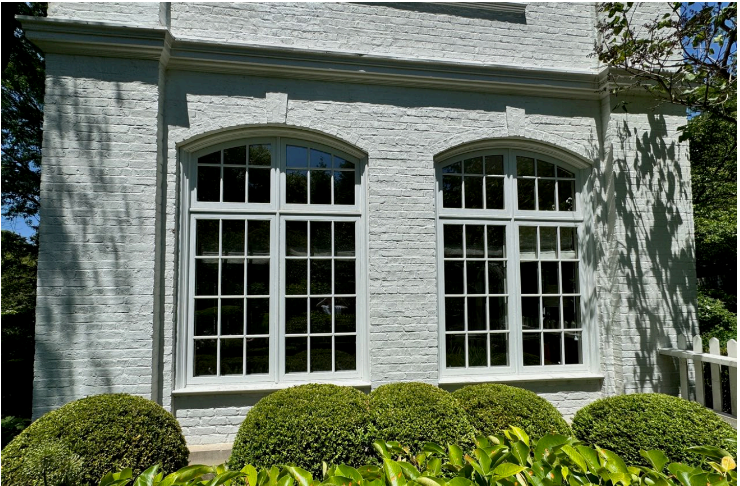
South Building Façade – Windows Proposed For Replacement
