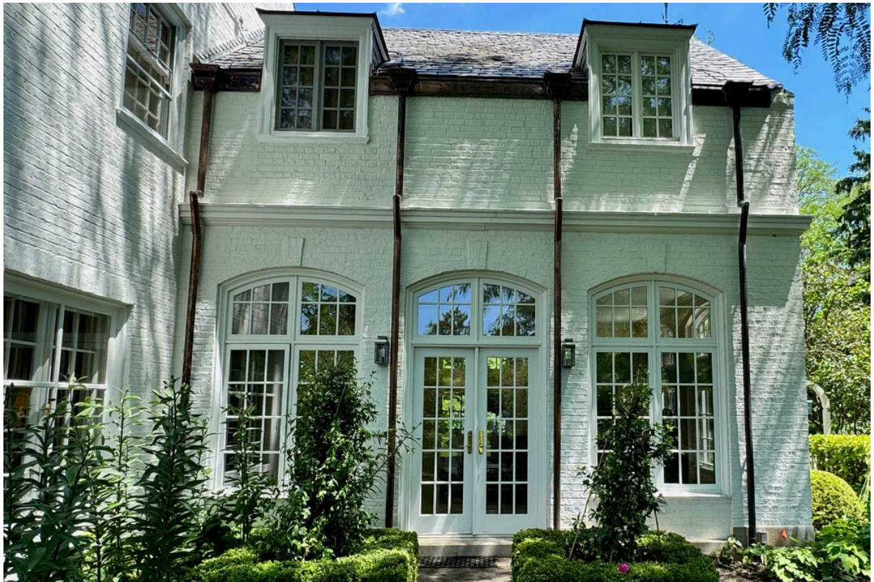
West Building Façade – Windows and Doors Proposed For Replacement
