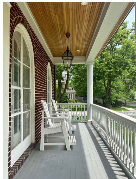
Front porch looking east
