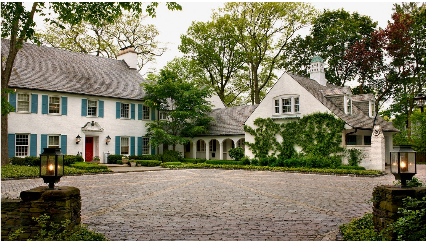
Front Building Face – July 2024
