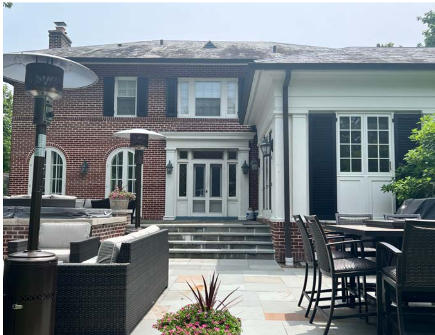
North (Rear) Facade
