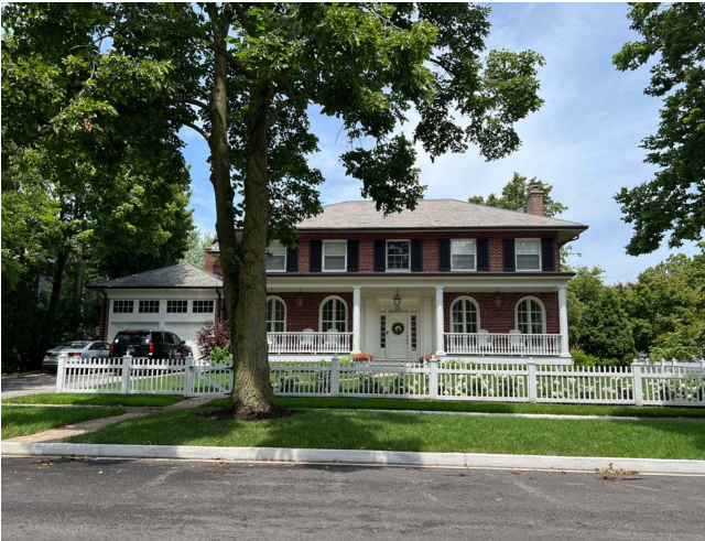
Main (south) façade
