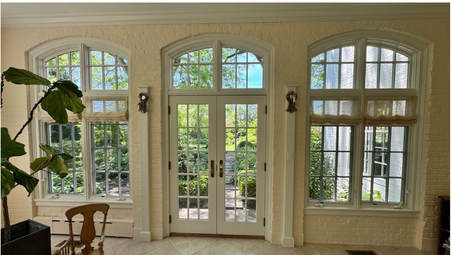
West Building Face – Interior View of Windows Proposed for Replacement
