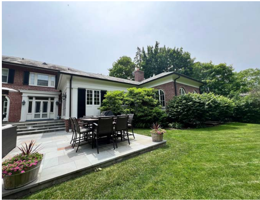
North (Rear) Facade
