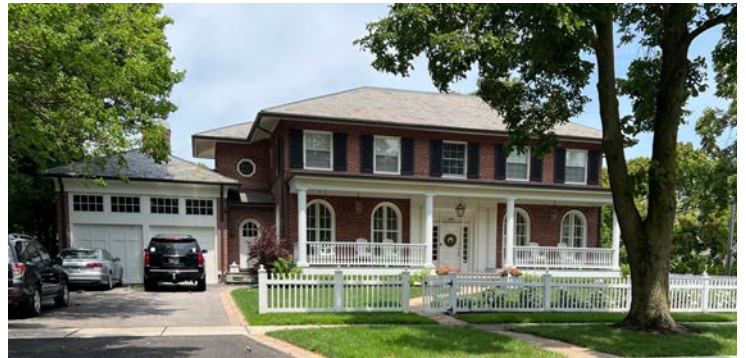
Main (south) façade
