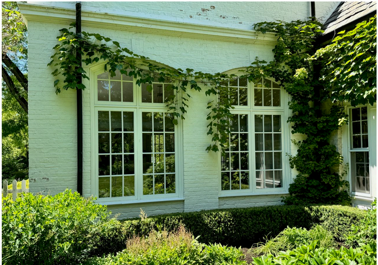
East Building Façade – Windows Proposed For Replacement
