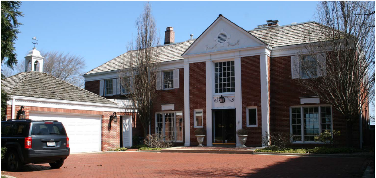
Figure 4 – Subject Property - Front Elevation (West)
