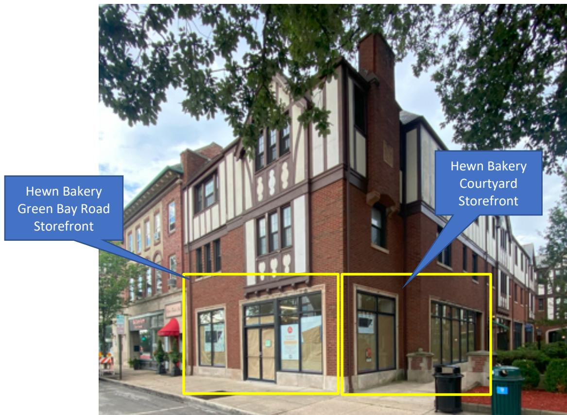
Figure 2 – Subject Property – Storefront of Hewn Bakery/View from Green Bay Road
