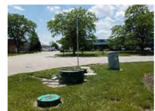
Thomas Foster Lift Station will be converted from a 'can-type' to a submersible station.
