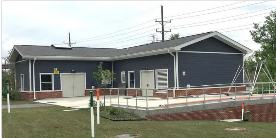
The FRWRD's pumping station 31.
