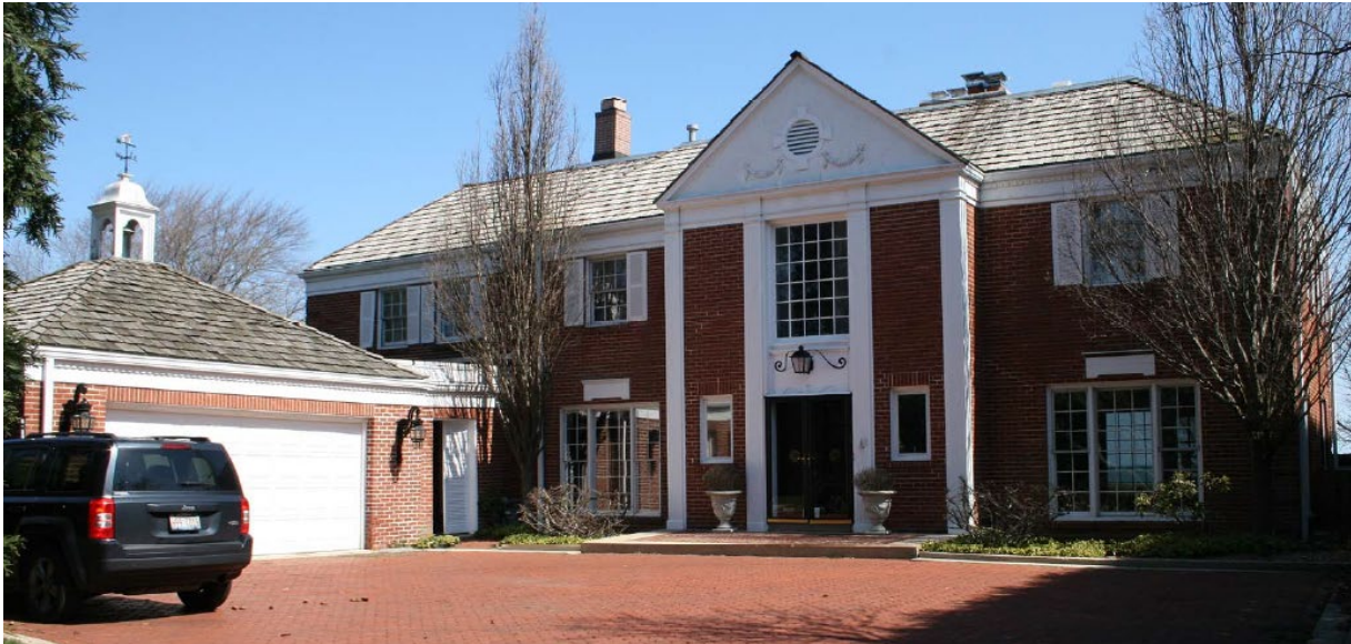
Figure 4 – Subject Property - Front Elevation (West)
