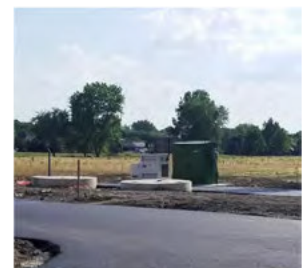
141st Street pumping station constructed in 2020.
