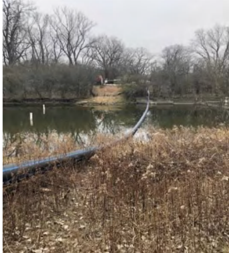
16-inch-diameter HDPE water main fused together to be installed via HDD through the FPDCC Skokie Lagoon. Multiple lagoon crossings were required, and extensive laydown area was needed to fuse together 2,650 feet of pipe.
