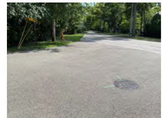
The Village may want to consider modification to the dual gravity sewers on Old Green Bay Road with this project.
