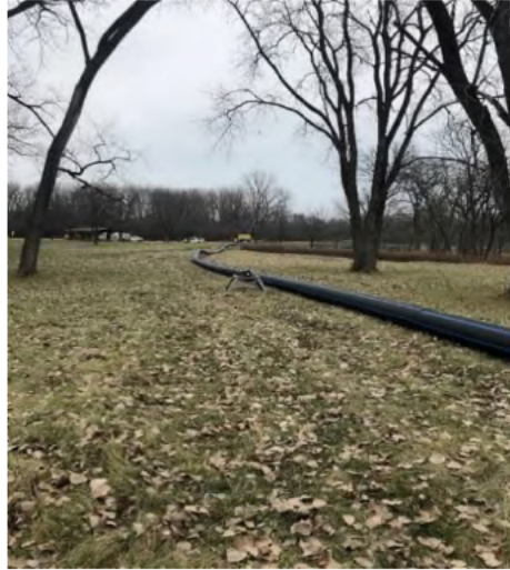
16-inch-diameter HDPE water main fused together to be installed via HDD through the FPDCC Skokie Lagoon. Multiple lagoon crossings were required, and extensive laydown area was needed to fuse together 2,650 feet of pipe.
