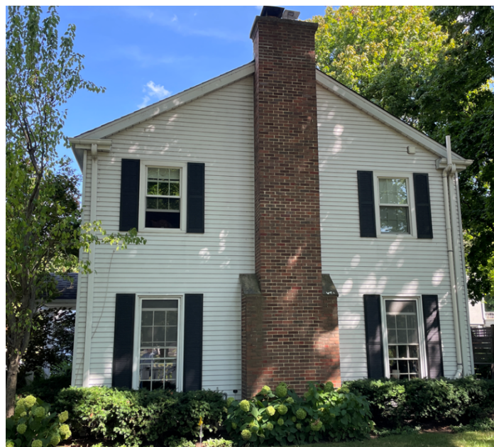
Figure 5 – Subject Property - South Elevation (Elm Street)
