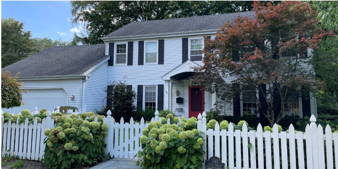
Figure 3 – Subject Property – Corner Elevation (Maple Street)
