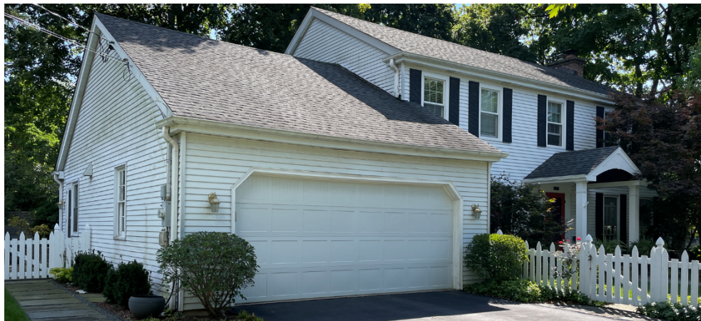
Figure 4 – Subject Property – Corner and North Elevation (Maple Street)
