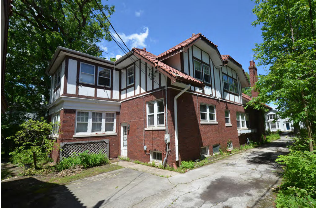
VIEW OF SOUTH & EAST FACADE
