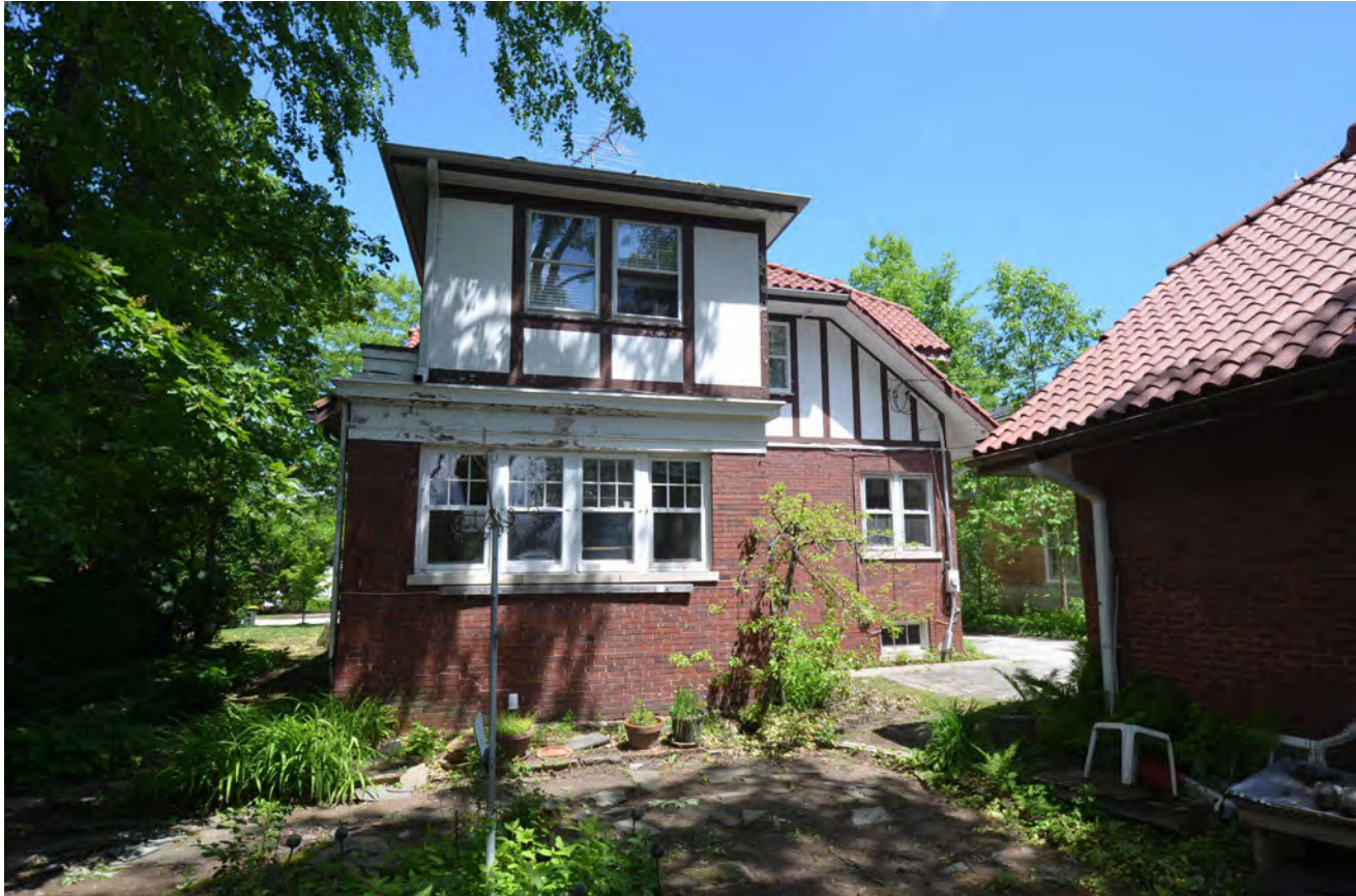
VIEW OF SOUTH FACADE
