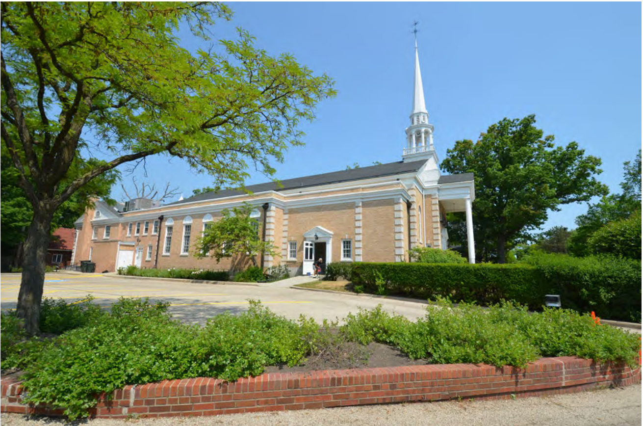
VIEW OF SOUTH FACADE
