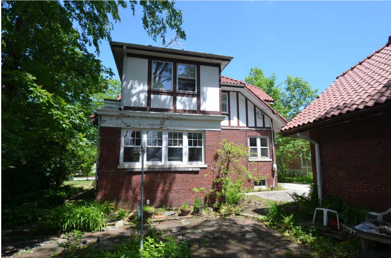
VIEW OF SOUTH FACADE
