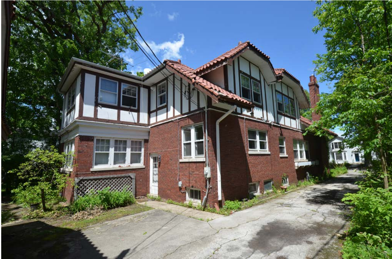
VIEW OF SOUTH & EAST FACADE
