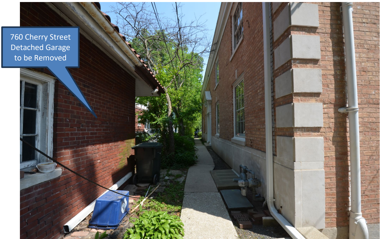
Figure 6 – Grace Presbyterian Church – West Façade
