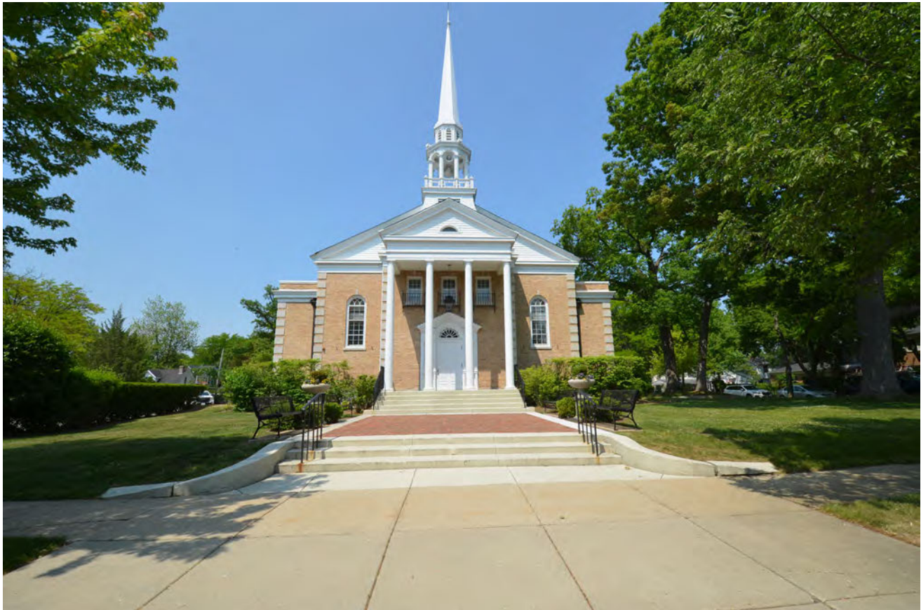
VIEW OF EAST FACADE
