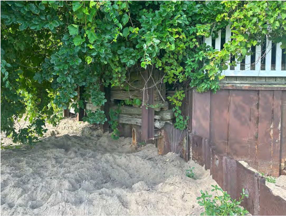
North Seawall (Looking West)
