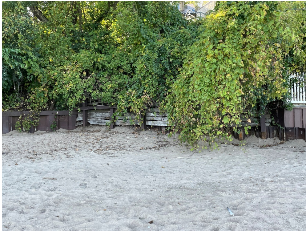
Figure 15 - Existing Wooden Timbers, Steel I-Beams, and Steel Sheet Piling to be Replaced
