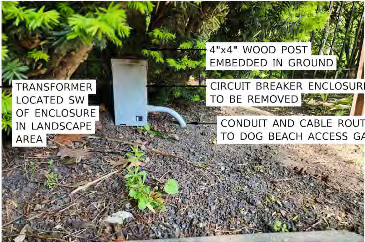
EXISTING ELECTRIC SERVICE (FOR REFERENCE ONLY) N.T.S.
