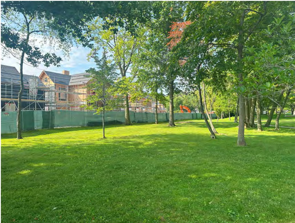
Upper Park (Looking South)
