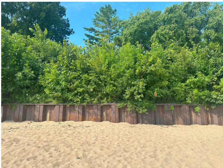
Figure 11-Existing Sea Wall on Subject Property
