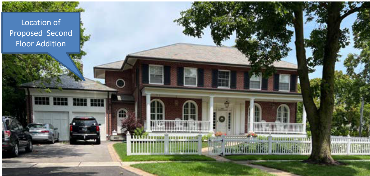
Figure 3 – Subject Property - Front Elevation (Elm Street)
