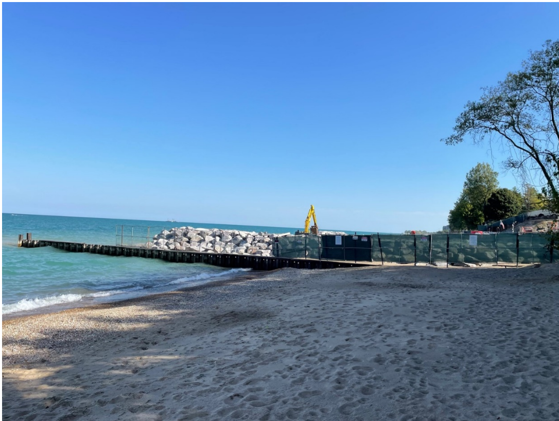
Figure 8 – Subject Property – Looking South at Existing Steel Groin on Centennial Beach & Stone Groin at 205 Sheridan Road Property
