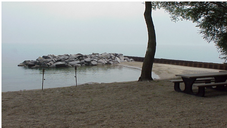
Figure 9 - Steel and stone groin
