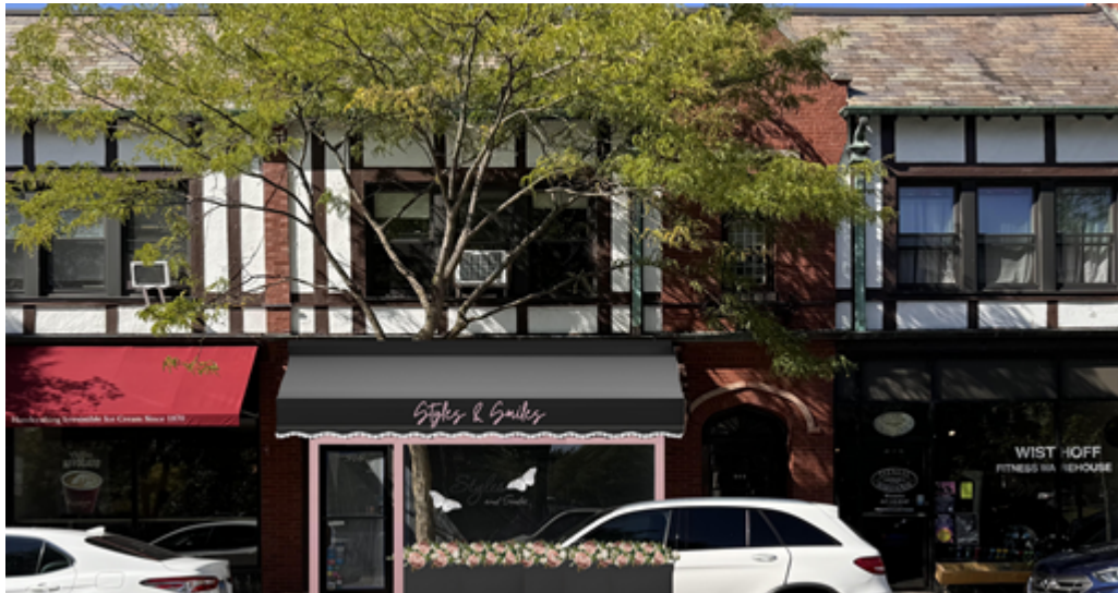
Subject Property – Proposed awning fabric and door and window trim paint changes to the storefront
