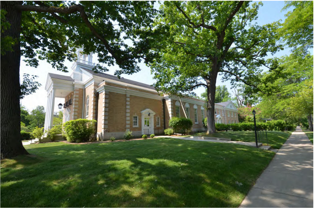
VIEW OF NORTH FACADE
