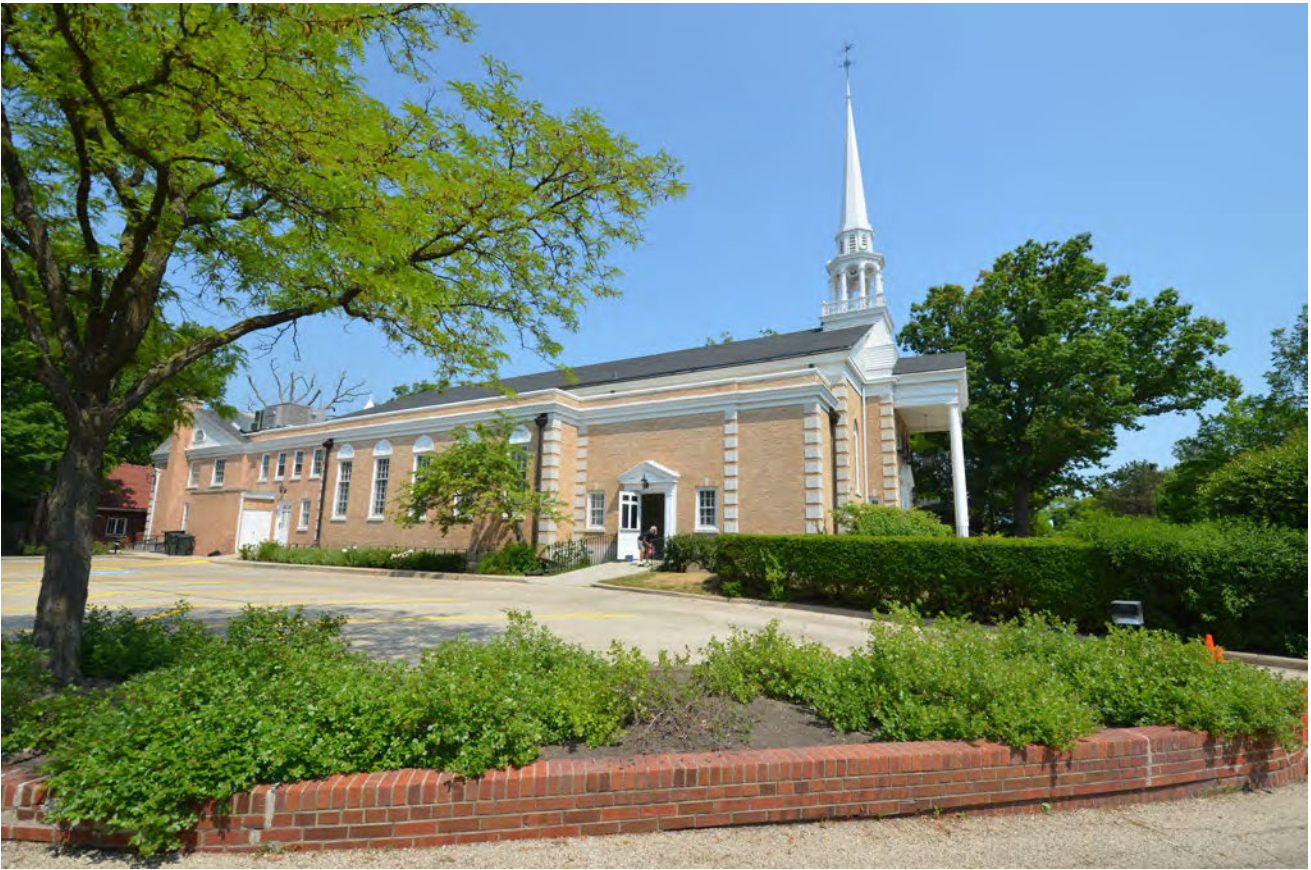
VIEW OF SOUTH FACADE
