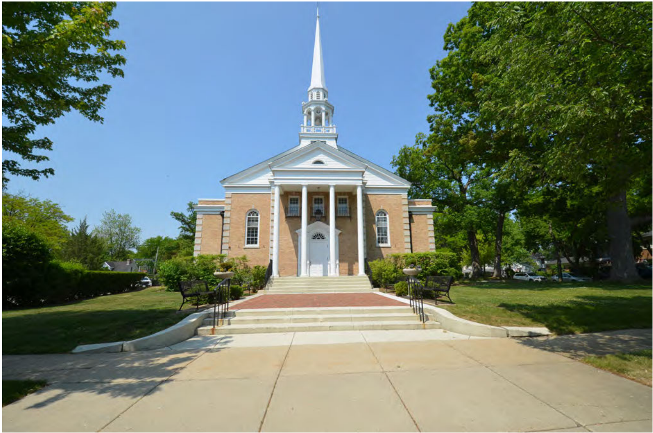
VIEW OF EAST FACADE
