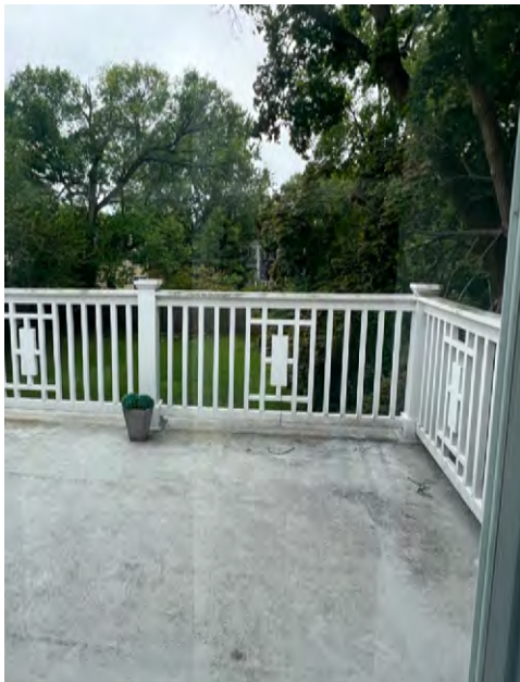
Deck over sunporch view south
