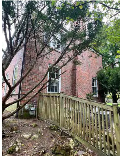
West façade view southeast
