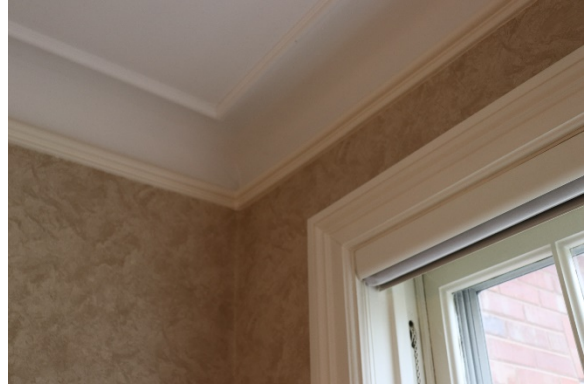
Detail of window and historic casings and cove trim
