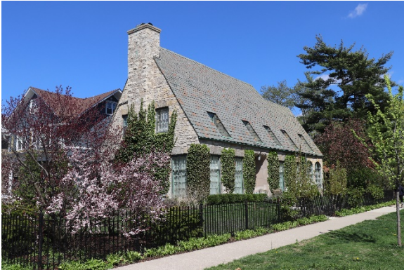
700 Fair Oaks, Oak Park – A 1926 Norman Cottage Style home with stone walls and a slate roof with inset dormers
