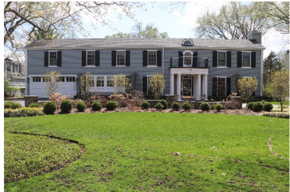
1180 Broadmeadow – A 1950 Colonial Revival Style with clapboard siding
