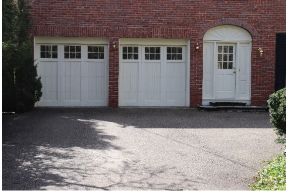
Garage doors and secondary entry
