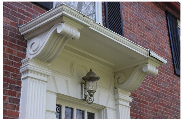
Detail of entry portico
