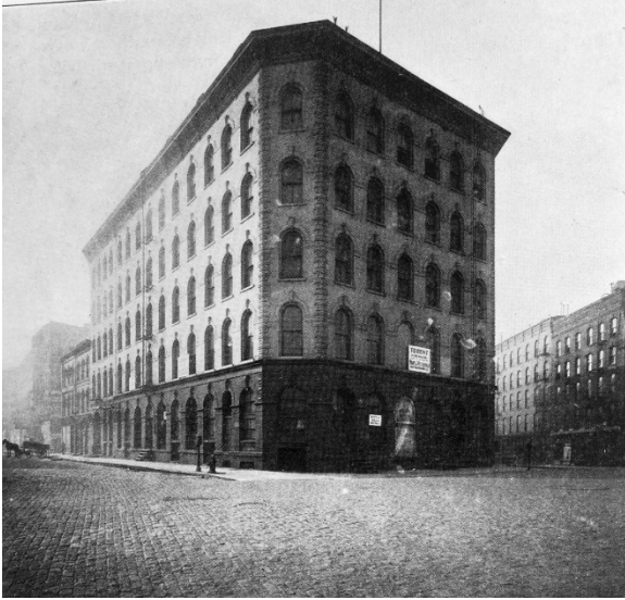
William M Hoyt Company Building at Michigan Avenue and River Street (demolished – now the London Guarantee Building at Wacker Drive)
