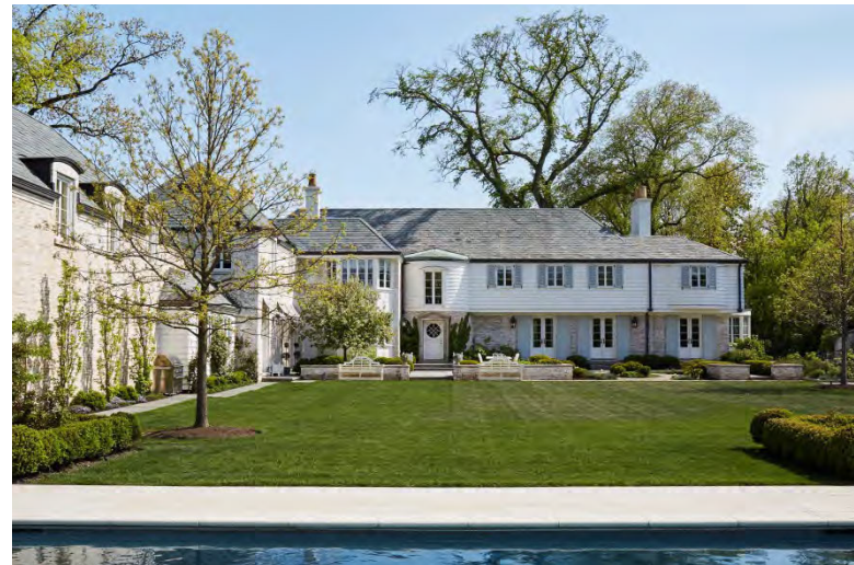
North (rear) elevation post-renovation.
