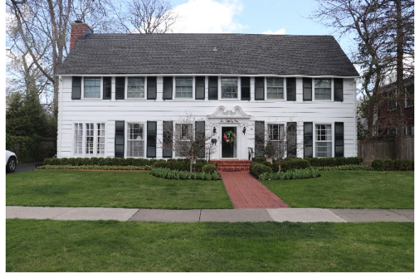
681 Garland – A 1927 Colonial Revival Style with clapboard and excellent integrity
