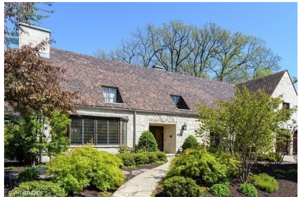
2424 Lincoln, Evanston – A 1930 Norman Cottage house with stone and a tile roof with inset dormers
