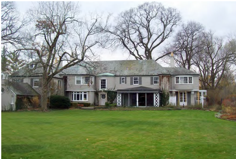
North (rear) elevation pre-renovation.
