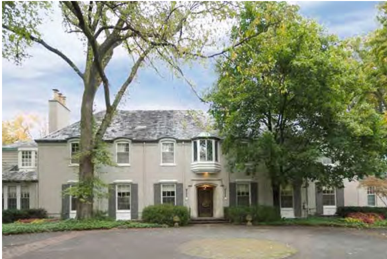
South (front) elevation pre-renovation.
