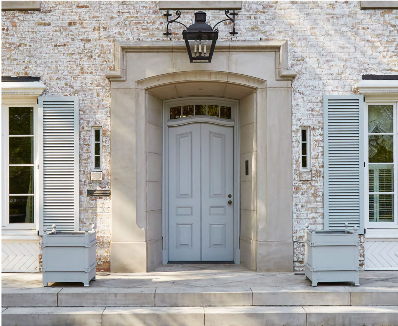
Replicated limestone surround to match original. New door and transom.
