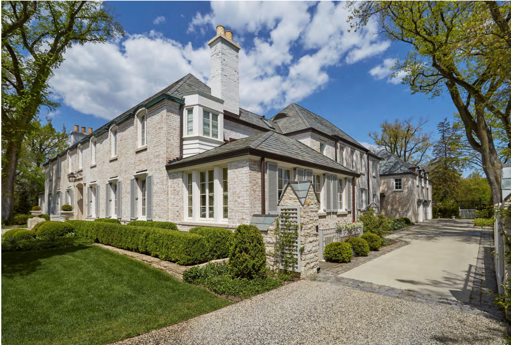
South and east elevations with gate posts reconstructed from salvaged material to original design..
