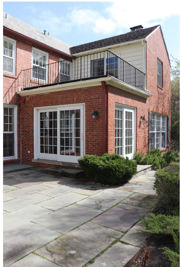
1979 addition at east end of the south elevation
