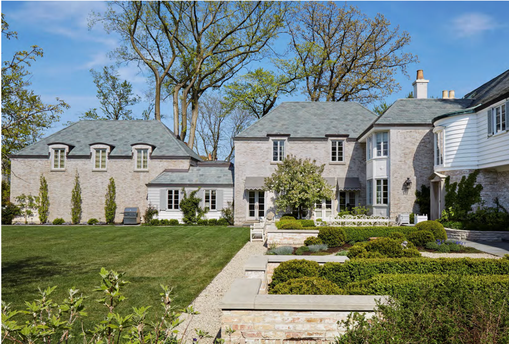
New wing with existing house at right.
