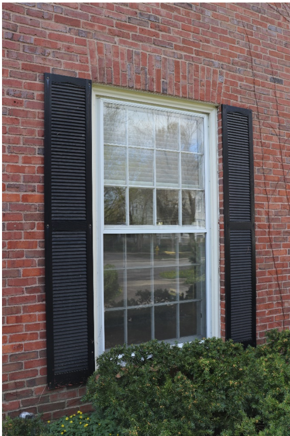
Ground floor multi-light windows and non-historic shutters
