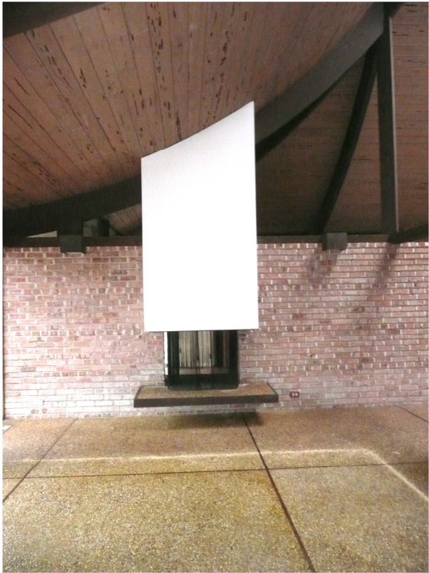
Living room fireplace, looking east
