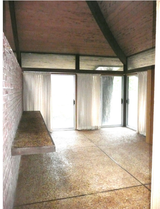
Dining room, looking east
