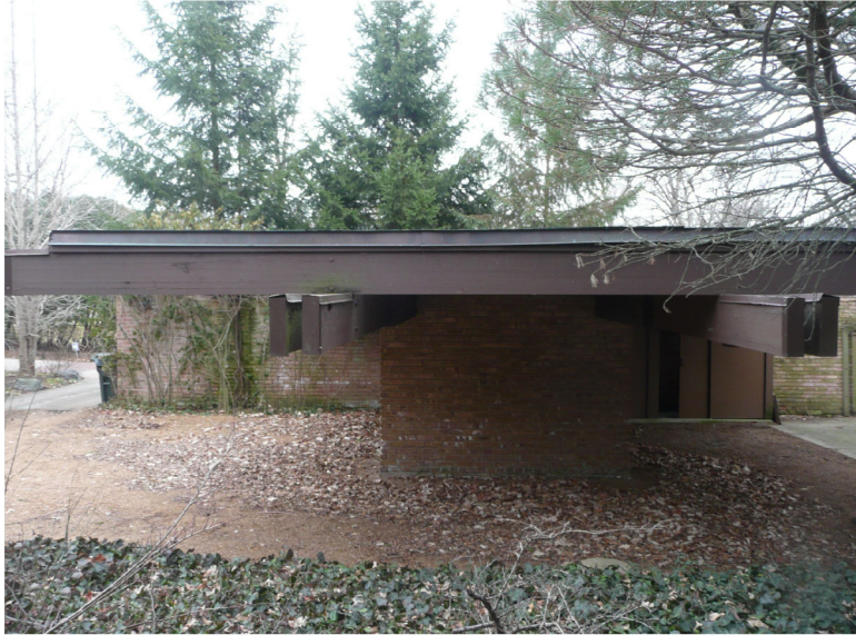
View of carport from house, looking south
