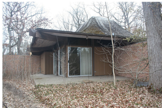
West atrium looking southeast
