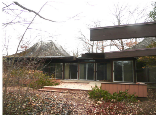
West atrium, south elevation
