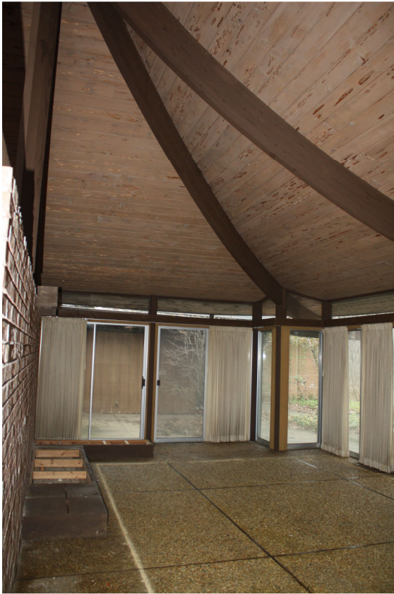
Living room, looking northwest
