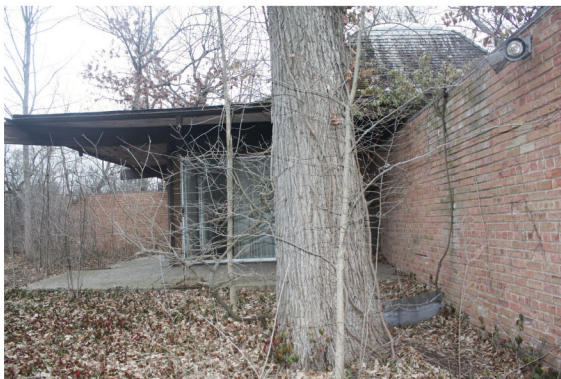
West atrium looking east
