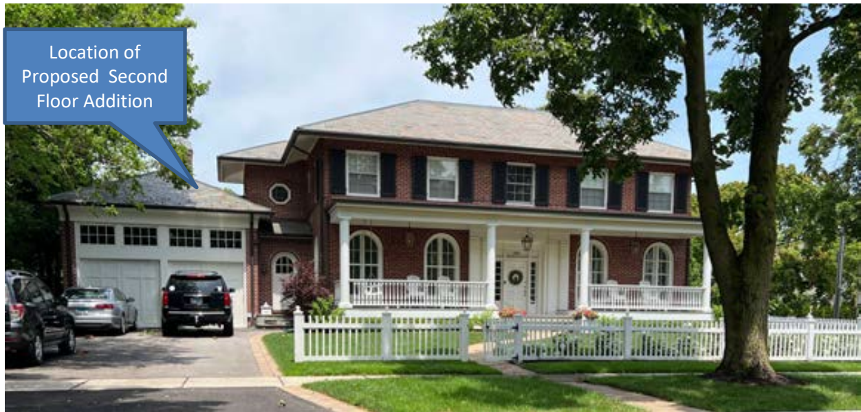
Figure 3 – Subject Property - Front Elevation (Elm Street)
