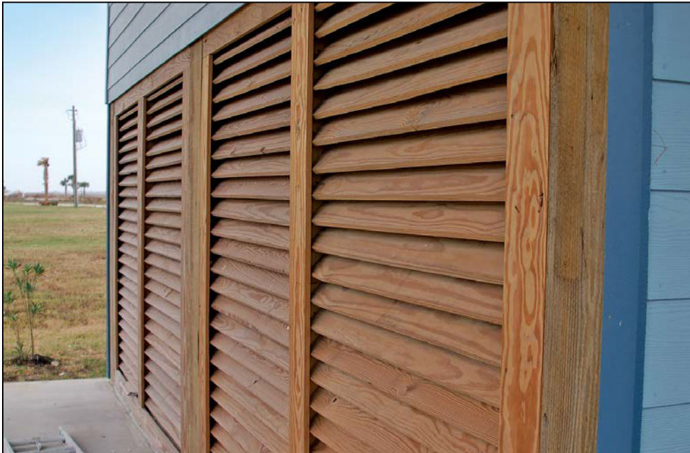
Figure 5: Compliant, fixed, wood louvers installed between pilings
