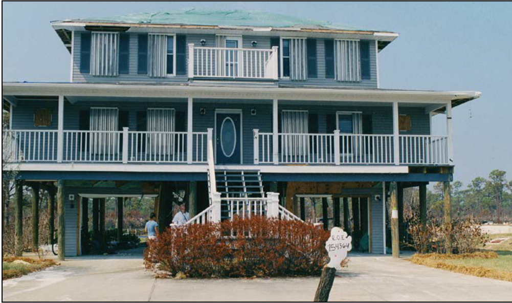
Figure 2: Open stairs, which minimize transfer of flood and wave forces
