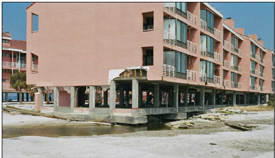
Figure 17: Grade beams that were exposed to flood forces during hurricane-induced scour; grade beams must resist flood, wave, and debris loads when undermined
