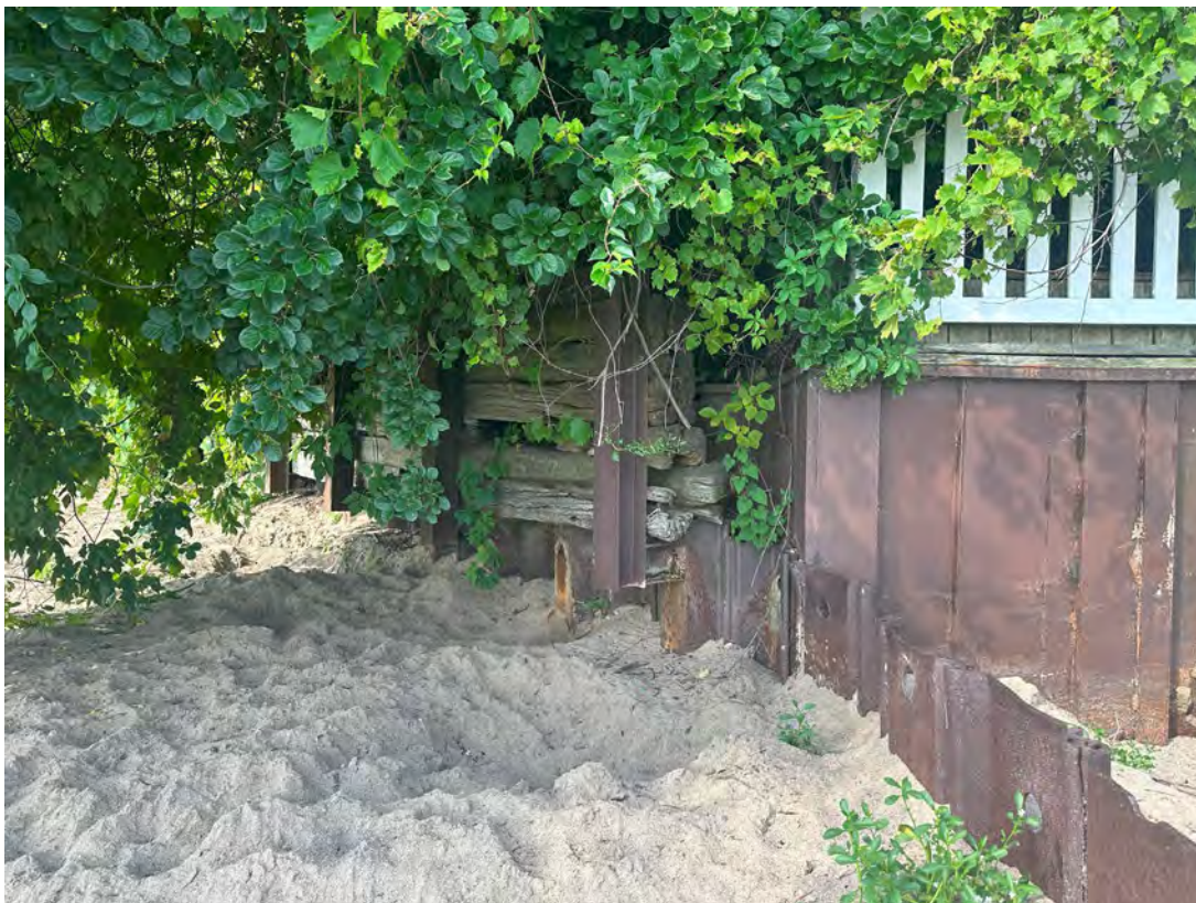
North Seawall (Looking West)
