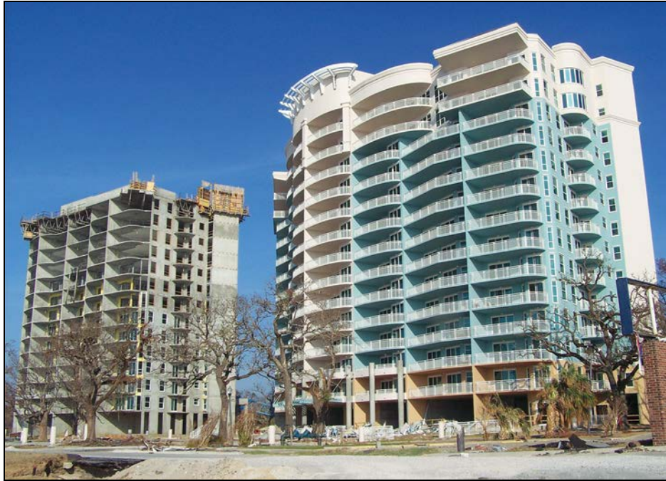
Figure 18: High-rise buildings elevated on shore-perpendicular shear walls
