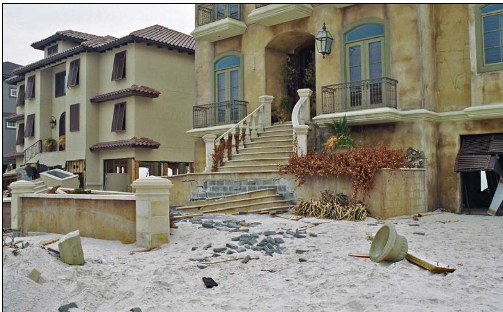
Figure 3: Massive stairs attached to an elevated coastal home, which act as an obstruction
