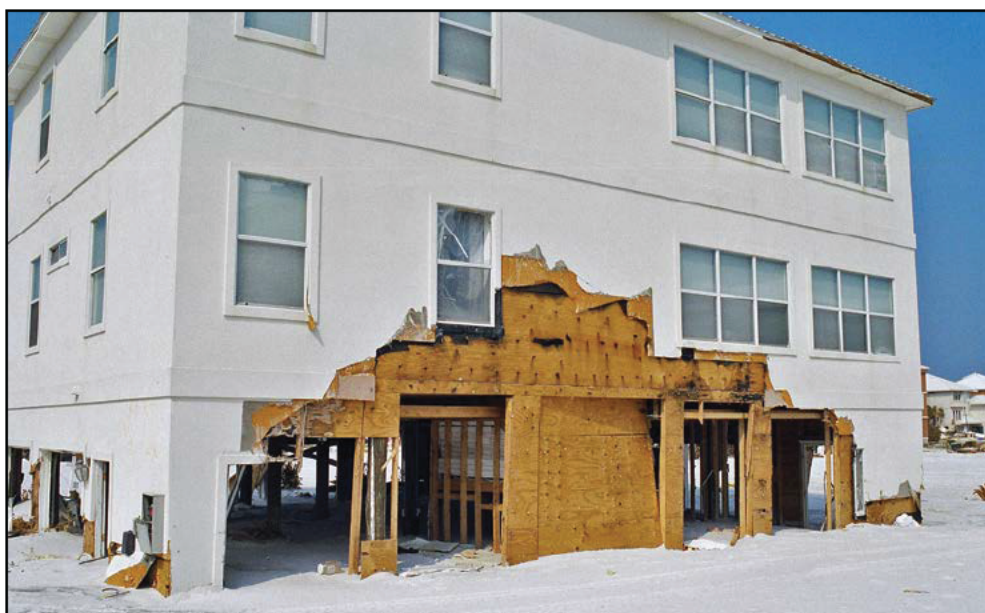
Figure 7: Breakaway wall that did not break away, which led to wave runoff and contributed to flood damage on the side of the elevated building
