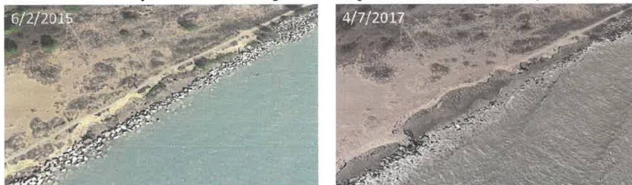
Figure 10. Revetment failure and coastal erosion at Kenosha Dunes State Natural Area. Images obtained from Google Earth for 2015 and 2017.
