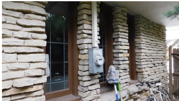
West façade of garage.
