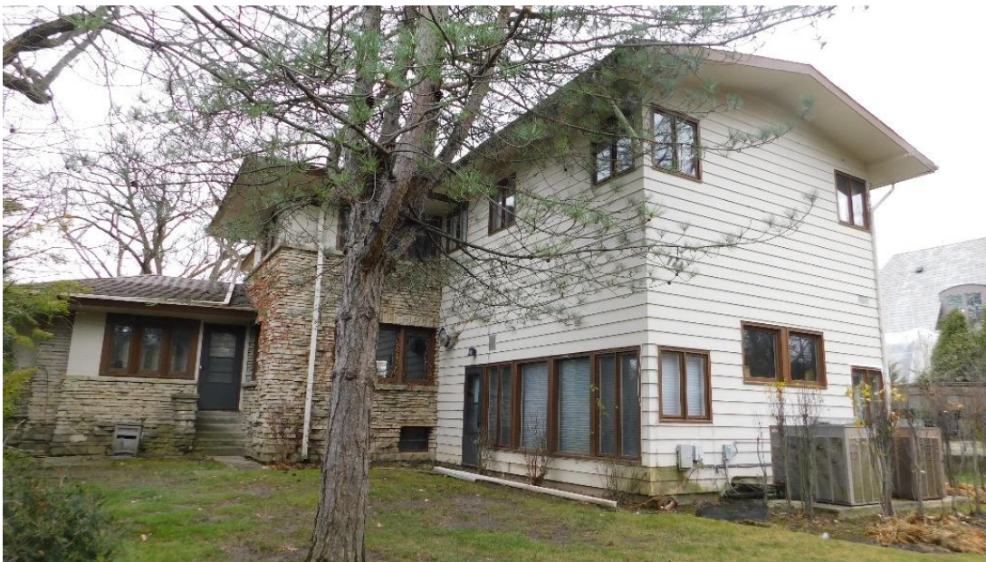
1965 rear addition sheathed in aluminum siding.
