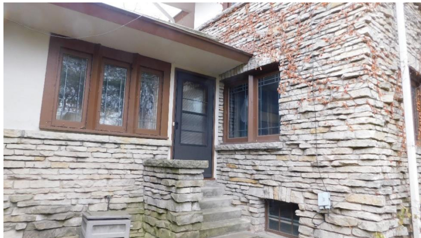
Rear entrance to one-story wing.
