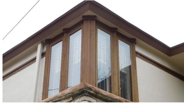
Casement “wraparound” windows above front entrance.
