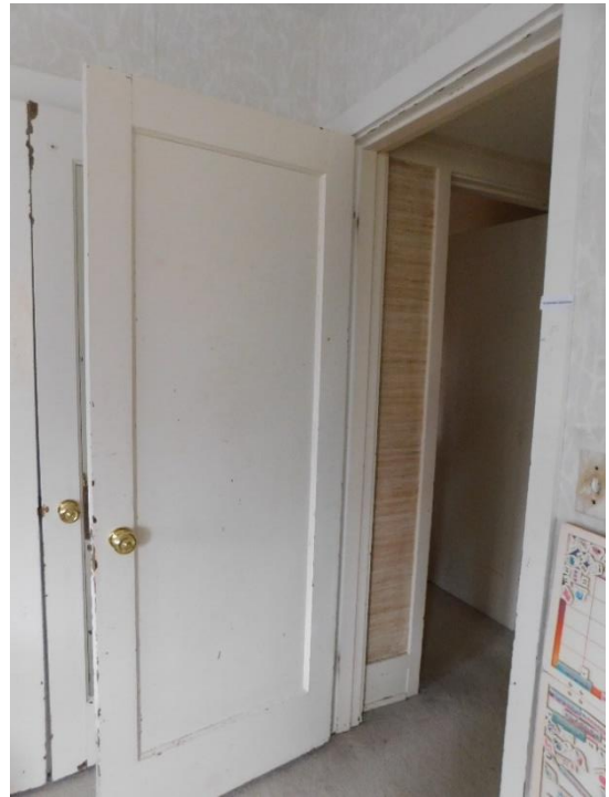
Painted door in Bedroom 3.
