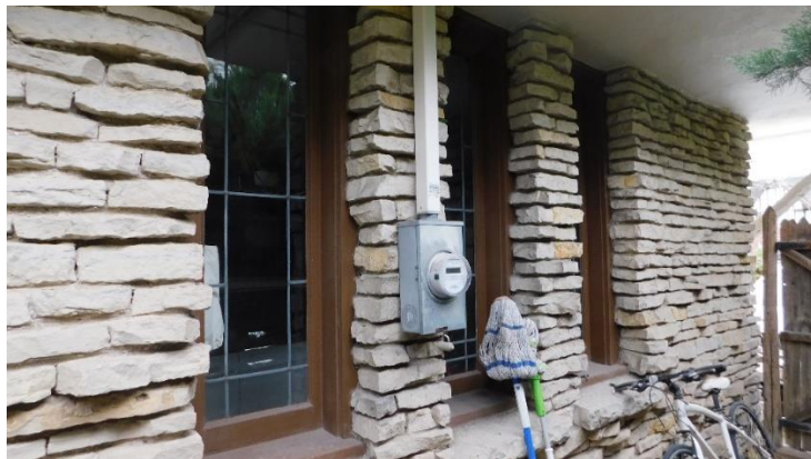
West façade of garage.
