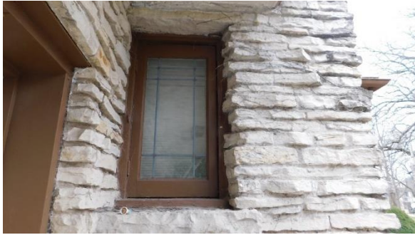
Window adjacent to garage door.
