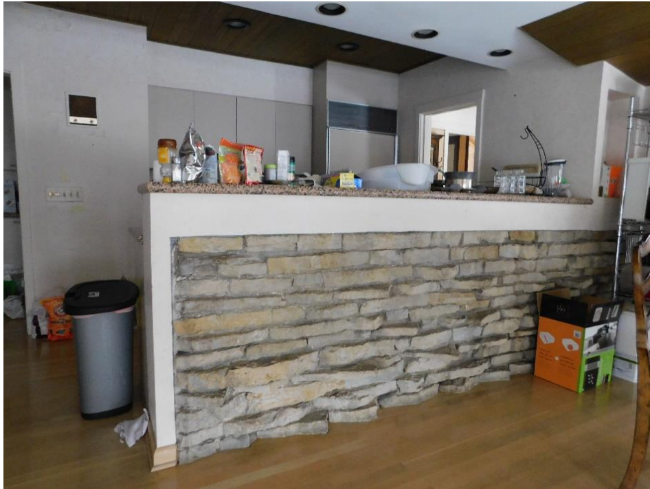
View of island with stratified stonework in kitchen.
