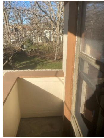
Balcony off the second fl. Office.
