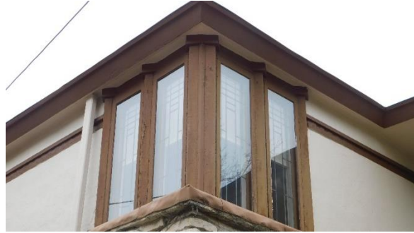
Casement "wraparound" windows above front entrance.
