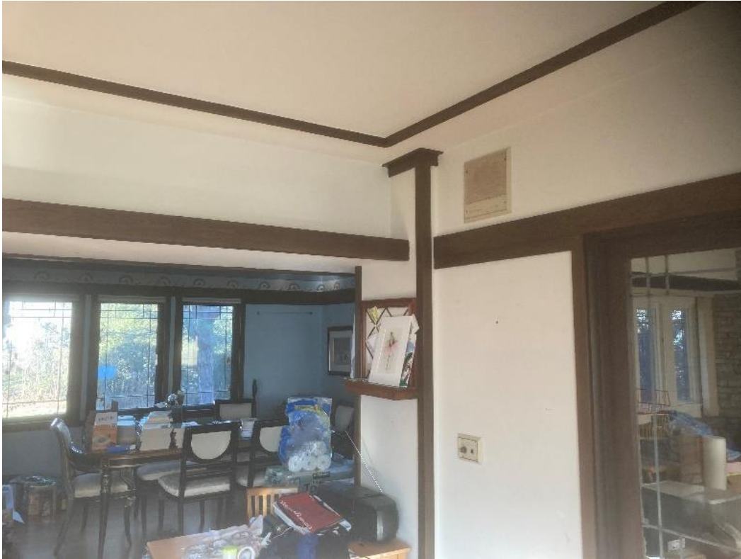
Detail of original wood banding.
