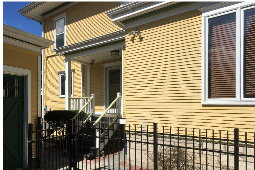
Figure 2 – Subject Property – Existing Rear Porch to be Enclosed
