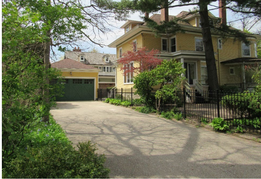
Figure 2 – Subject Property – East Façade From Walnut Street
