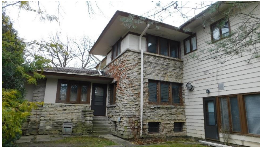
Rear façade of original house block.
