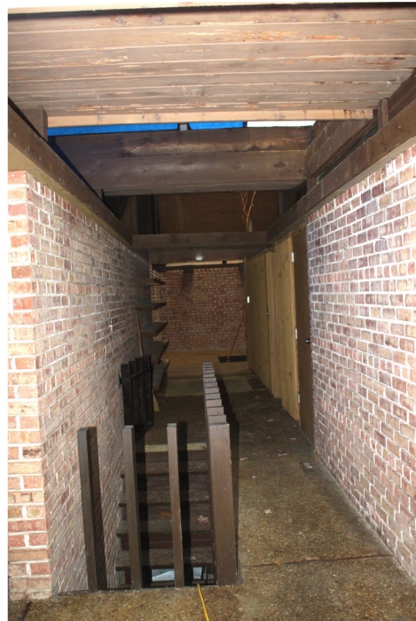
Hall looking west, stairs to basement
