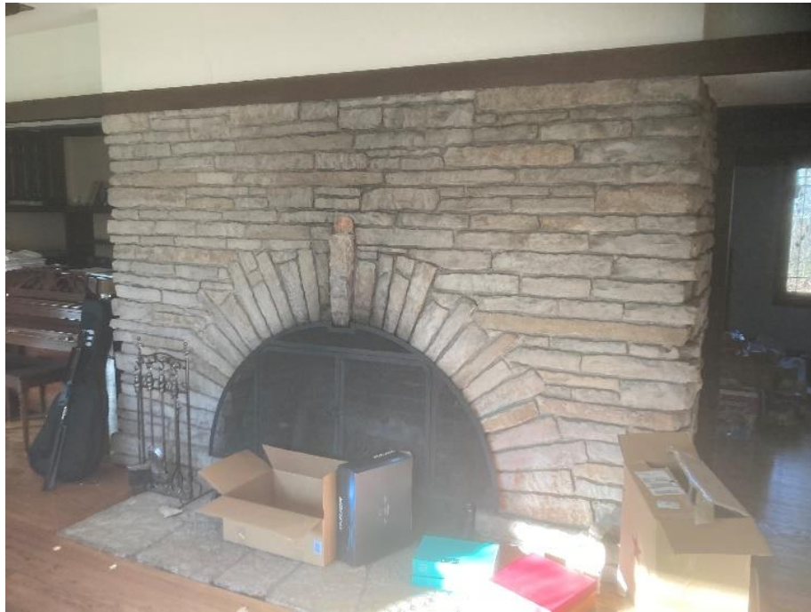
Round arch stone fireplace in living room.
