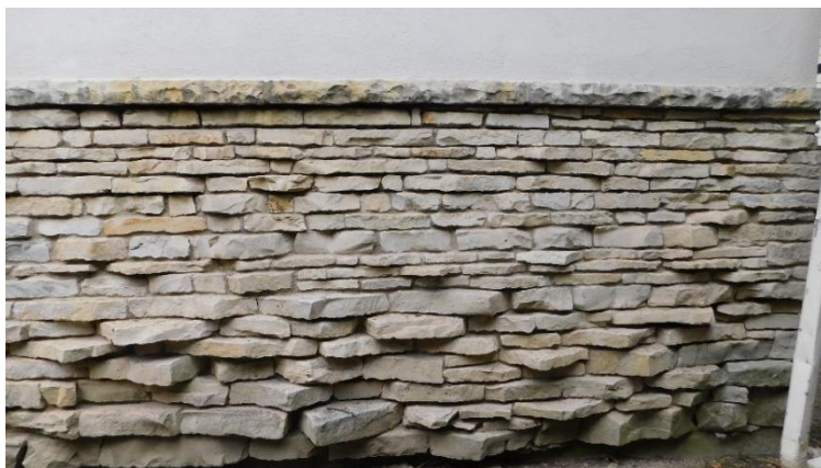
Stonework on east façade.
