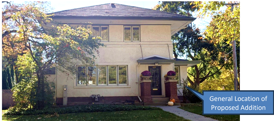
Figure 3 – Subject Property - Front Elevation (Hawthorn Lane)
