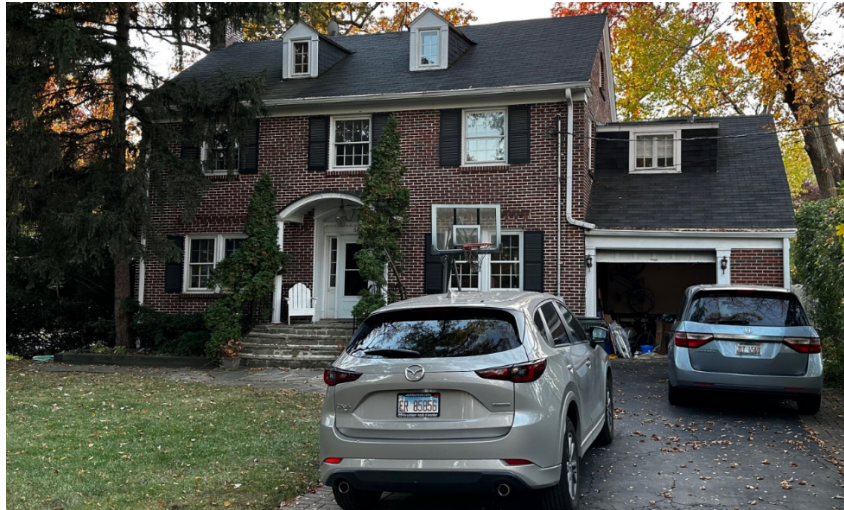
Figure 3 – Subject Property – East Front Elevation (Walden Road)
