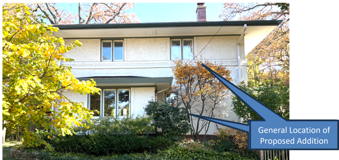
Figure 5 – Subject Property – Corner Elevation (Woodland Avenue)
