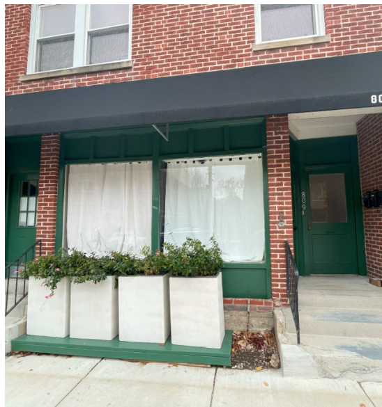
Figure 3 – Subject property – Newly painted storefront and movable planters.
