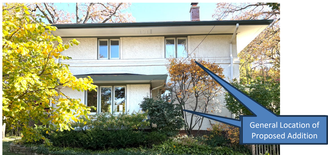
Figure 5 – Subject Property – Corner Elevation (Woodland Avenue)
