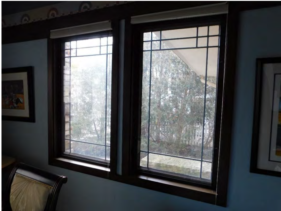
Detail of original casement windows in dining room.
