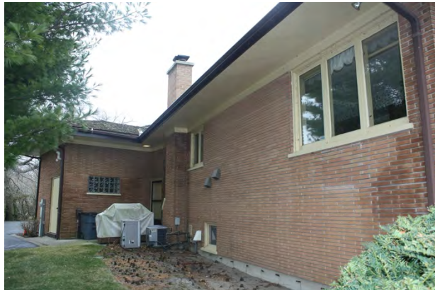
South elevation, looking northwest
