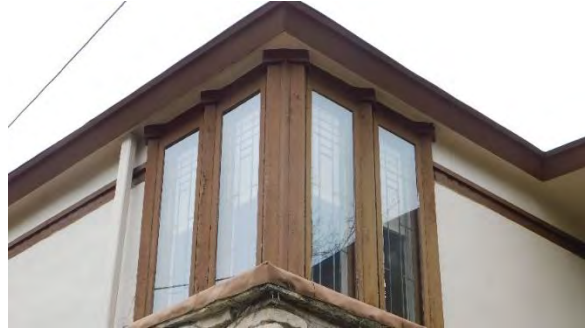
Casement “wraparound” windows above front entrance.
