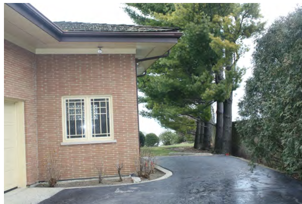
South elevation looking east, garage on left
