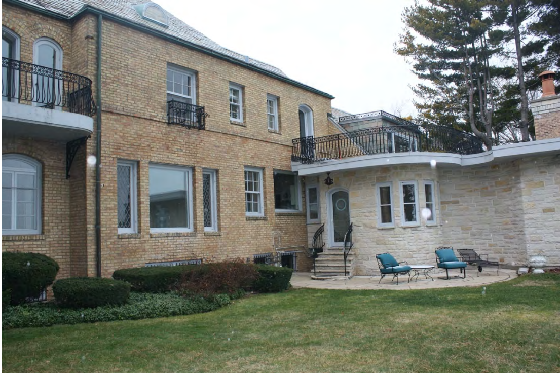
East elevation, looking northwest
