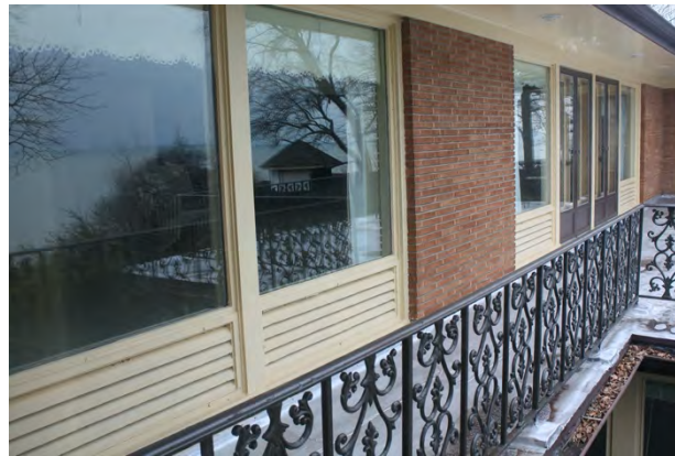
East elevation, second floor balcony, looking north
