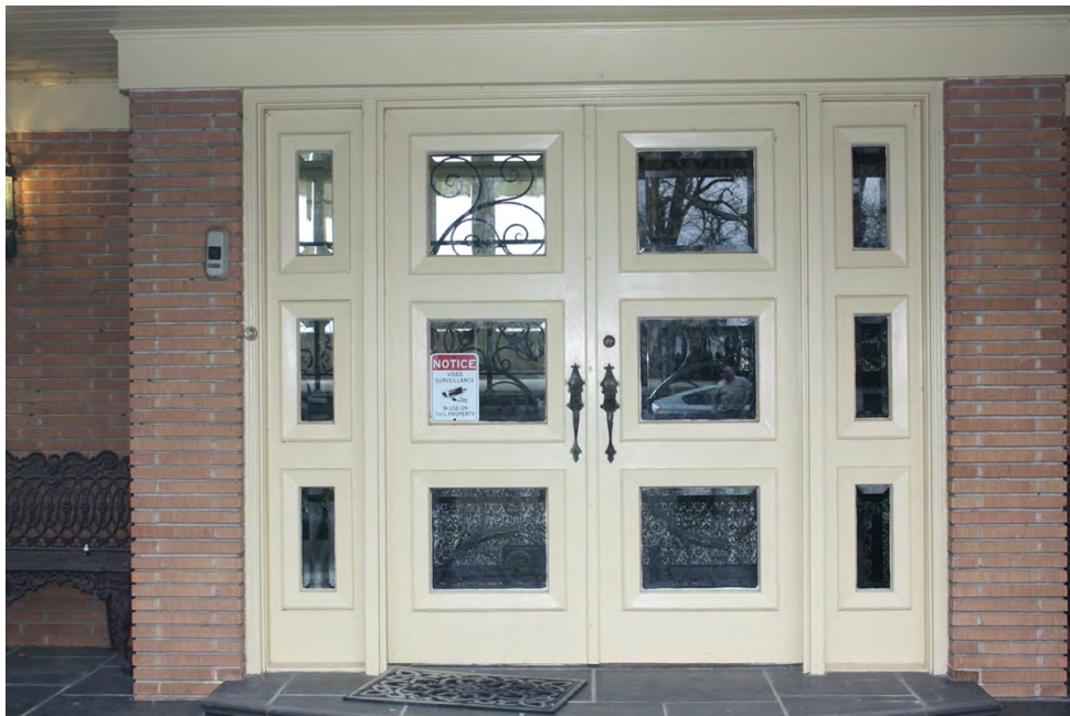
West elevation, front entry
