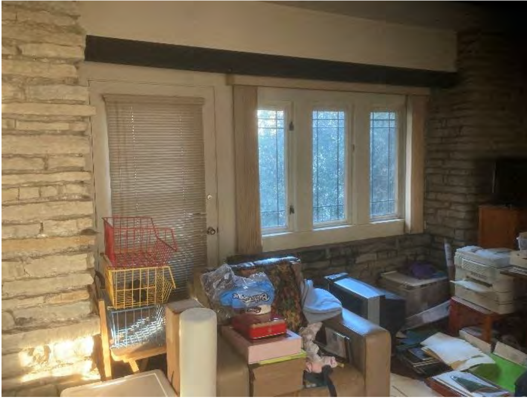
View of den's exterior door and strip of three original leaded glass casement windows
