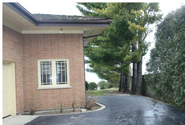
South elevation looking east, garage on left
