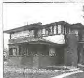
21. Harry B. Roberts Residence 344 Elm Place • 1929 Note the detail of the windows that appear to wrap around the corner. Wright also used this detail in his designs of the time.
