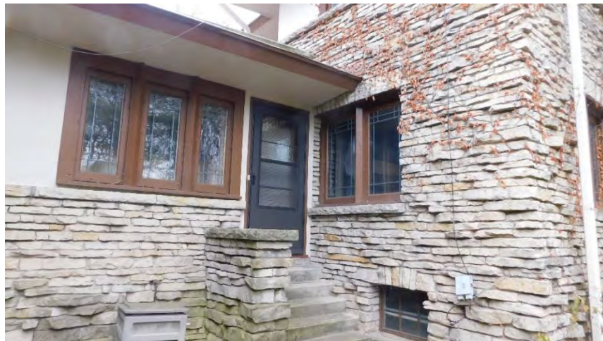
Rear entrance to one-story wing.
