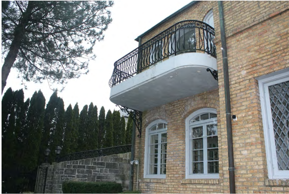
East elevation, south side, 1976 balcony addition
