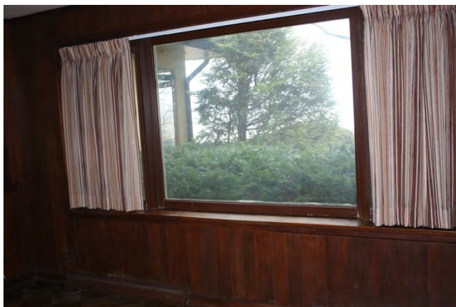
Lower level office, east wall
