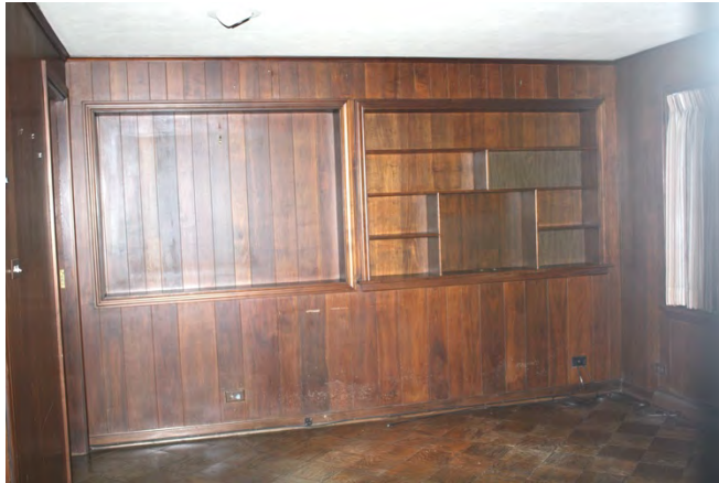
Lower level office, north wall
