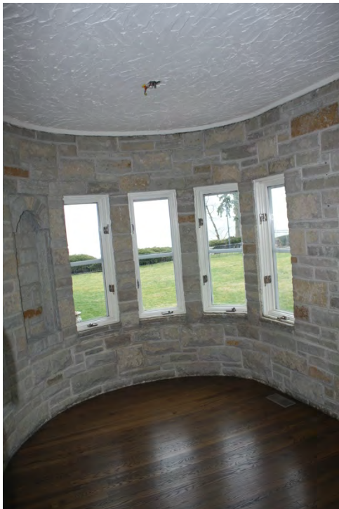
Porch addition, south side looking east
