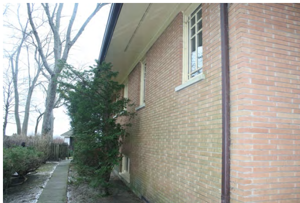
North elevation, looking east
