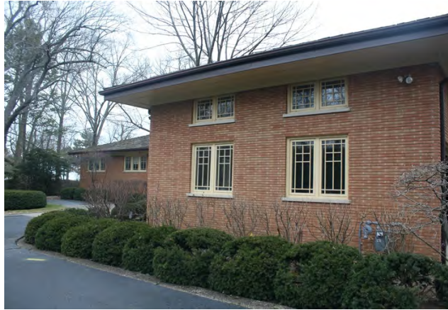
West elevation, south side
