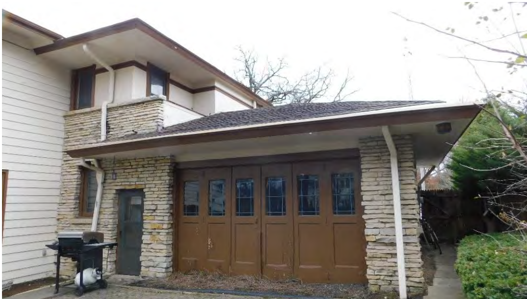
Rear façade of garage showing original paired doors.
