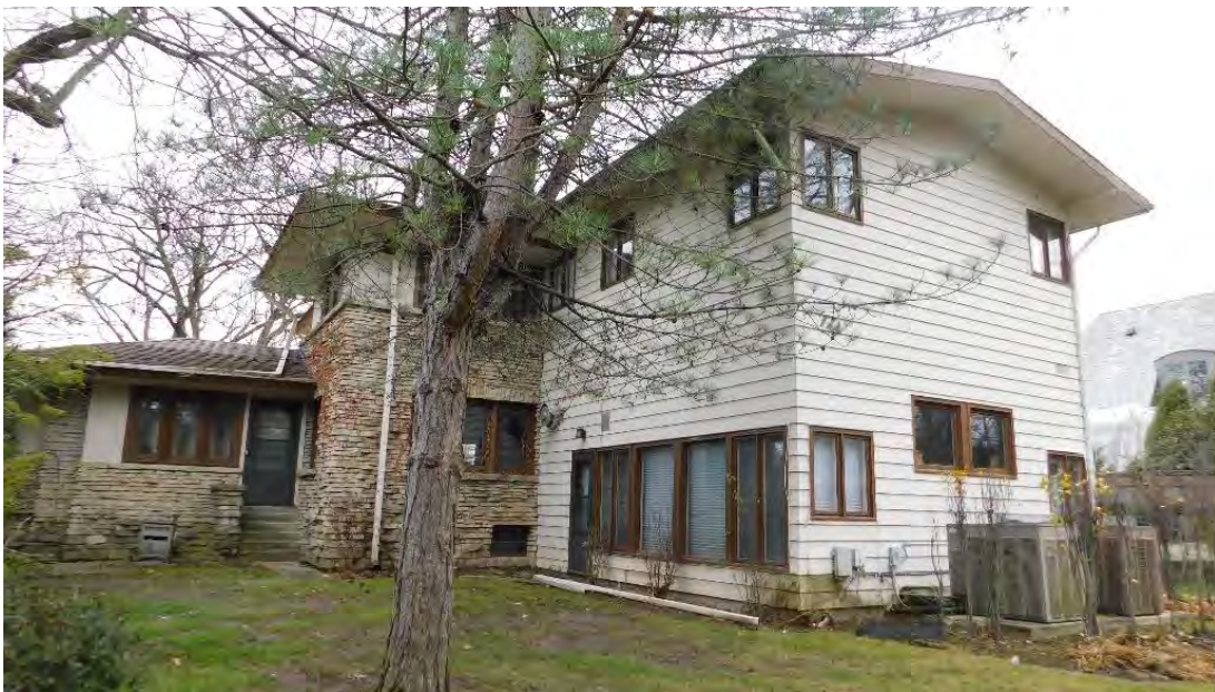
1965 rear addition sheathed in aluminum siding.
