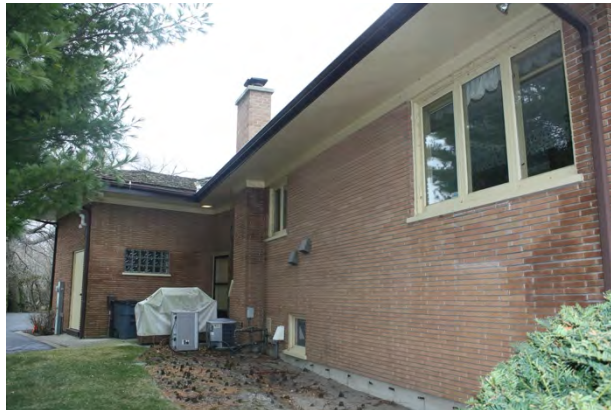
South elevation, looking northwest
