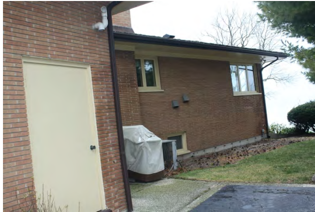
South elevation, east side, looking northeast
