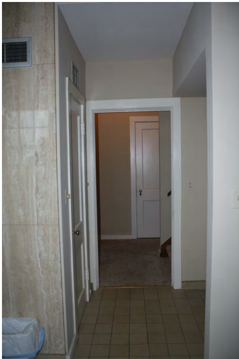
Kitchen, west wall, looking through hall to door to front entry hall
