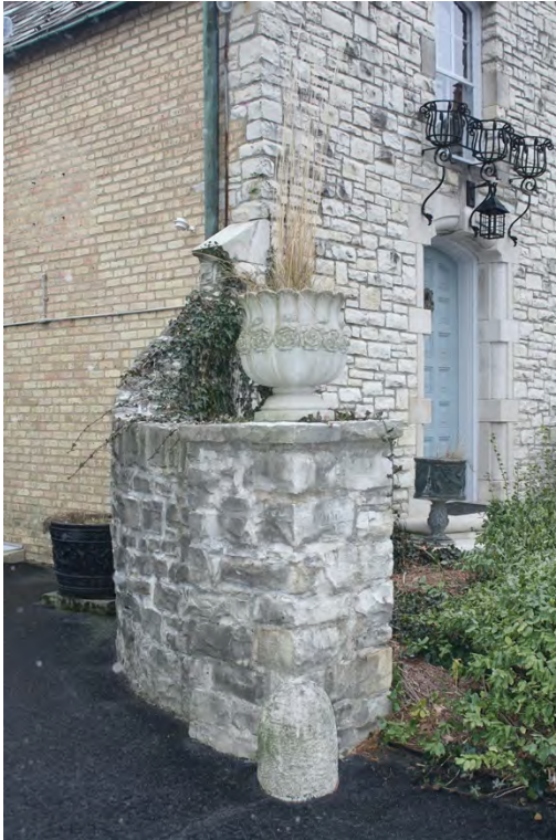
Wall at northwest corner of house
