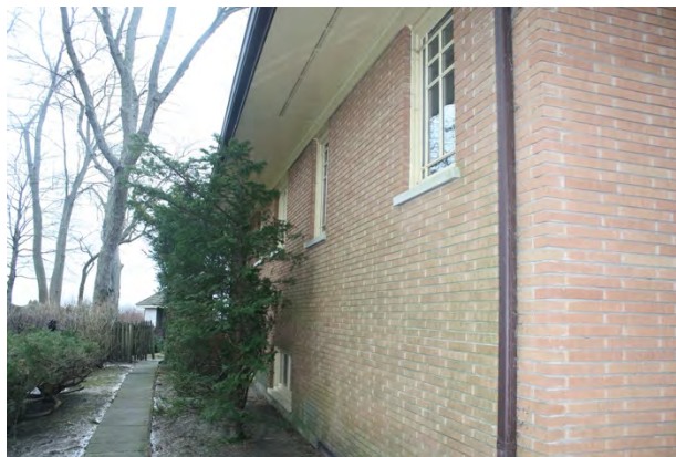
North elevation, looking east
