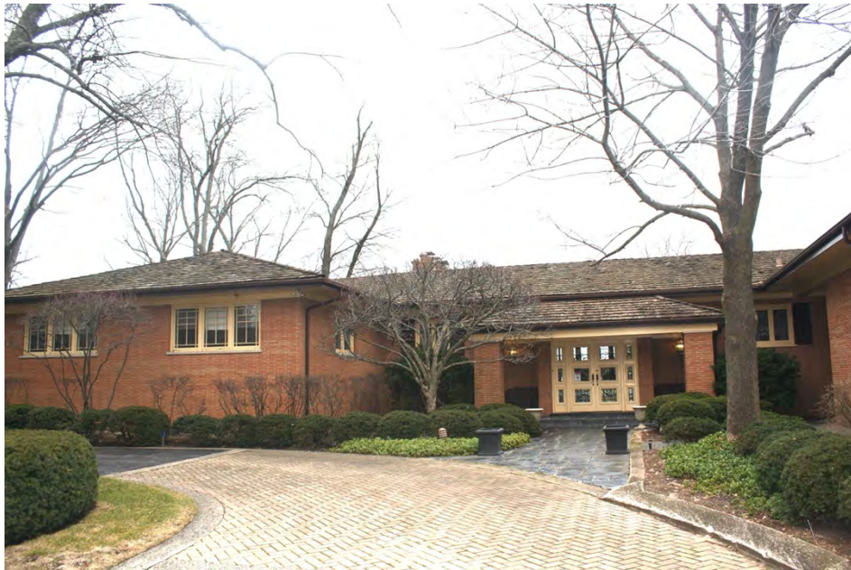
West elevation, front entry
