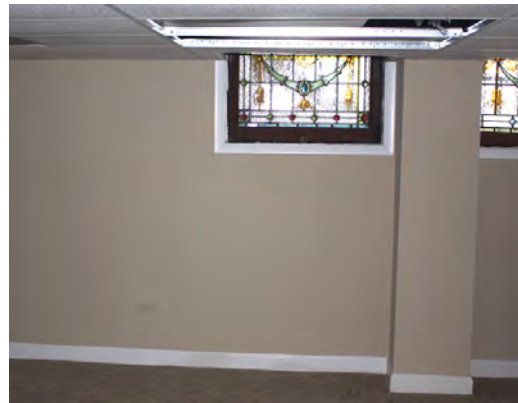
Basement, east wall
