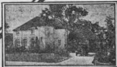
Residence of Mrs. Henrietta Huszagh, 203 Sheridan Road, Winnetka. 9 rooms, 2-car garage. Fuel cost all winter, $268
