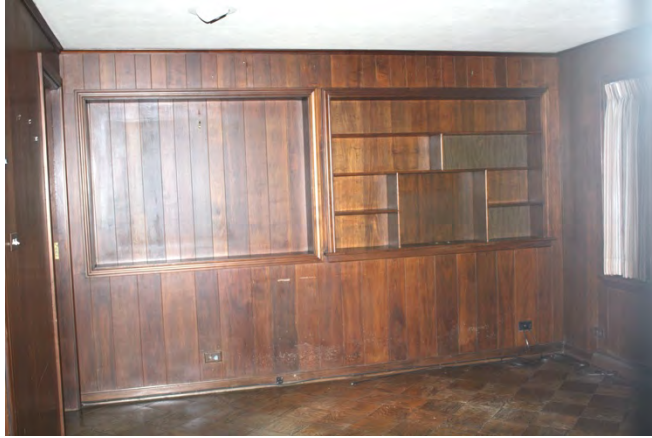
Lower level office, north wall
