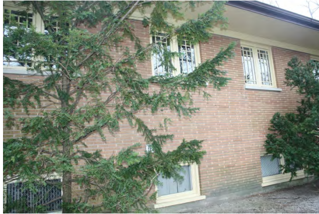
North elevation looking west
