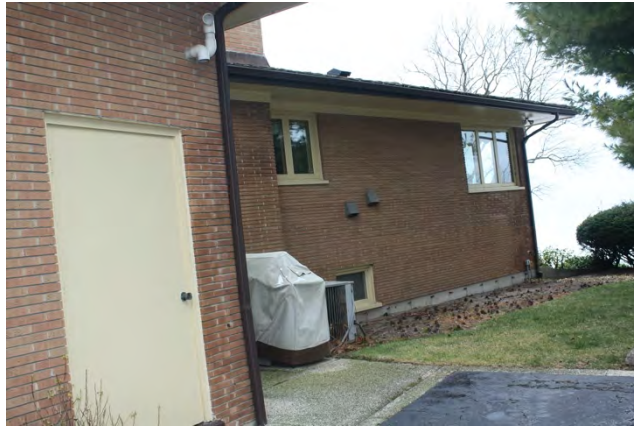
South elevation, east side, looking northeast
