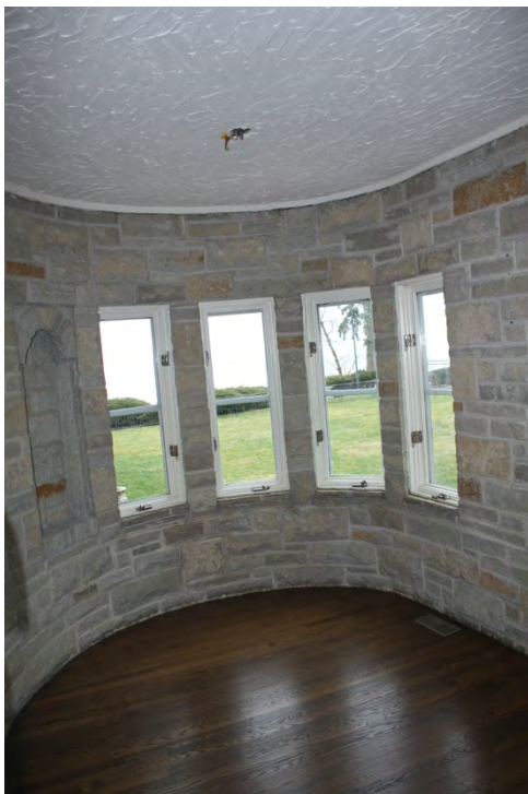
Porch addition, south side looking east
