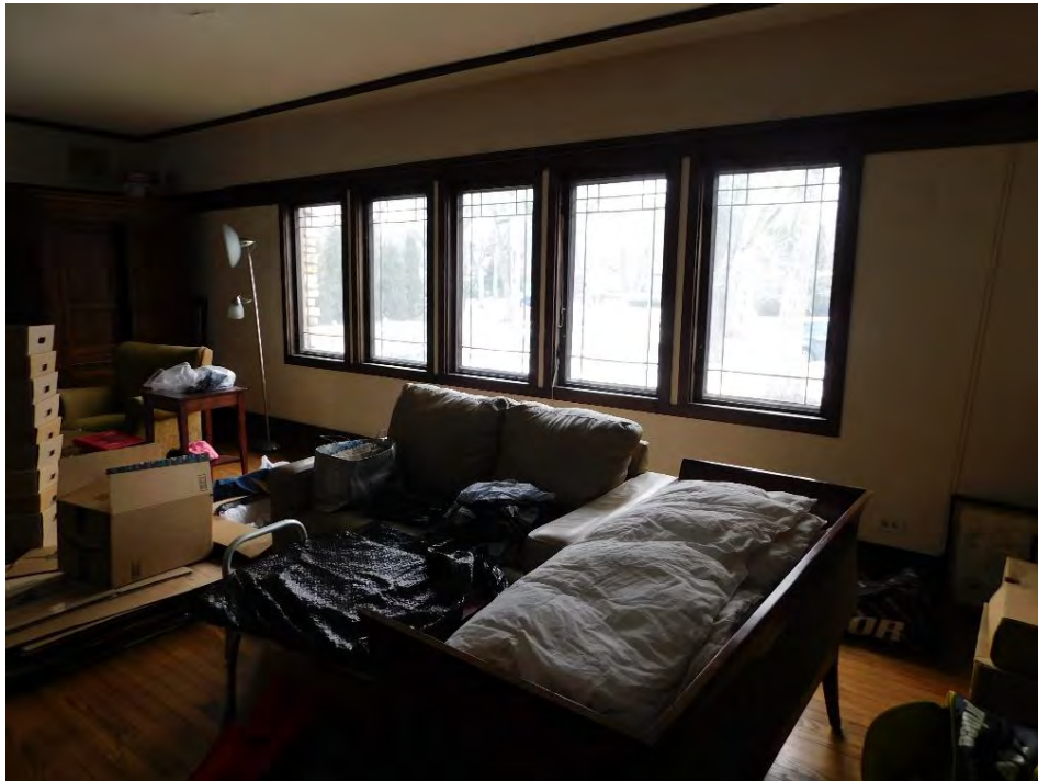
Strip of original five casement windows in living room.
