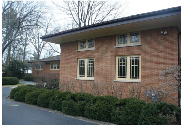
West elevation, south side
