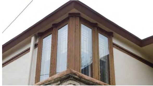
Casement “wraparound” windows above front entrance.
