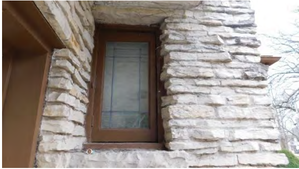
Window adjacent to garage door.
