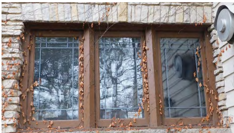
Group of leaded glass casement windows on rear façade of original house.
