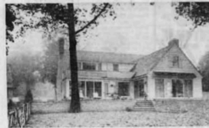
Exterior of the attractive home on which the Penningtons and Architect Ralph Hunsath pooled ideas and changed their minds several times before arriving at perfection.
