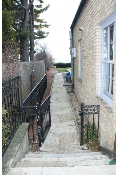
Steps to back yard, north elevation, looking east
