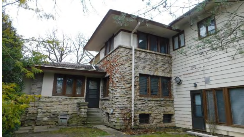
Rear façade of original house block.
