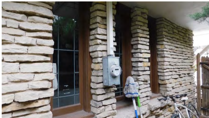
West façade of garage.
