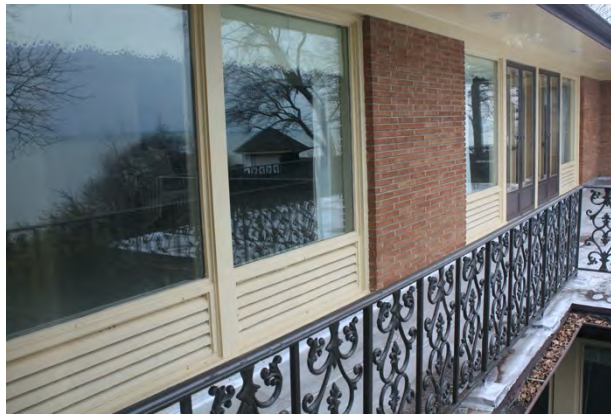
East elevation, second floor balcony, looking north
