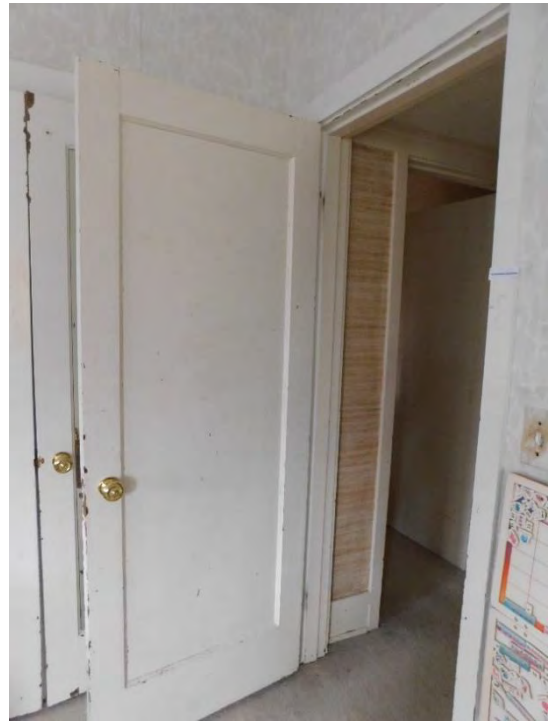
Painted door in Bedroom 3.
