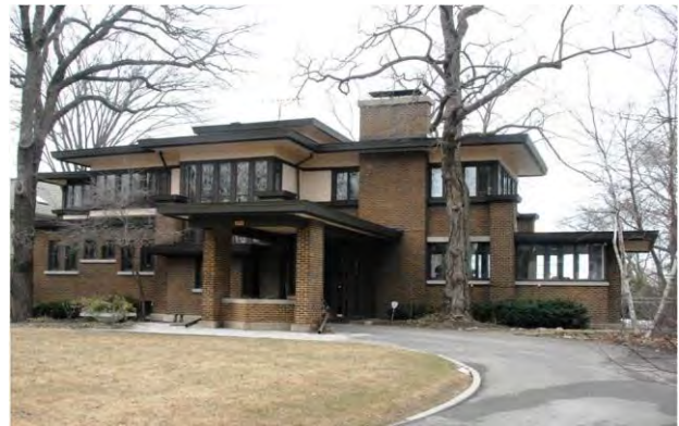
A. Bersbach House (1914) at 1120 Michigan Avenue, Wilmette.
