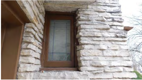
Window adjacent to garage door.
