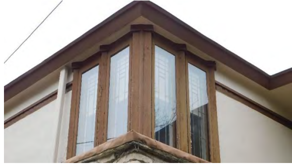
Casement “wraparound” windows above front entrance.
