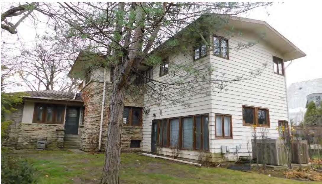
1965 rear addition sheathed in aluminum siding.
