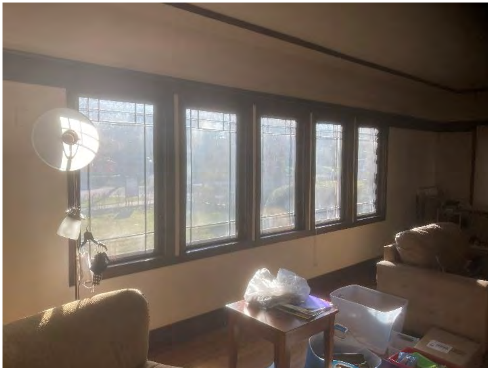
Original leaded glass casement windows illuminating the living room.
