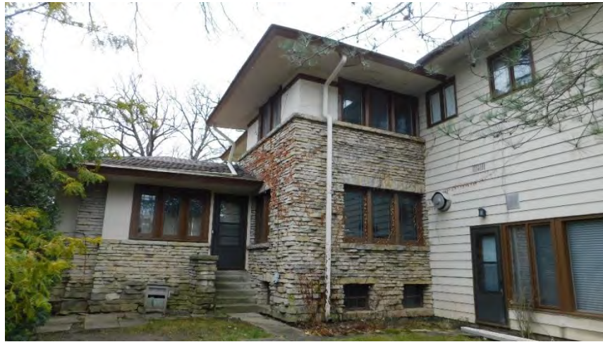
Rear façade of original house block.
