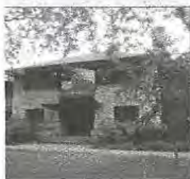
1. Braeside School & Additions 150 Pierce Road • 1927
