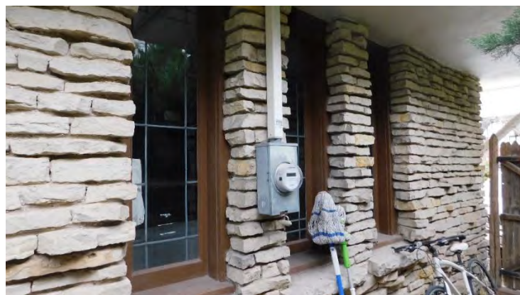
West façade of garage.
