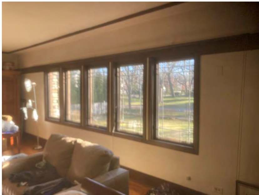
South wall of living room with strip of five original leaded glass casement windows.
