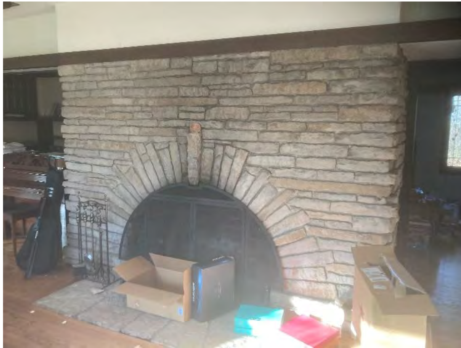
Round arch stone fireplace in living room.
