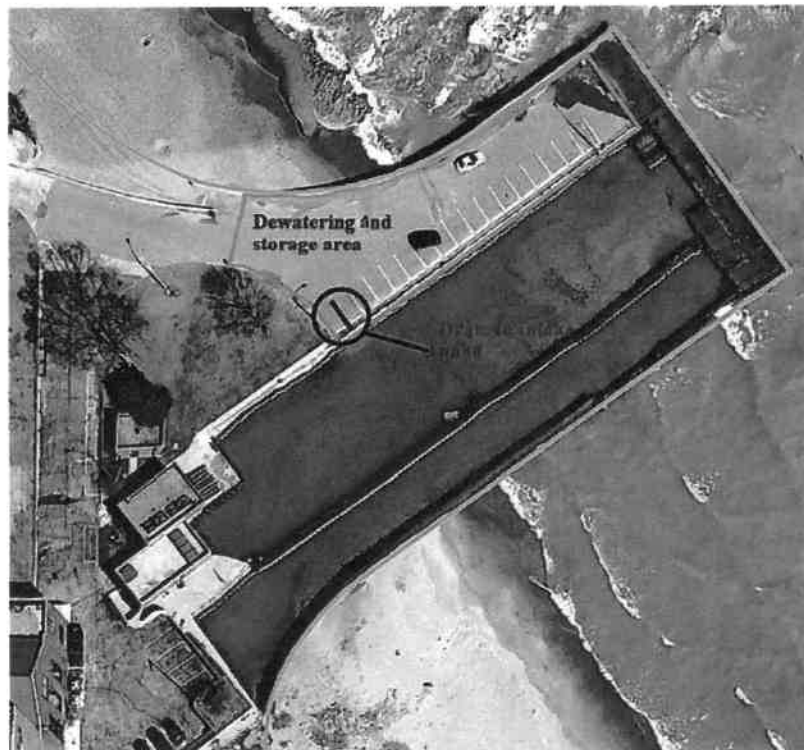
Dewatering And Storage Area – Adjacent To Intake Pond
