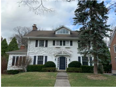
Front Façade, south elevation
