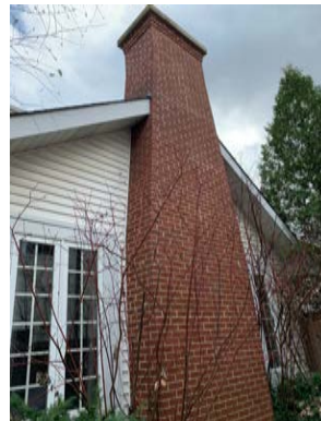
West elevation, non-historic chimney
