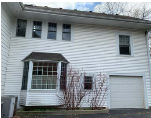
East elevation of north projecting wing
