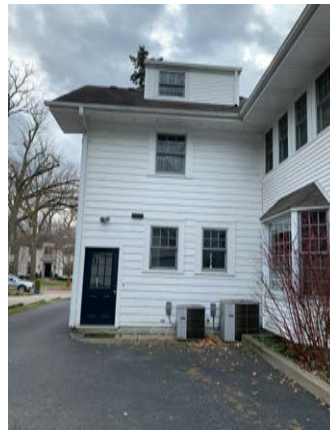
North elevation, east side
