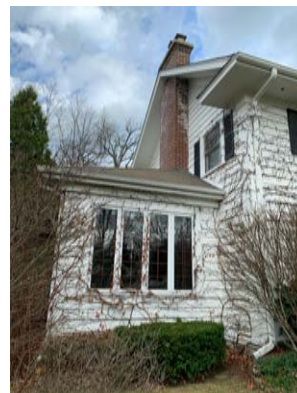
South elevation, west side
