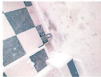
Photo 2c: Moisture on baseboards in the rear living room.
