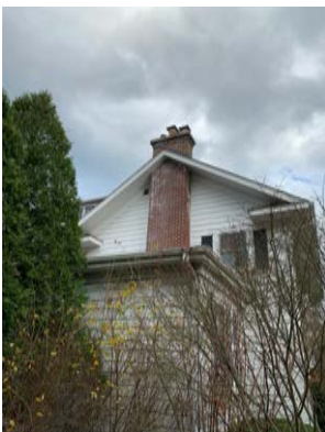
West elevation, historic chimney
