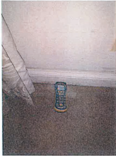
Photo 2c: Moisture on baseboards in the rear living room.
