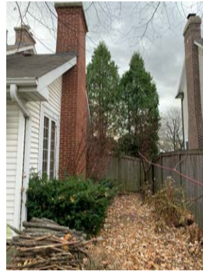
West elevation, looking south
