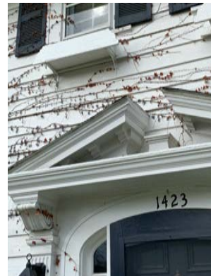
Pediment details above front door
