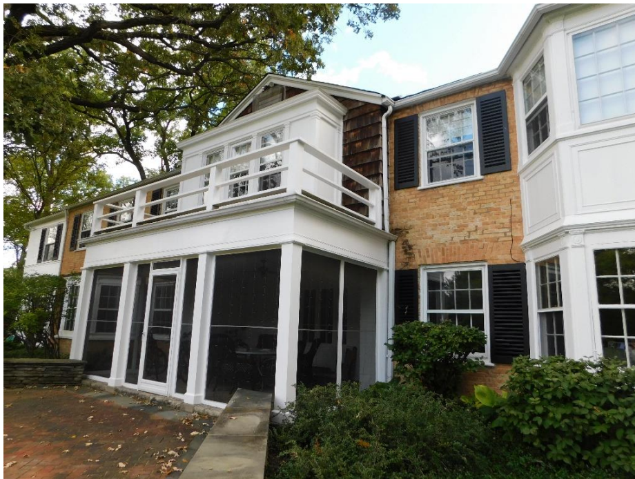
Screened-in rear porch.
