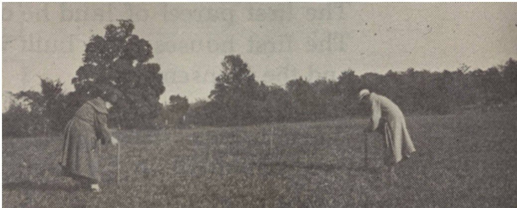
Eleanor Torbet and Florence Aitkin setting stakes for the Torbets' Home, the "first foundation to be dug in Bannockburn." Undated photograph, Bannockburn Beginnings , 18.
