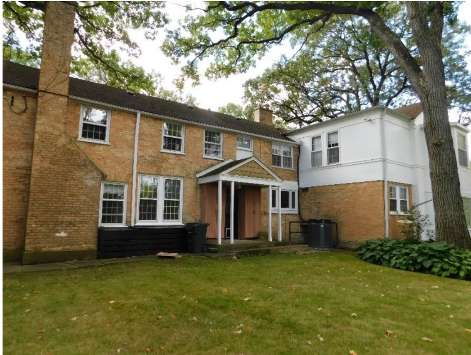
North façade, looking southwest.
