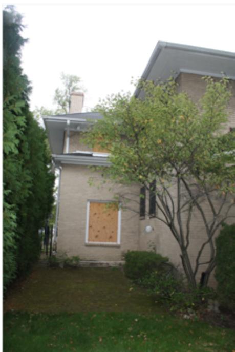
South elevation, west side, looking north
