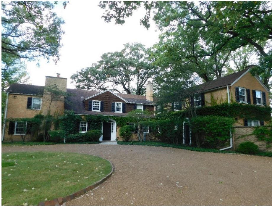
Front façades of main block and east wing, view looking northwest.
