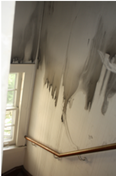
Second Floor rear staircase
