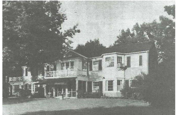
Rear façade showing one-story north wing on the left, which was added in 1932, and the original balustrade above the screen-in porch.
