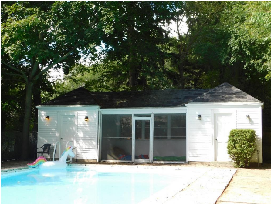
View of pool house, looking southwest.
