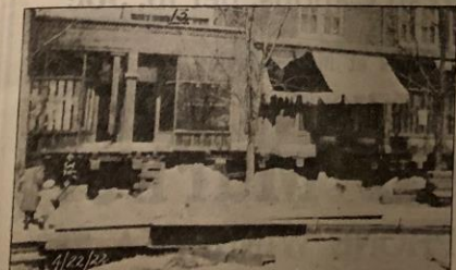
"It couldn't be done," but here is a section of the old building before it was dropped on the new foundation. Looks like a cyclone did it.
