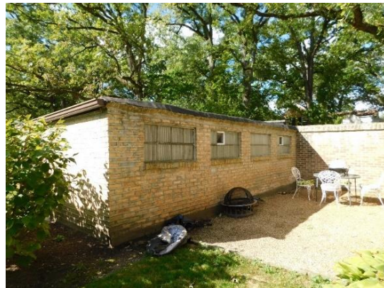
North façade of storage building.
