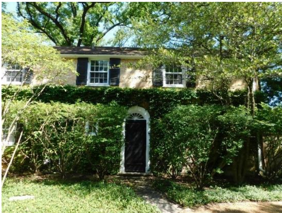
Front entrance to east wing.
