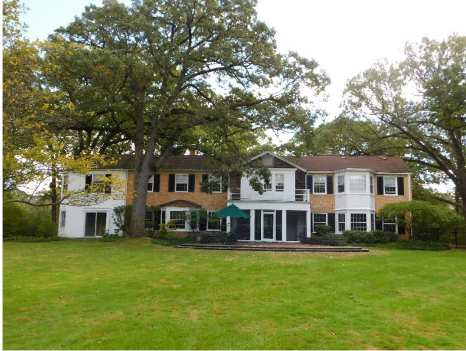
Rear façade, looking east.
