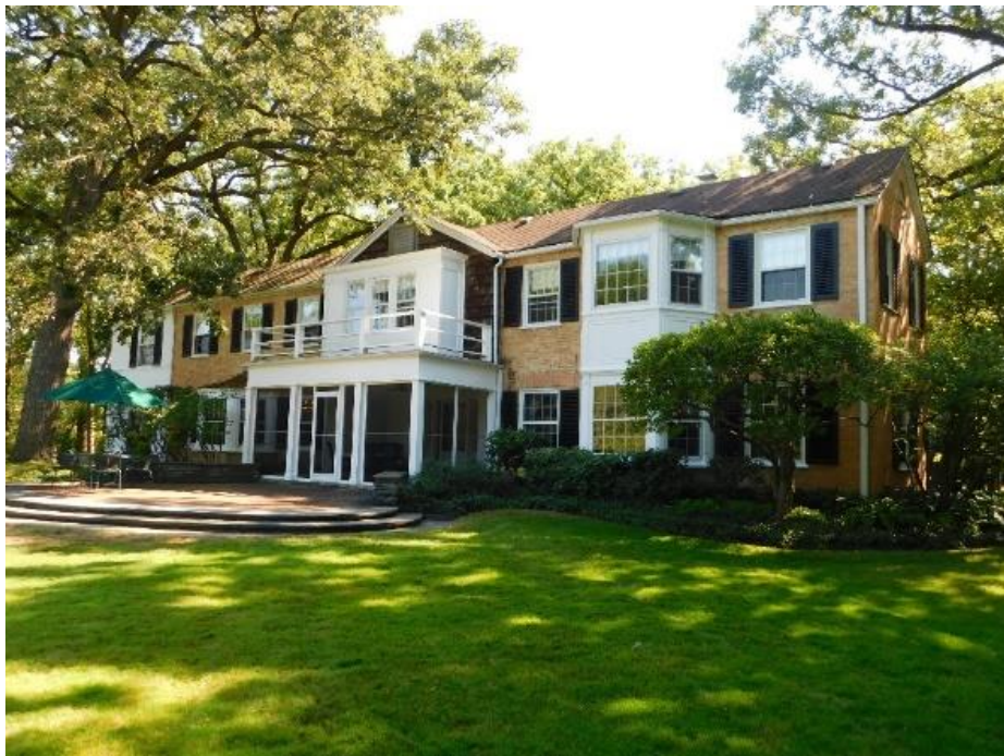
Rear façade, looking northeast.
