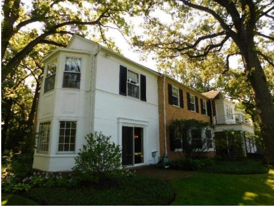
Rear façade, looking southeast.
