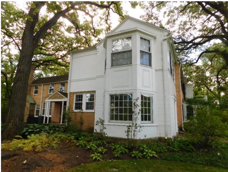
North façade, looking southeast.
