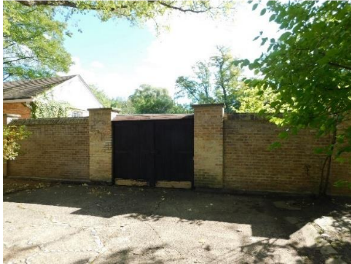
Storage building with flanking brick walls.
