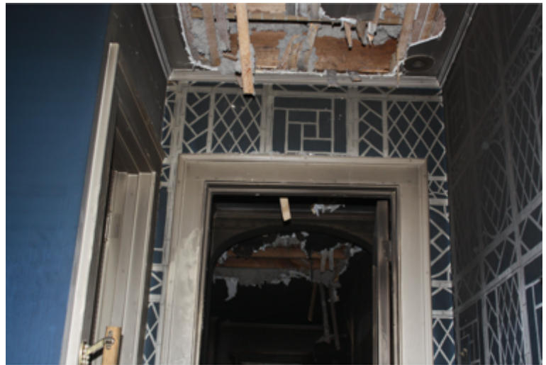
Second floor hallway facing master bedroom, looking east
