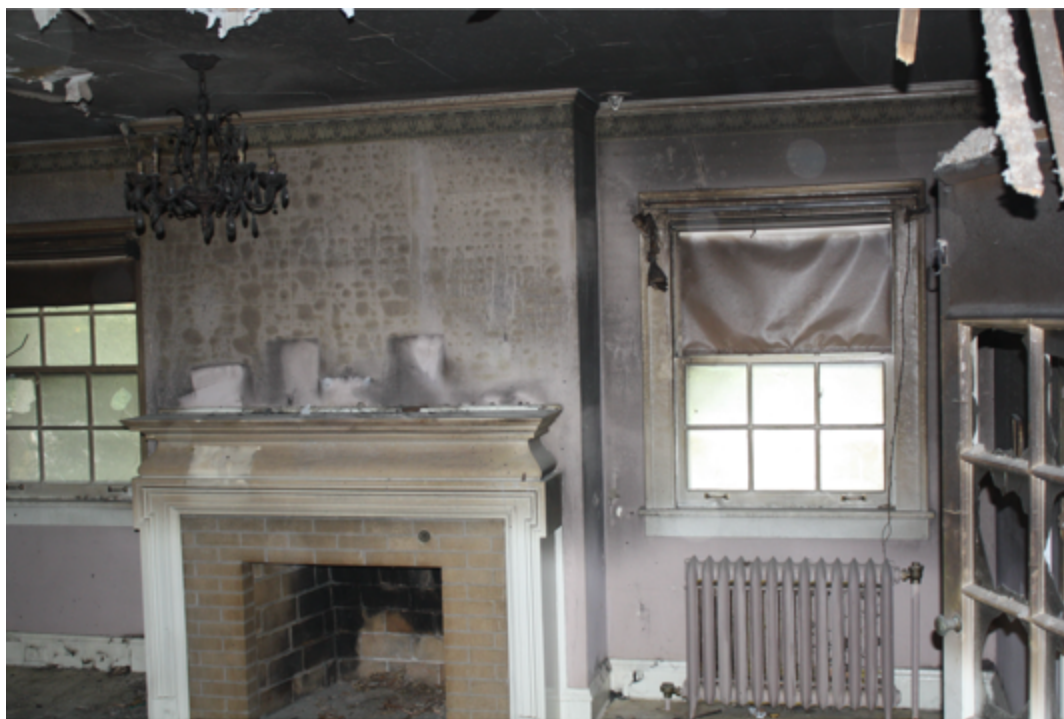
Master Bedroom, looking east
