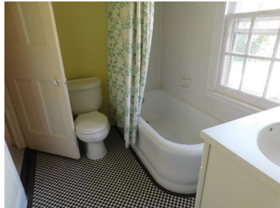
Second floor bathroom.
