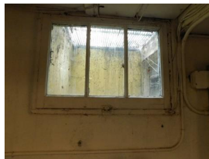
Views of basement.
