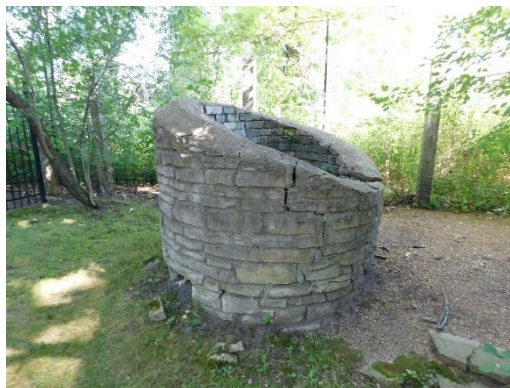
Stone well on west side of coach house.
