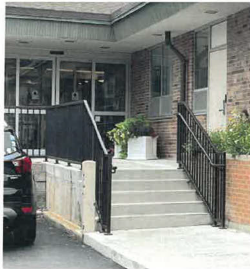
Existing South Entrance - Painted Steel Railings - FRP Door in Aluminum Frame
