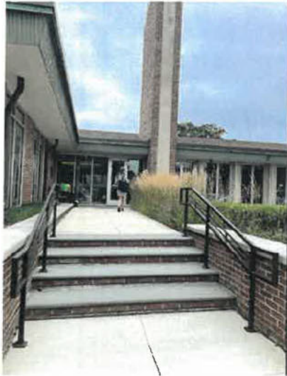
Existing North Entrance - Painted Steel Railings
