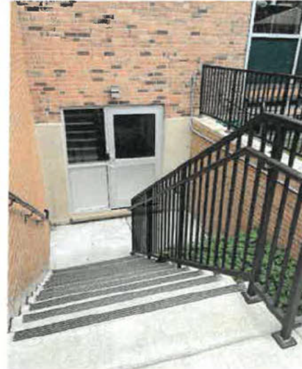
Existing Staff Exit - Painted Steel Railings - Aluminum Door and Frame
