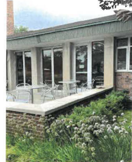
Existing Meeting Room (North Facade) - Aluminum Door and Frame
