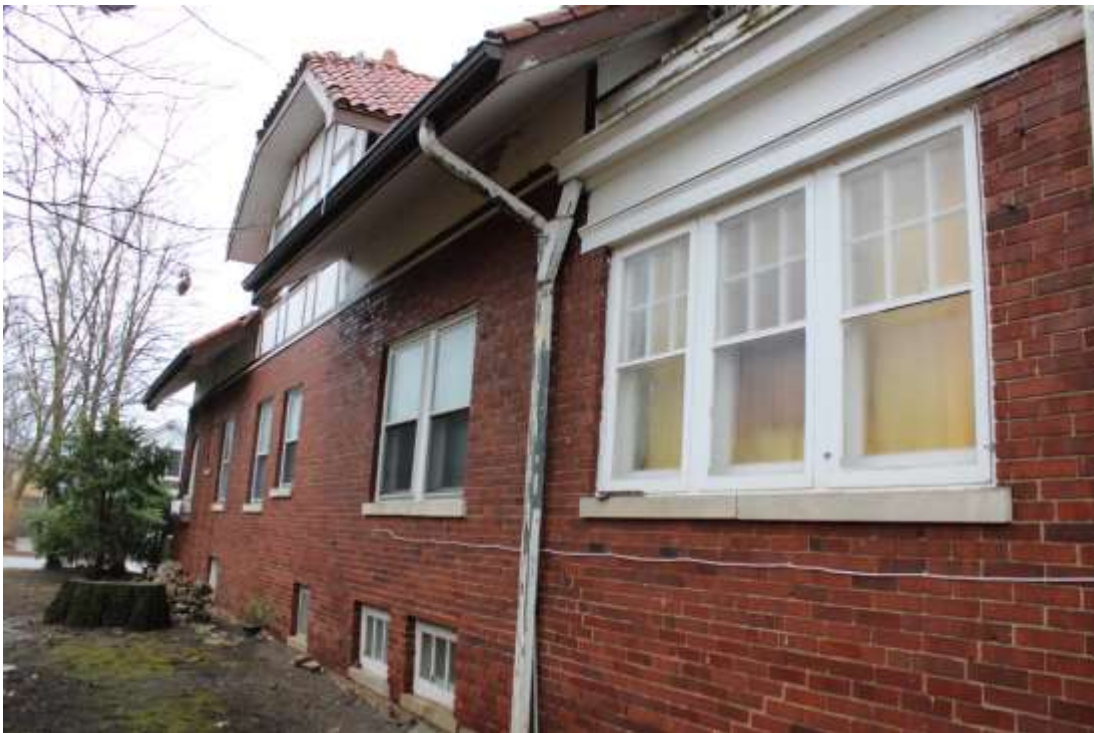
West façade, view northeast.
