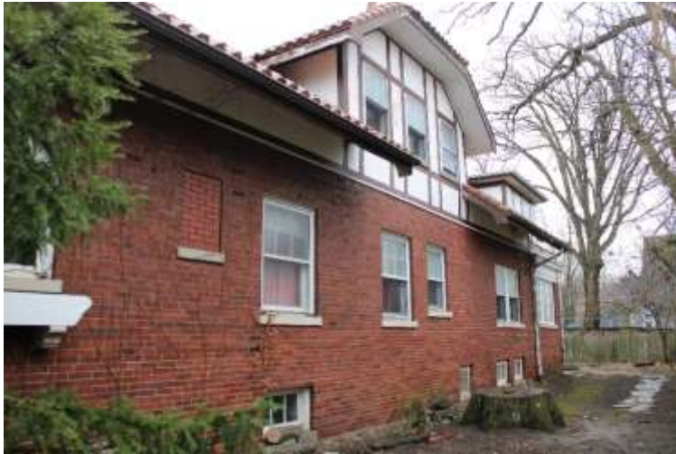
West façade, view southeast.
