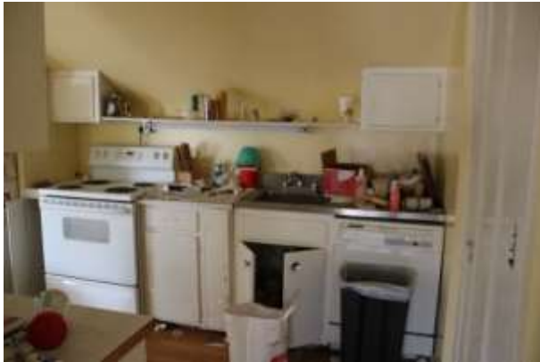
Second floor Kitchen, view southwest.
