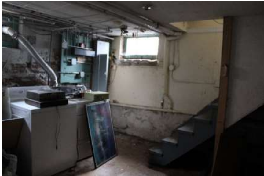
Basement, view southeast toward stairway.
