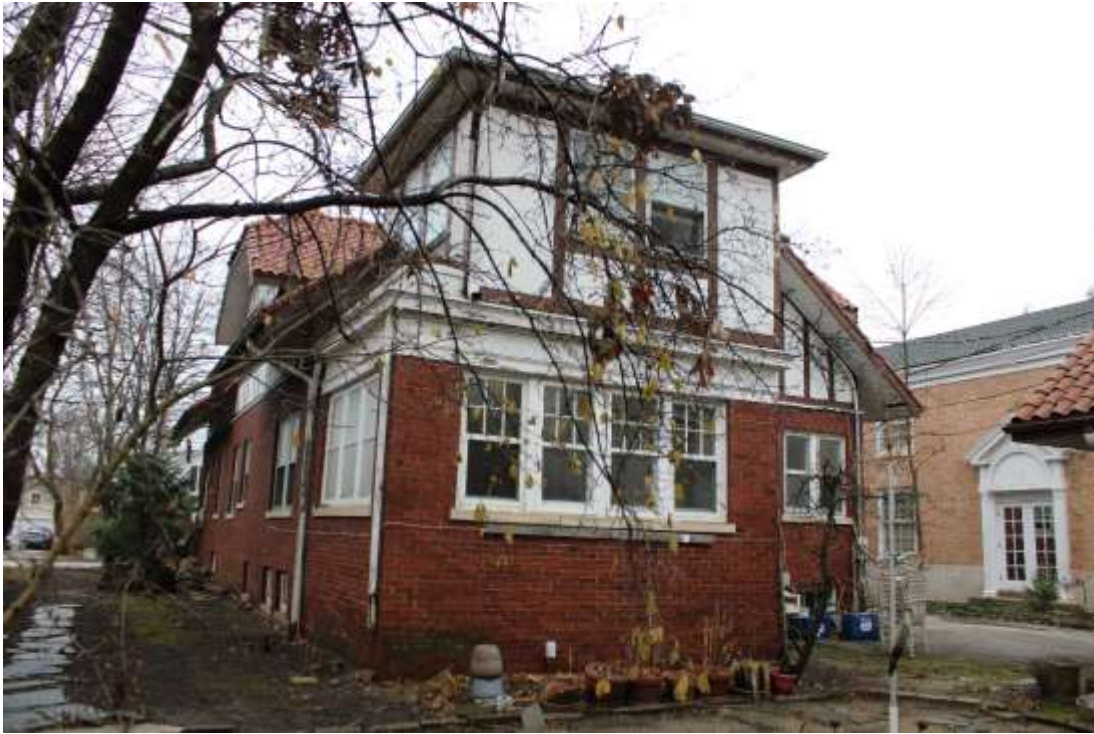
West and rear facades, view northeast.
