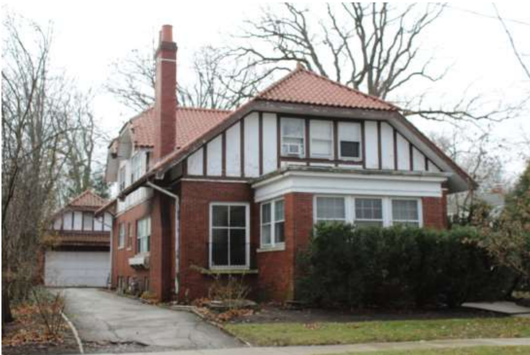
Front and east facades, view southwest.
