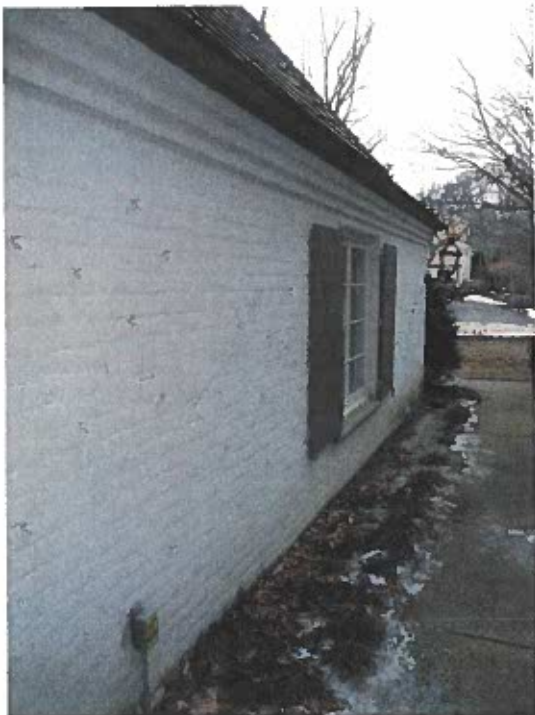
North Side of House, North Wall of Garage
