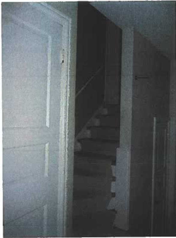
Back Staircase to Bedroom over Garage
