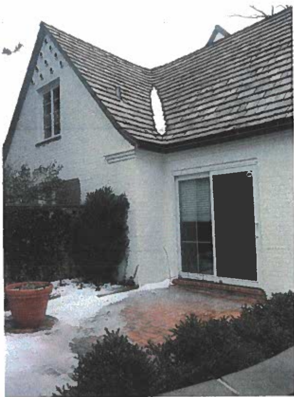
West End, South (Side) Facade. Doors from Master Suite to Side Terrace
