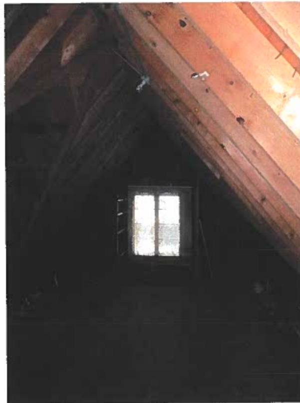
Attic over Master Suite, Office
