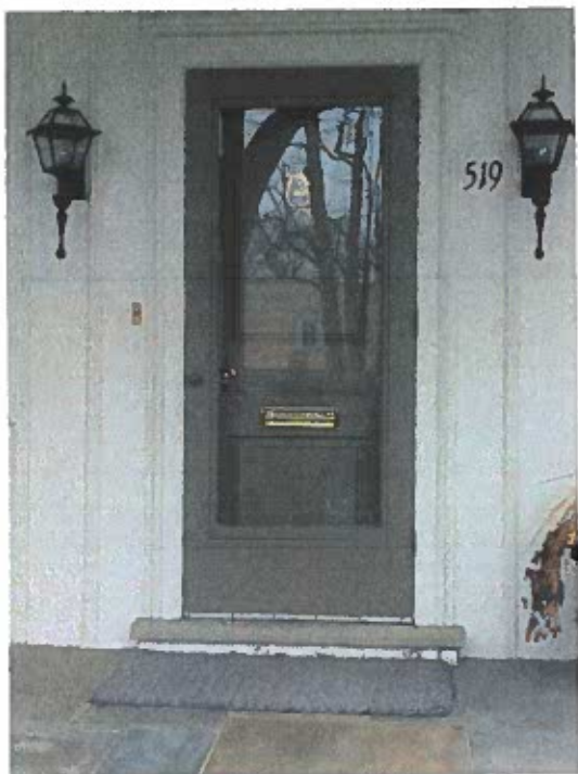
Entrance, West (Front) Facade
