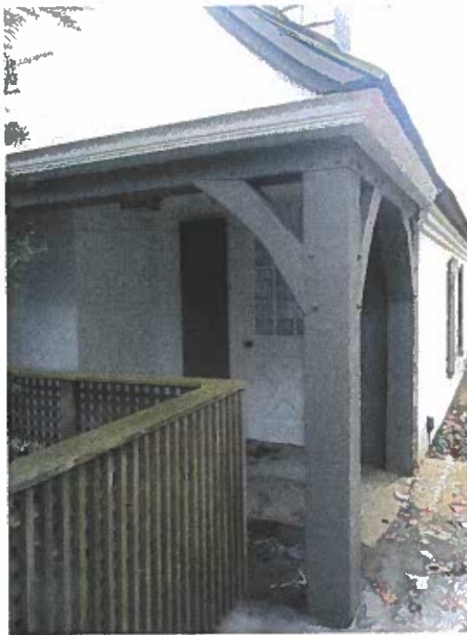
Side Porch, North Side of House, Door to Garage
