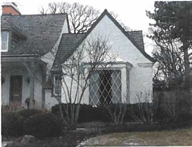
South End, West (Front) Facade
