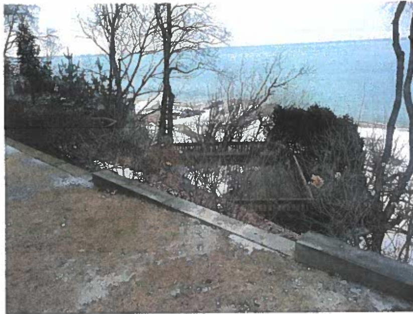
Deck Built in 1991 From Rear Yard to Beach of Lake Michigan
