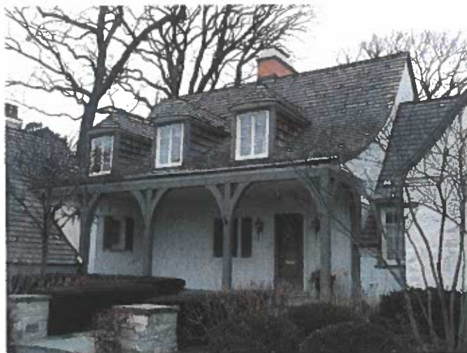
Open Porch, West (Front) Facade
