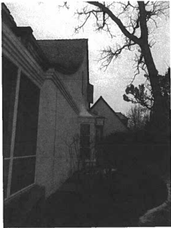
North (Side) Facade of House
