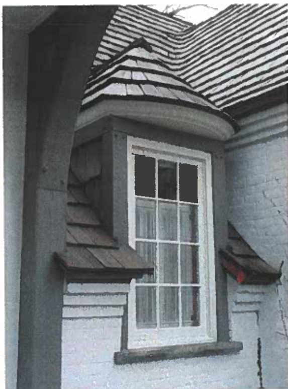
Dormer South of Entrance, West (Front) Facade
