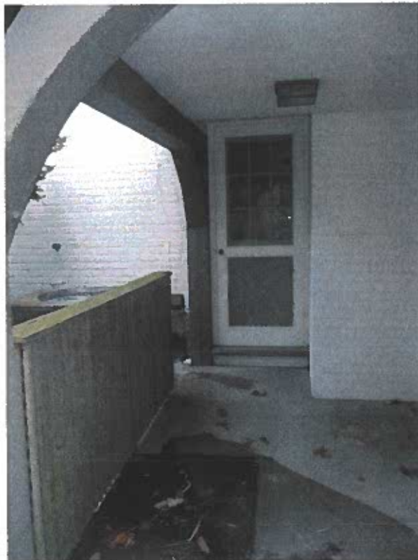
Side Porch, North Side of House, Door to House
