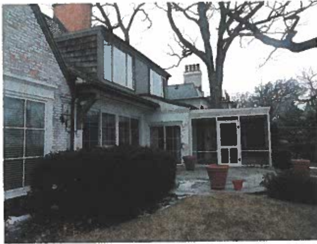
North End, East (Rear) Facade
