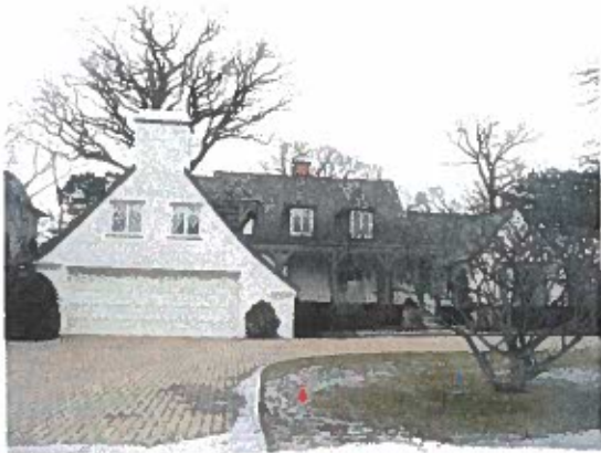
Front (West) Facade
