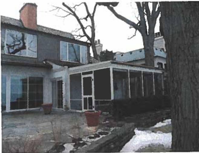
Rear Terrace and Screen Porch, East (Rear) Facade
