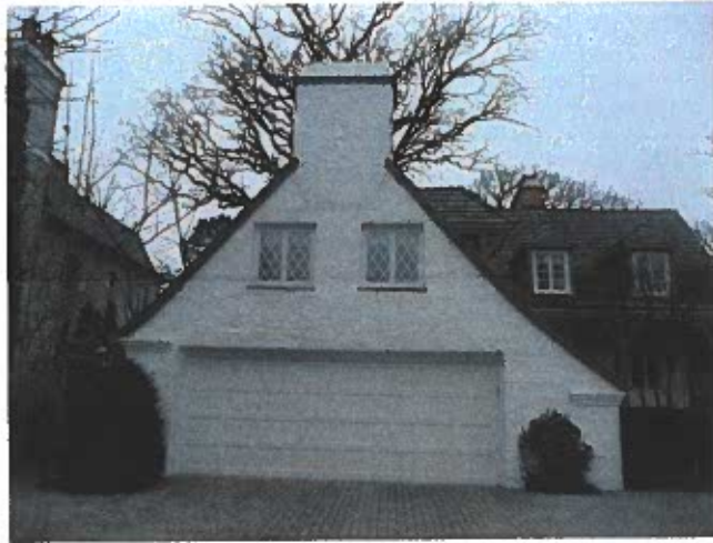
Garage, West (Front) Facade
