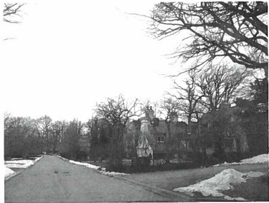
View Northeast Toward Elm Street from Mid Block
