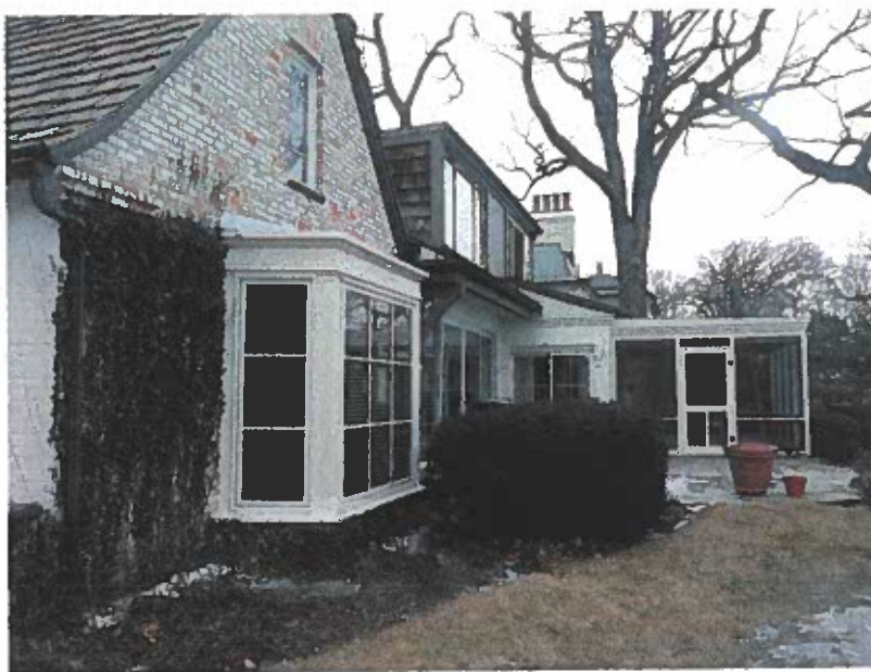
East (Rear) Facade
