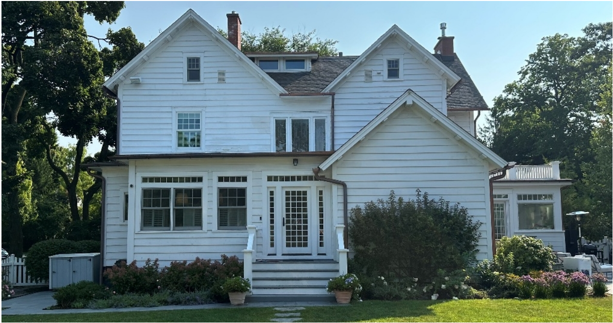
Figure 5 – Subject Property - Rear Elevation
