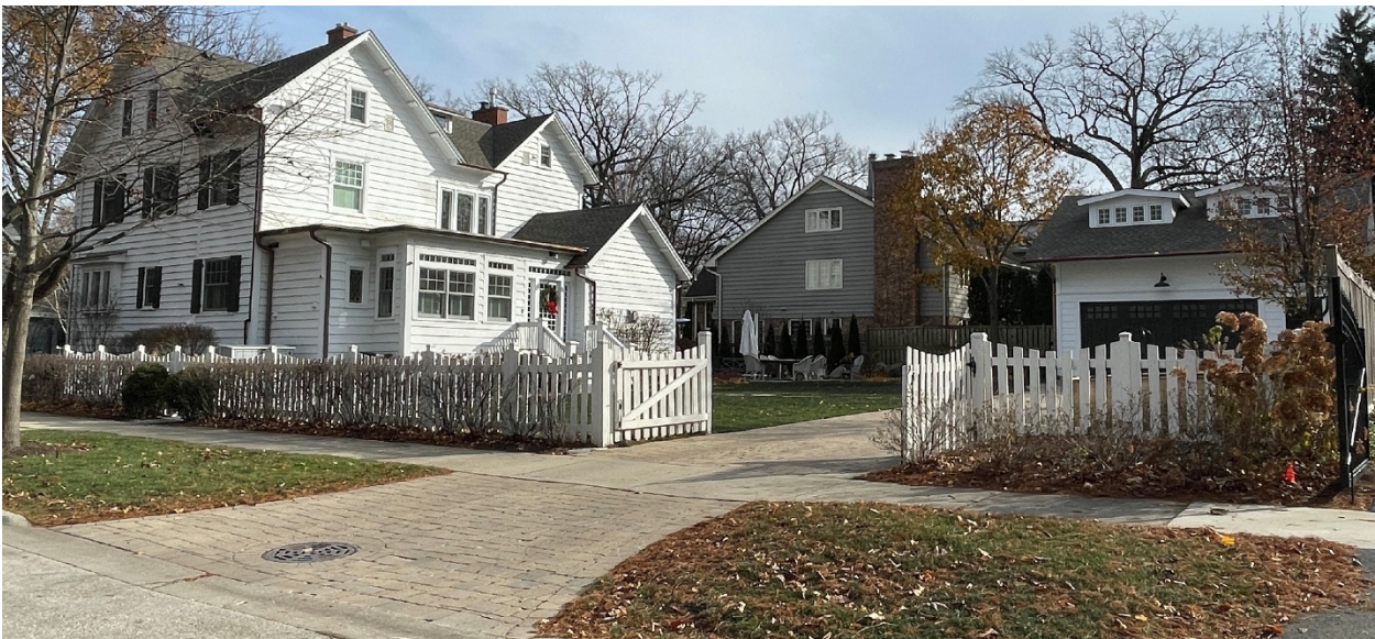
Figure 6 – Subject Property – Corner and Rear Elevations Along Summit Street
