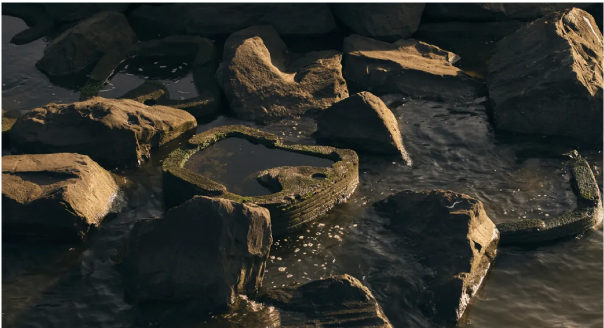
An artificial tidepool is cast into blocks of ECOCrete. Photo: SCAPE/Ty Cole
