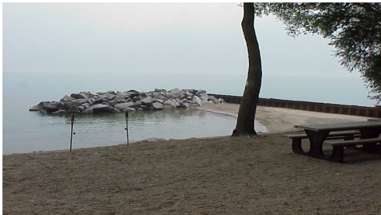
Figure 9 - Steel and stone groin
