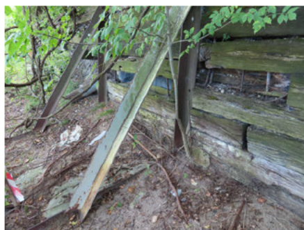
Bluff Toe Erosion and Damaged Retaining Walls
