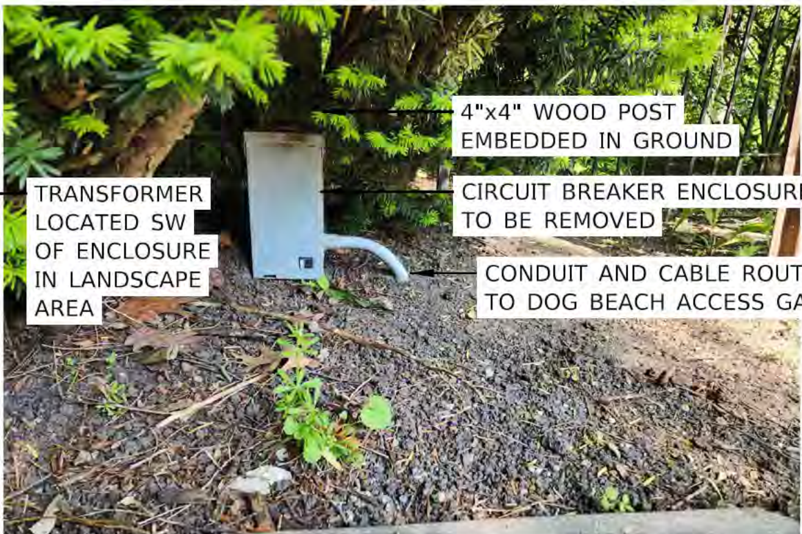
EXISTING ELECTRIC SERVICE (FOR REFERENCE ONLY) N.T.S.
