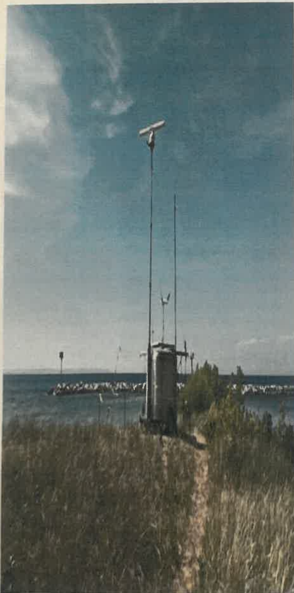
An Integrated Radar Monitoring System (IRaMS). Army Corps
