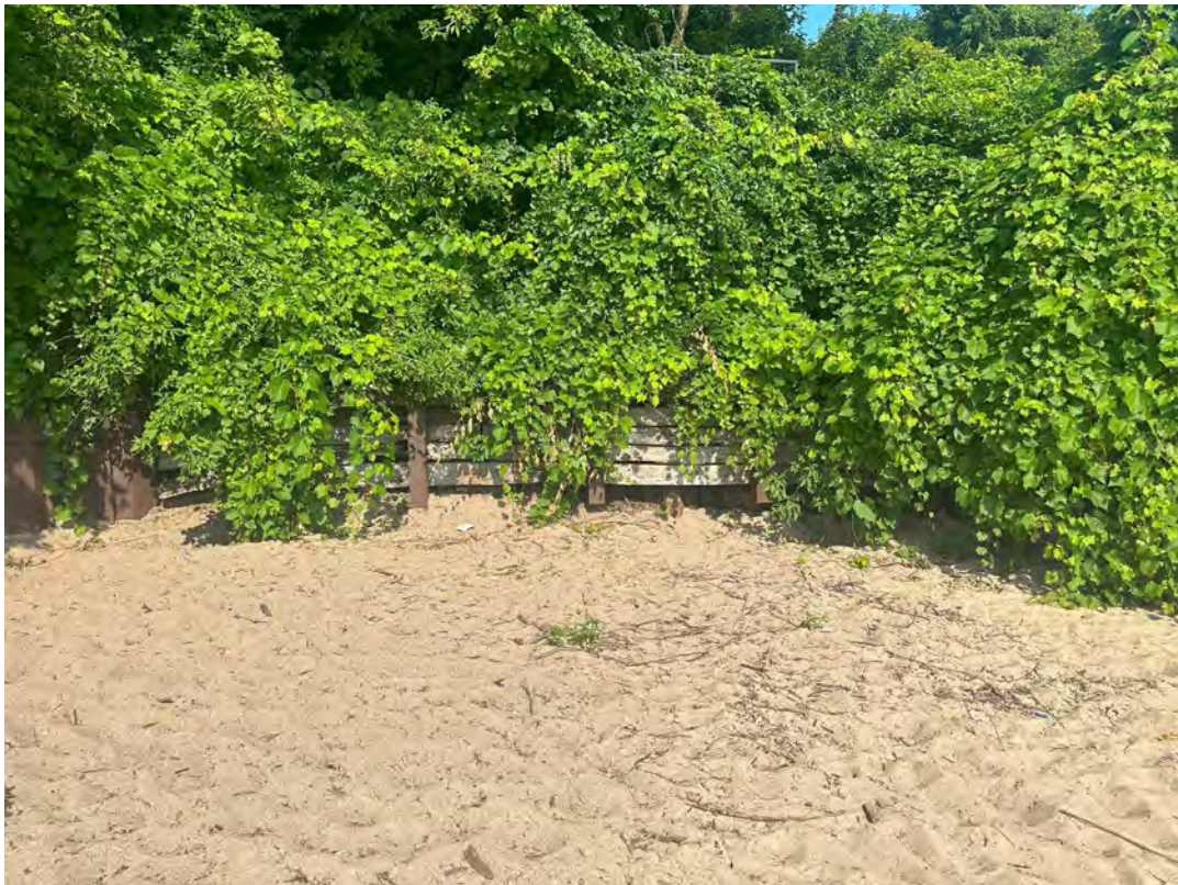
North Seawall (Looking Northwest)
