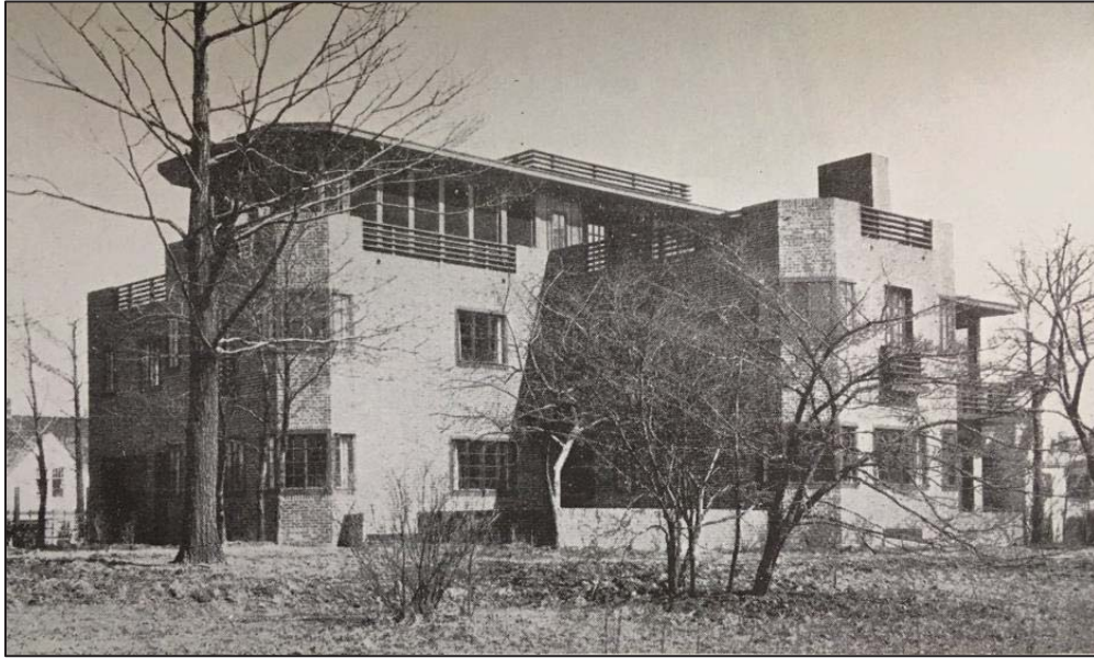
View looking northeast, with front entry at inside corner. Horn & Hound , 1929.
