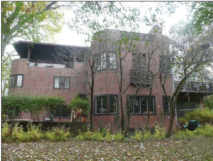
Side (South) façade (Fall, 2018)
