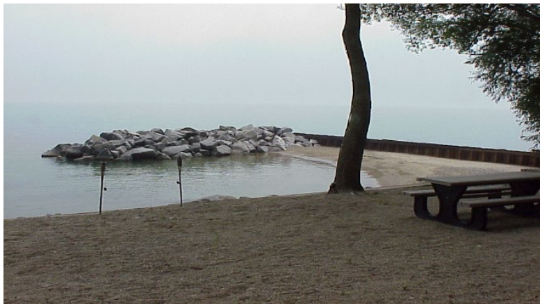
Figure 10 - Steel and Stone Groin
