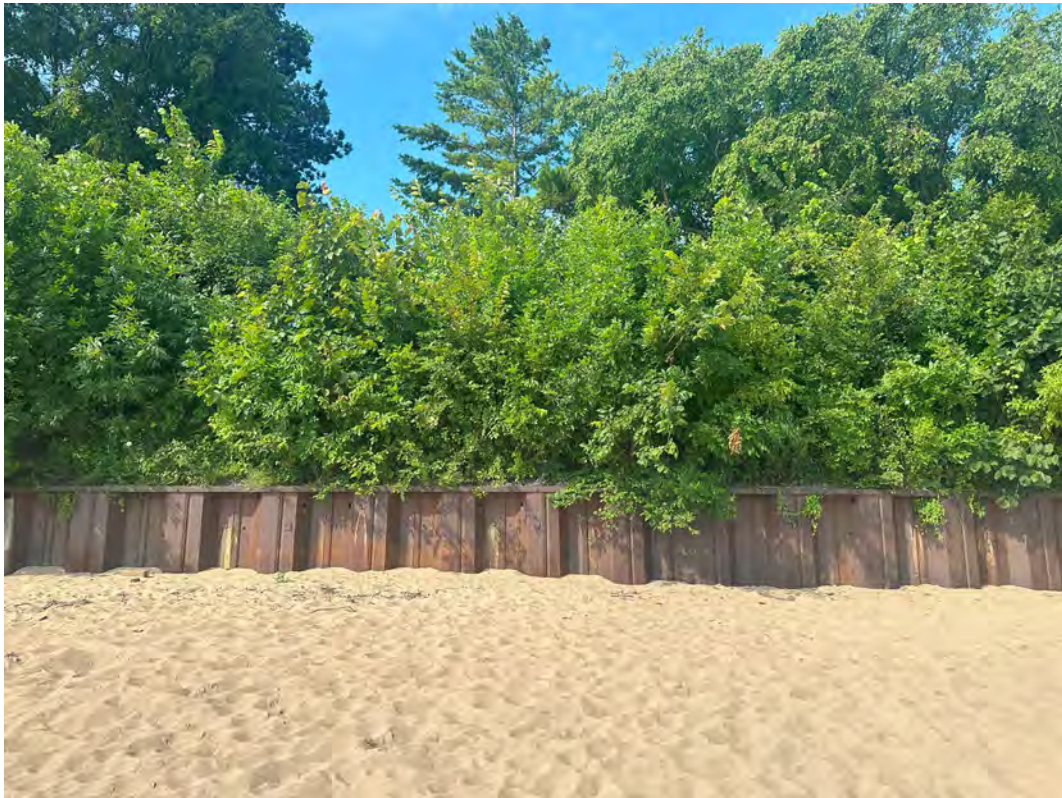
Dog Beach Seawall (Looking West)
