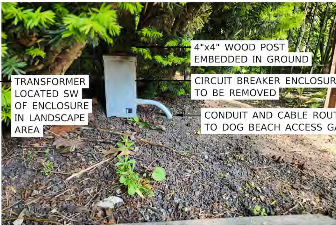
EXISTING ELECTRIC SERVICE (FOR REFERENCE ONLY) N.T.S.
