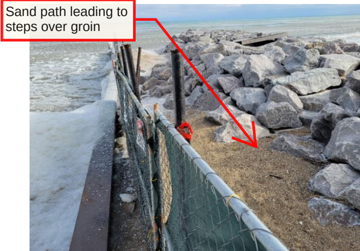
Accreted sand between steel & stone groin, Feb-9-2025
