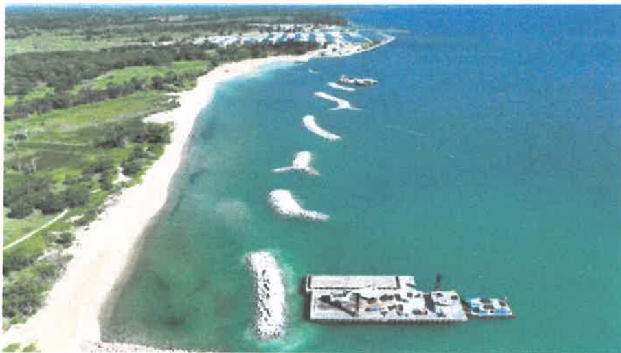
View of breakwater construction via Michels Construction
