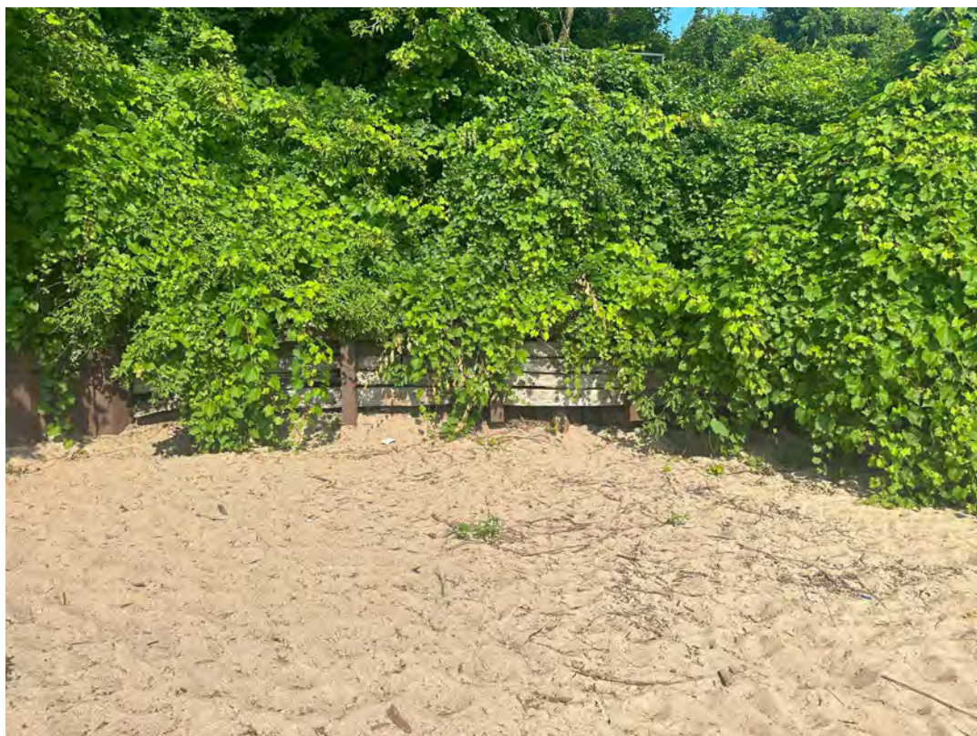
North Seawall (Looking Northwest)
