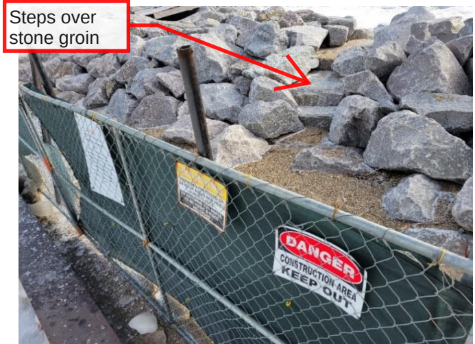
Steps over stone groin at 205 Sheridan, Feb-9-2025
