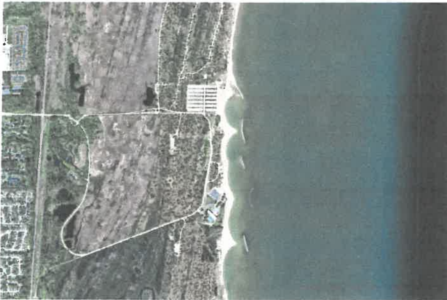
View of completed portion of shoreline reconstruction via Google Maps
