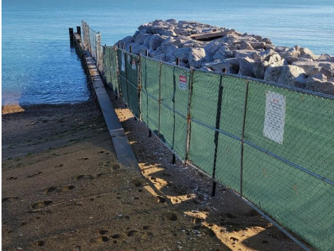
Sand level at Centennial South Groin, Oct-17-2024
