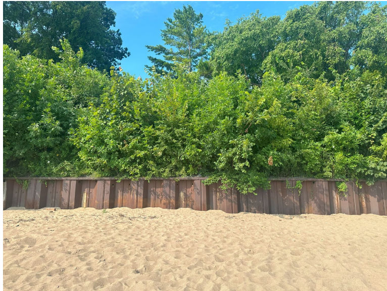
Figure 12 - Existing Sea Wall on Subject Property
