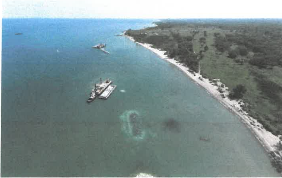
View of beach during construction via Google Maps
