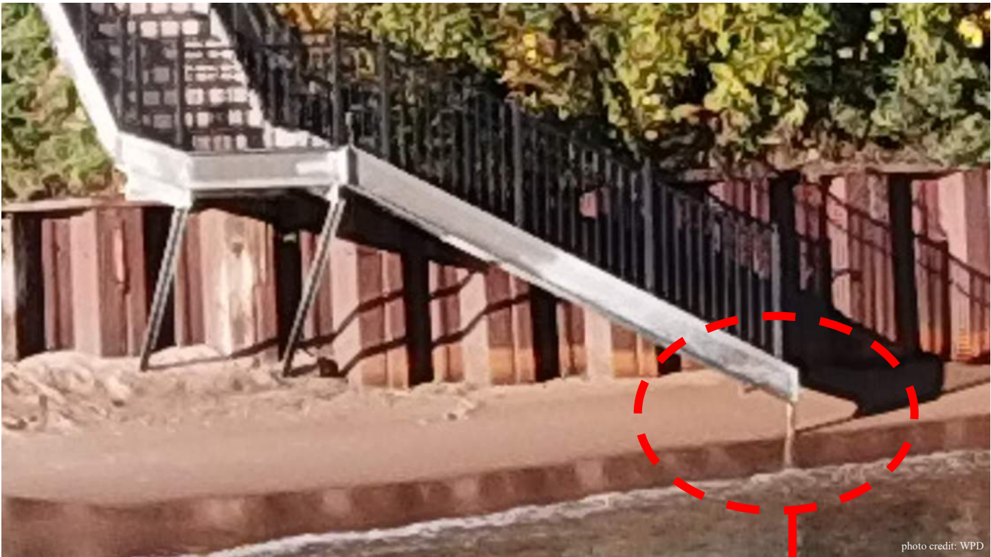
Beach erosion in 2020 meant stairs ended 24” above the beach level
