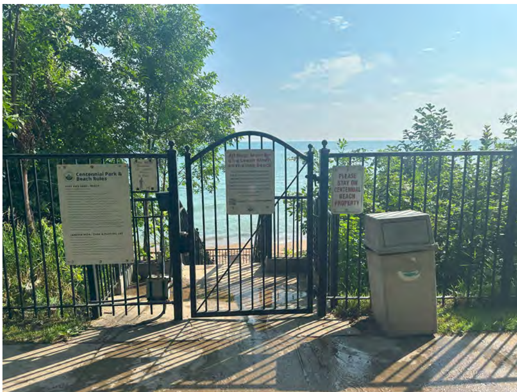
Dog Beach Access Gate (Looking East)
