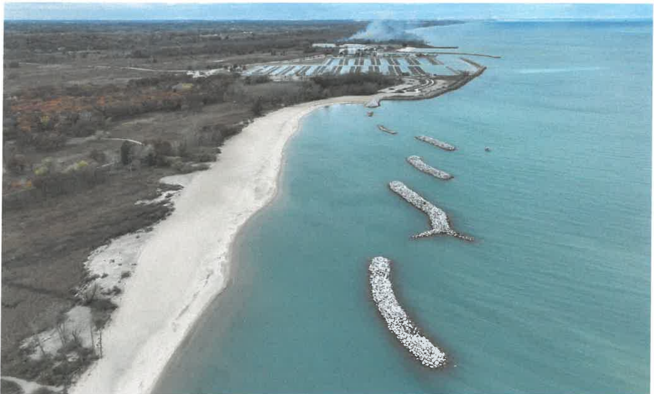
Beach and Breakwater Overview. Photo credit: Michels Construction, Inc.
