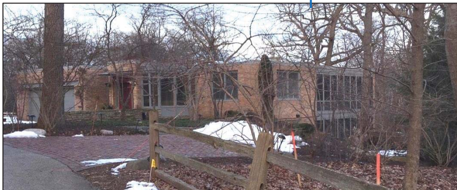
Howard Fisher House, view northeast, photographed February, 2019
