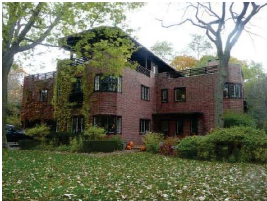
Front (West) Façade (Fall, 2018)
