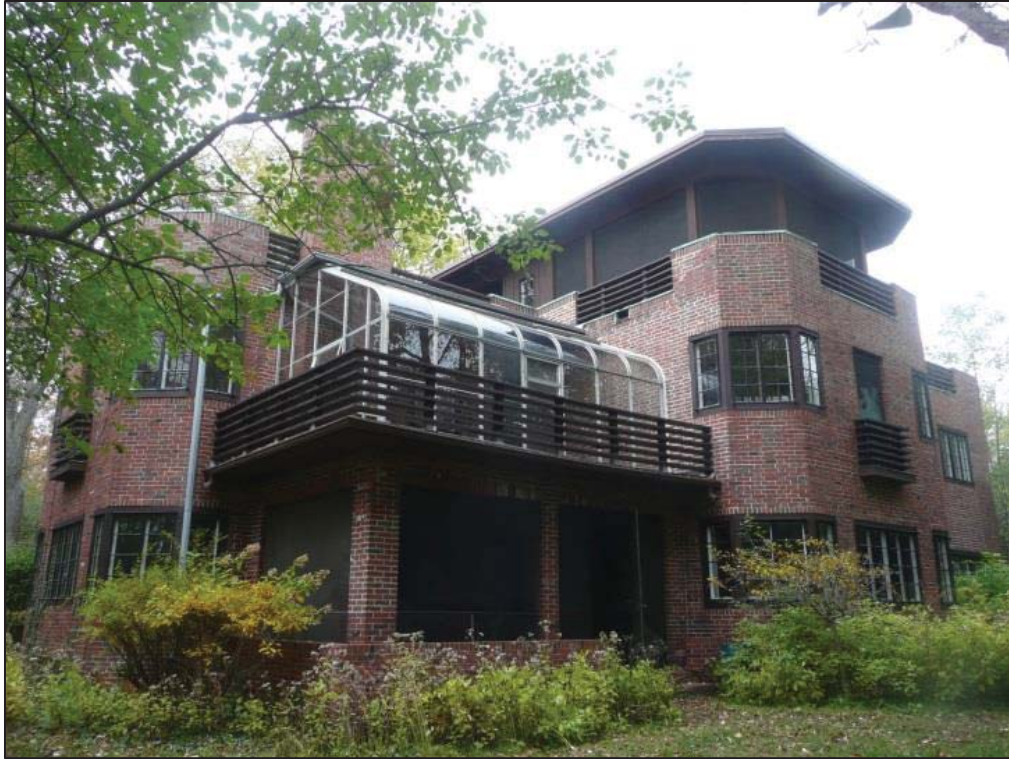
Rear (East) façade (Fall, 2018)
