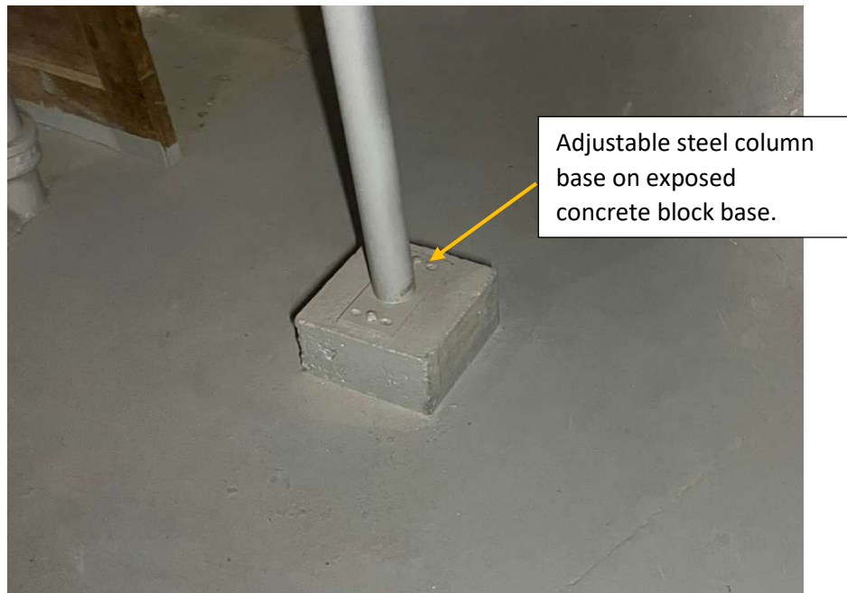
Picture 17: Adjustable Steel Column Base.
