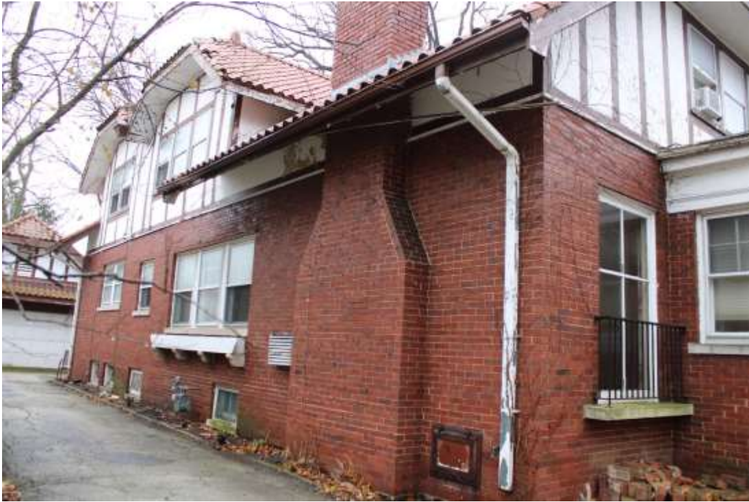
East façade, view southwest.
