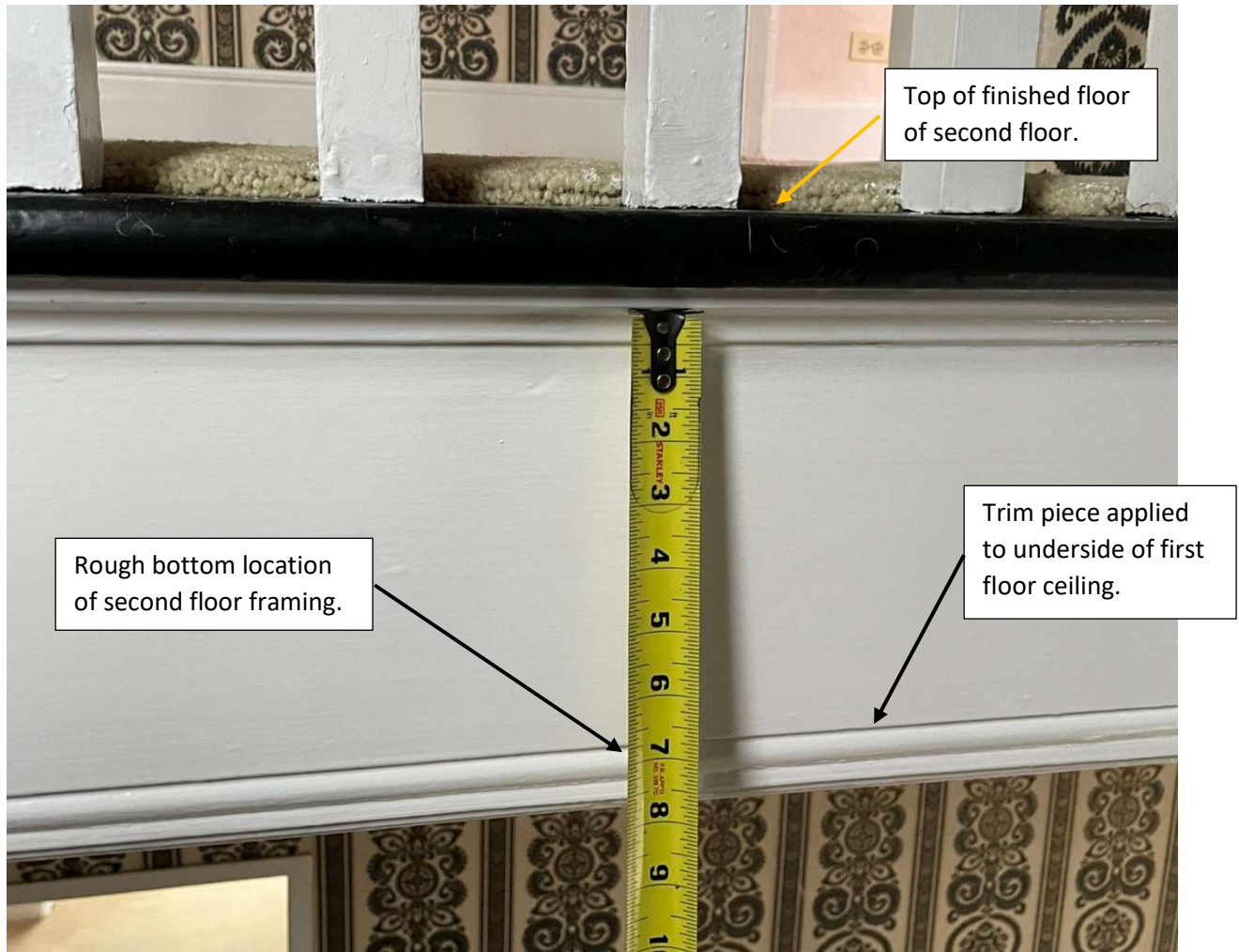
Picture 8: Rough Second Floor Framing Thickness Measurement.
