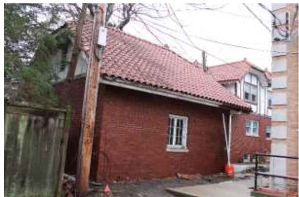
East façade of garage, view northwest.
