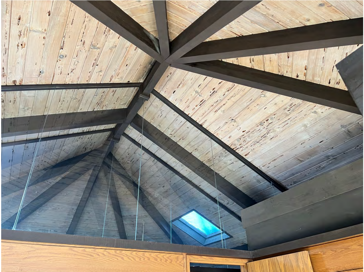
West wing ceiling over kitchen and servant's bedroom, looking northeast from servant's bedroom
