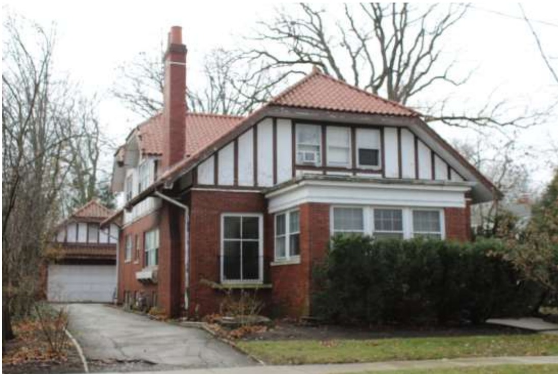
Front and east facades, view southwest.
