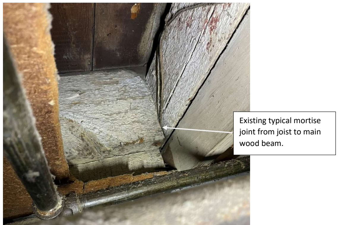
Picture 14: Mortise Joist to Main Wood Beam.
