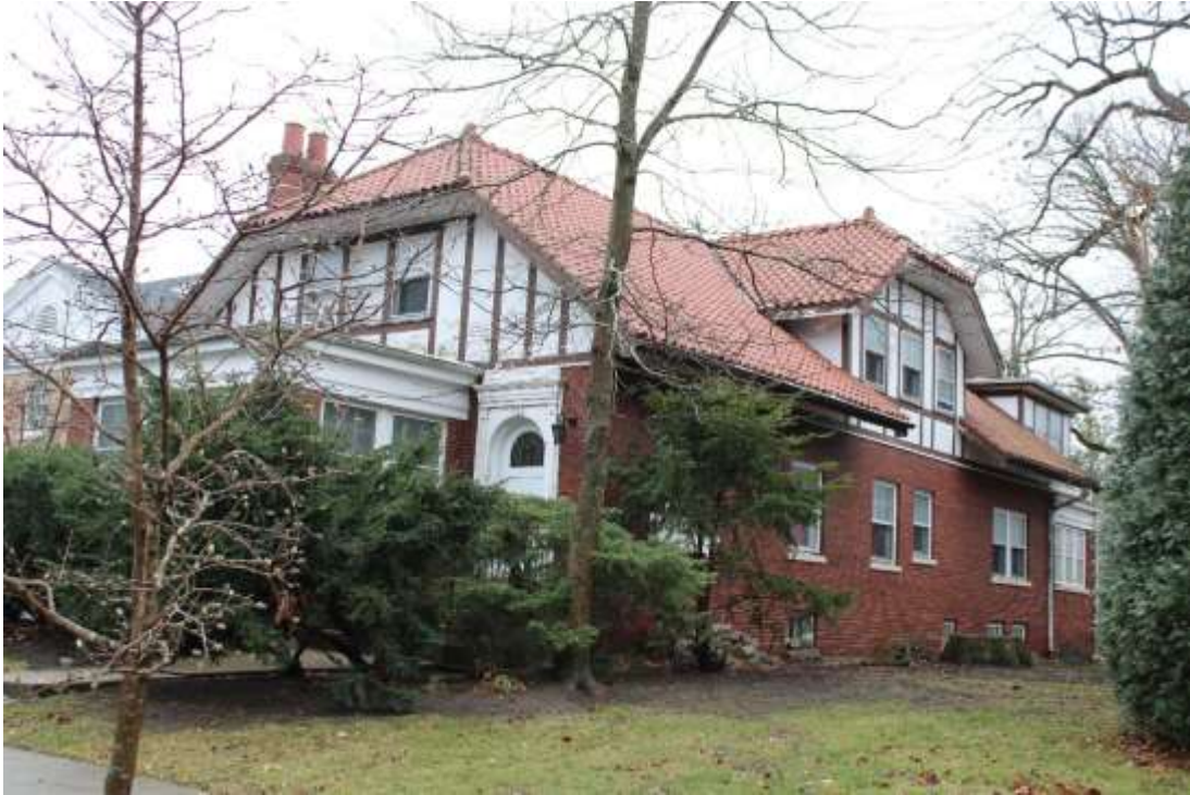
Front and west facades, view southeast.
