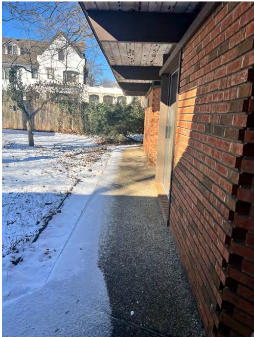
West façade of north wing, looking north
