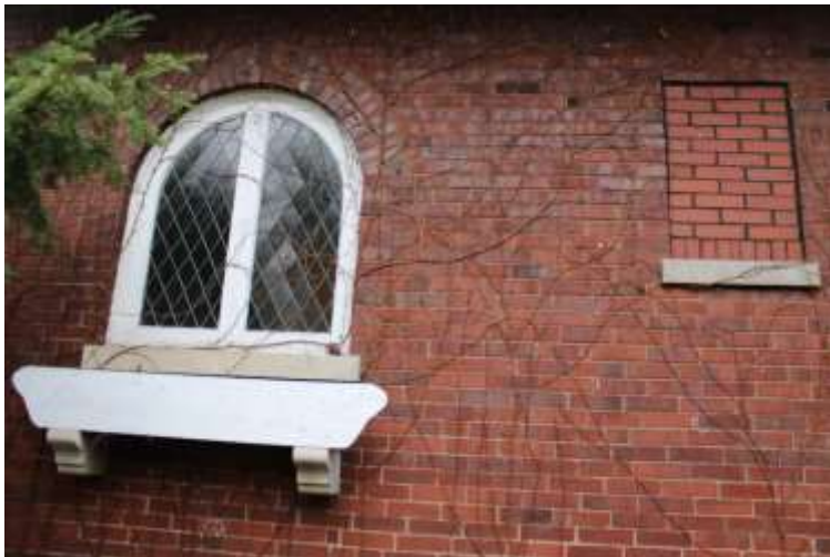
West façade detail.
