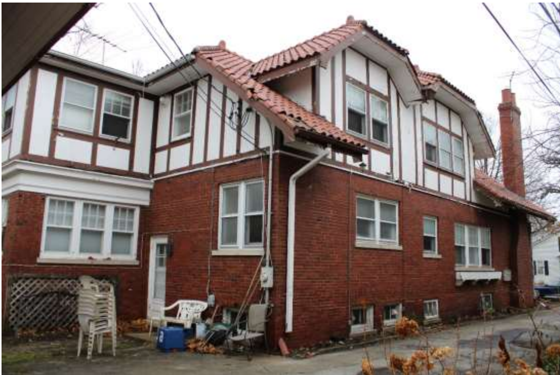
East and rear facades, view northwest.
