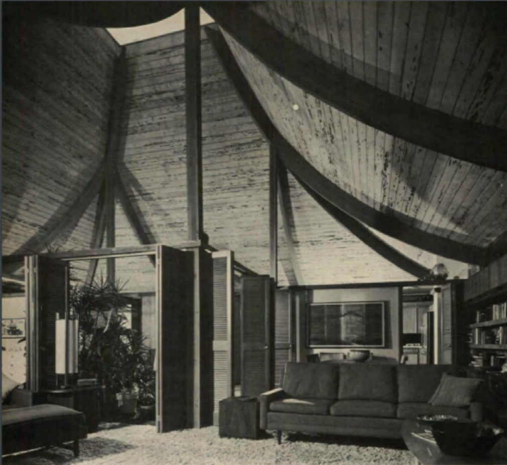
VAULTED ROOF over main living area (view E in plan) is framed with curved glue-lam beams, planked with pecky cedar. Skylight is 25' above floor.
