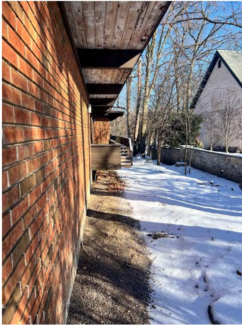
South façade, looking east
