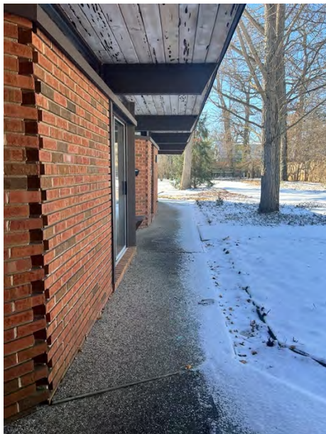
North façade of west wing, looking west
