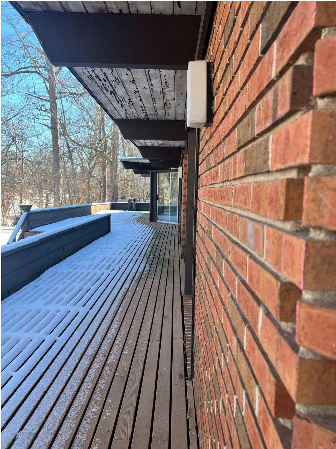
East façade and deck, looking south
