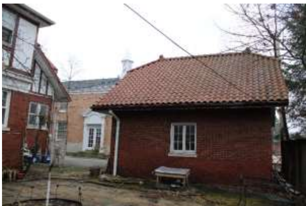
West façade of garage, view east.
