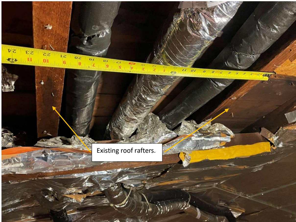
Picture 1: Existing Roof Framing
