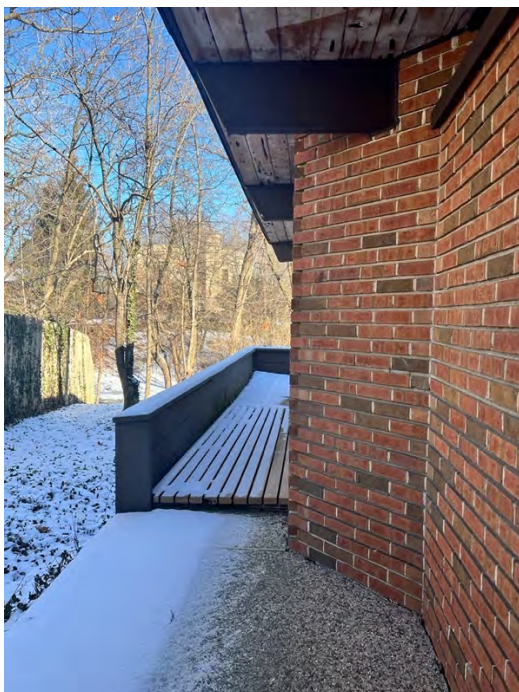
North façade of north wing, looking east to deck
