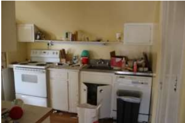
Second floor Kitchen, view southwest.
