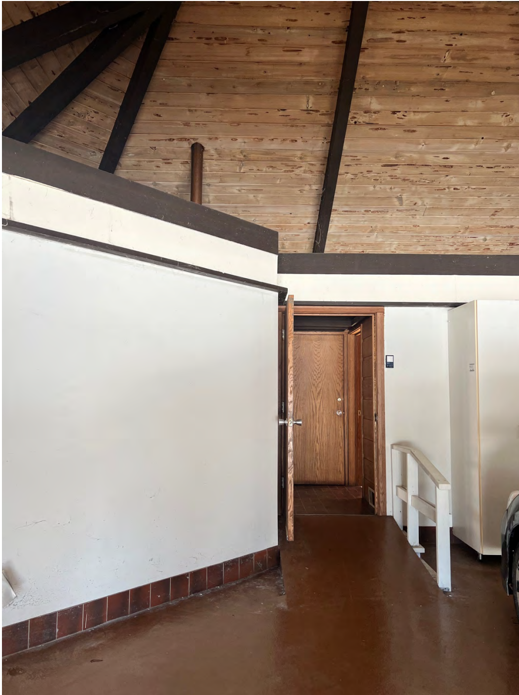
View of basement door from garage, looking east
