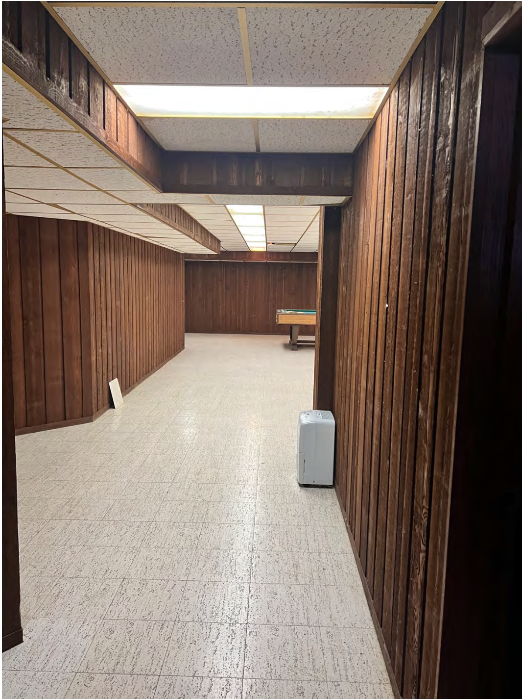
Basement, looking east
