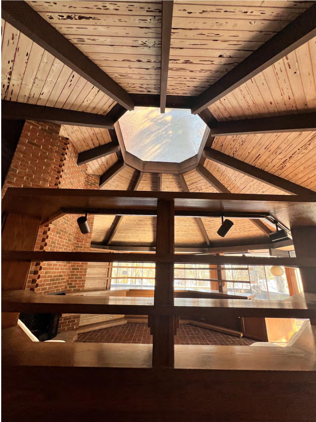
View of skylight above "cave"
