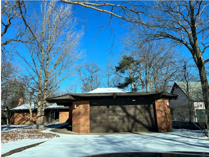
Front (west) façade, looking east
