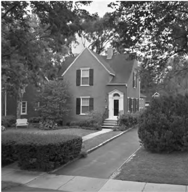
PHOTO OF ADJACENT BUILDING AT SOUTH SIDE OF PROPERTY
