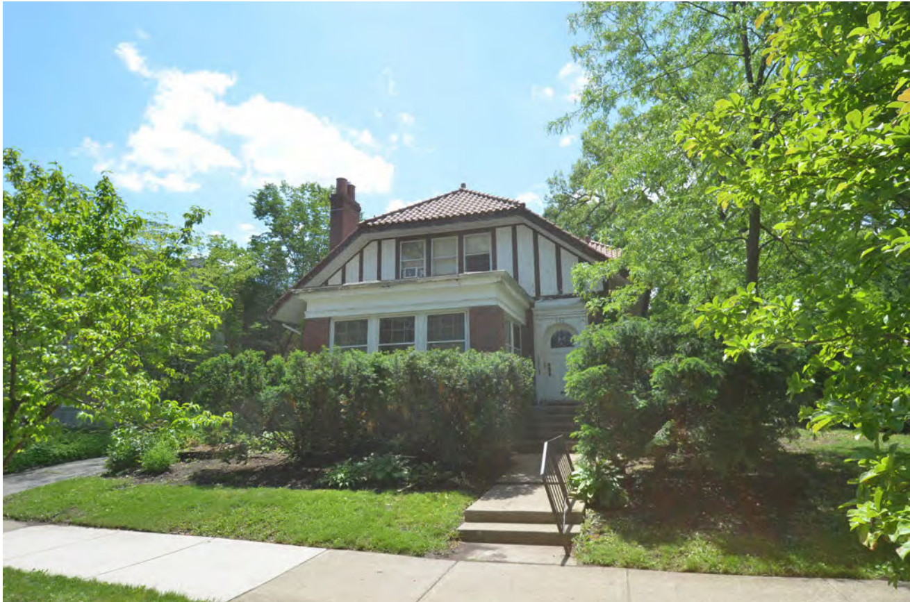
VIEW OF NORTH FACADE
