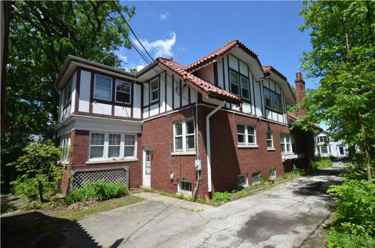
VIEW OF SOUTH & EAST FACADE
