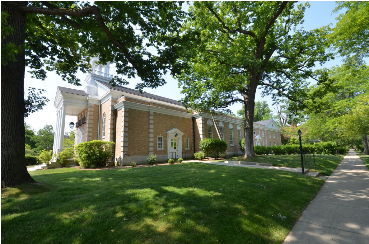
Figure 5 – Grace Presbyterian Church – North Façade
