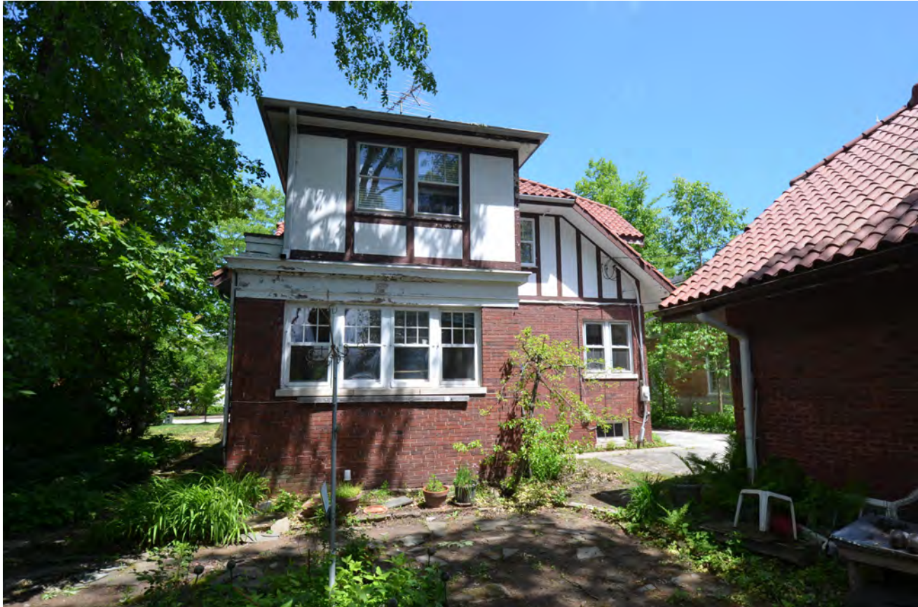
VIEW OF SOUTH FACADE
