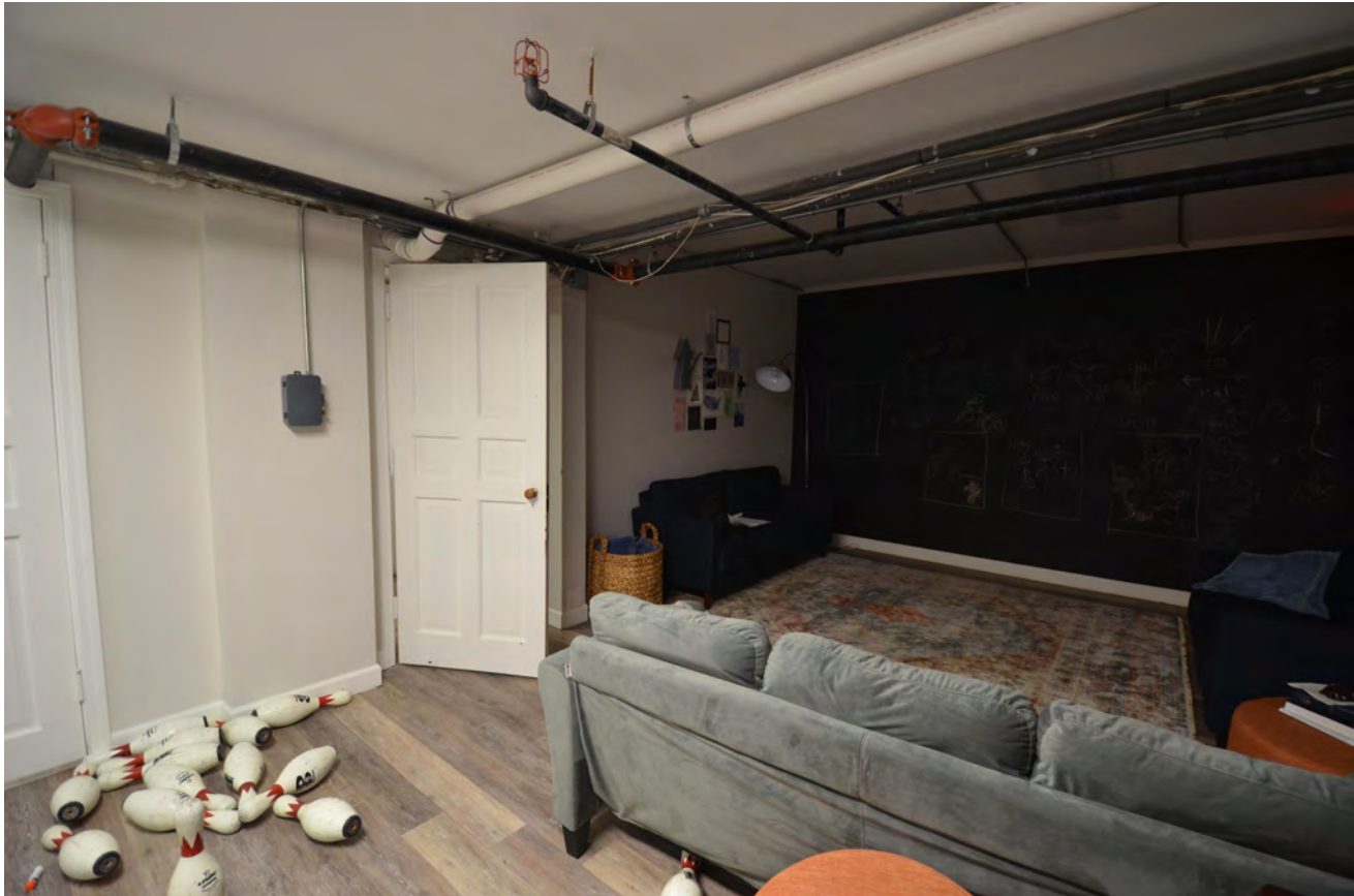
LIMITED HEADROOM IN EXISTING BASEMENT
