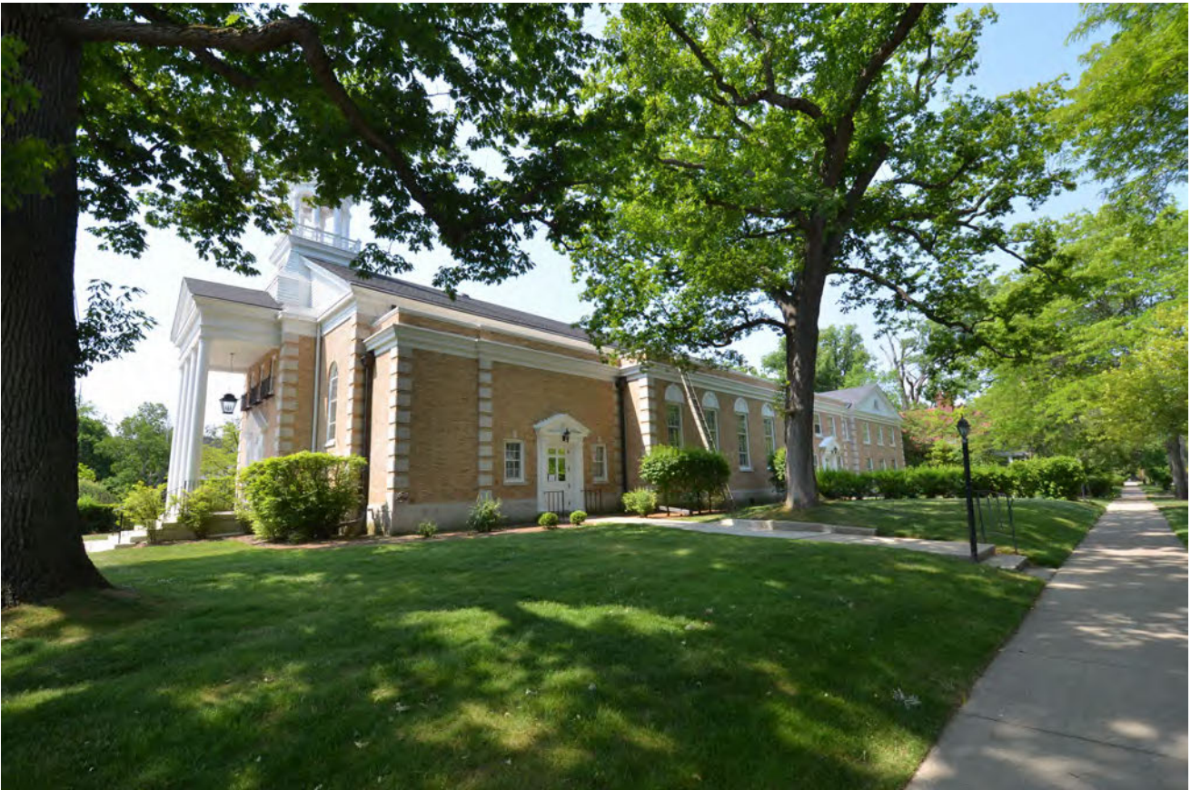
VIEW OF NORTH FACADE
