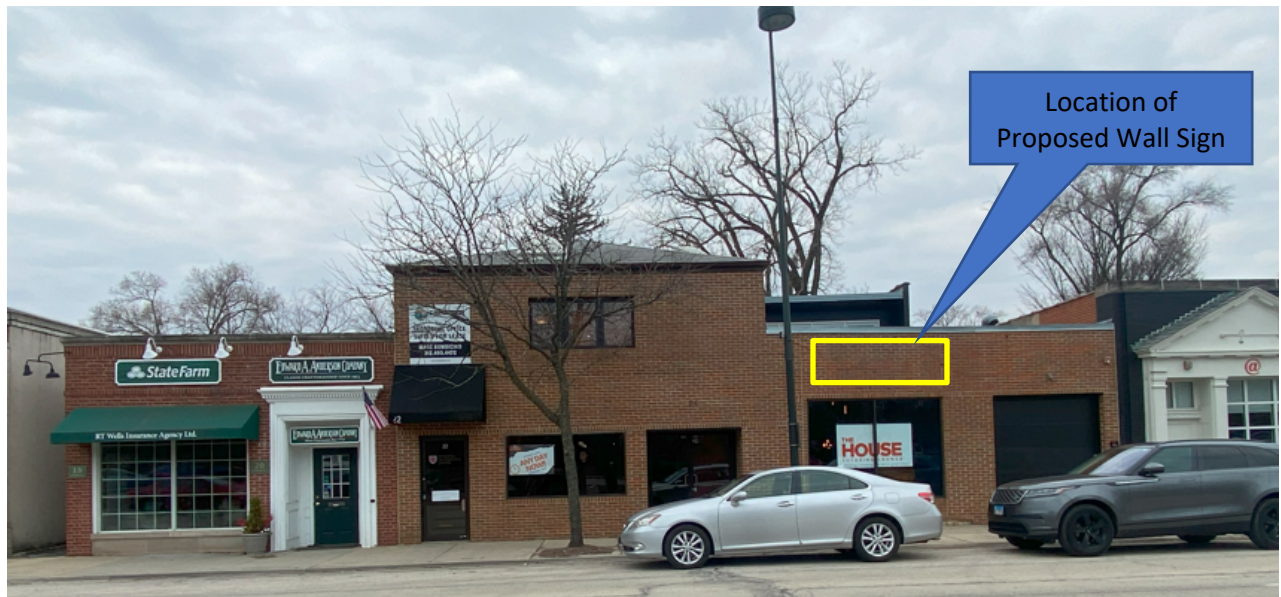
Figure 3 – Subject Property – Building View/Green Bay Road Elevation
