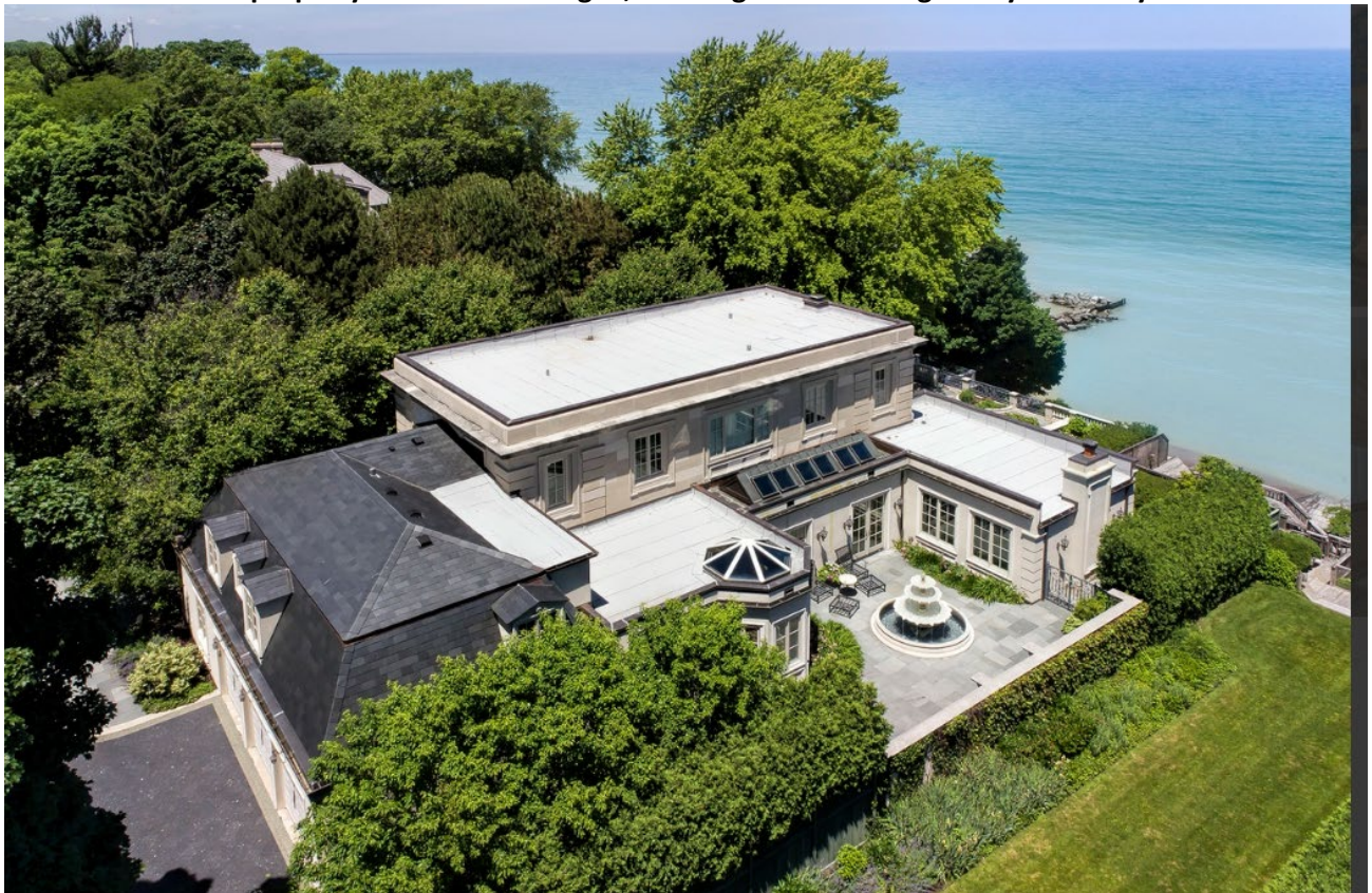
Aerial of South Façade, showing Garage addition; kitchen, atrium and family room additions
