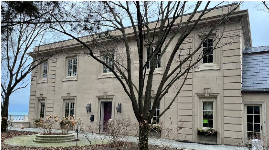
Figure 2 – Subject Property – Front Entrance of House (Northwest Elevation)
