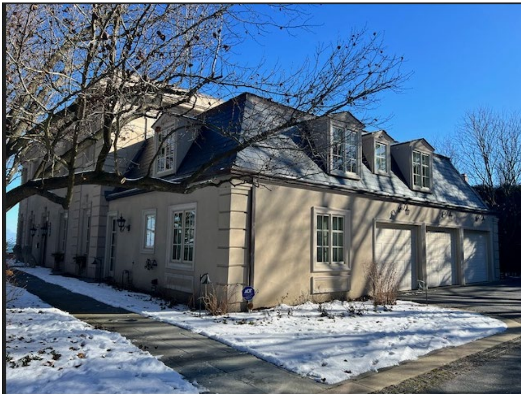
North and West facades, showing 1961 garage addition
