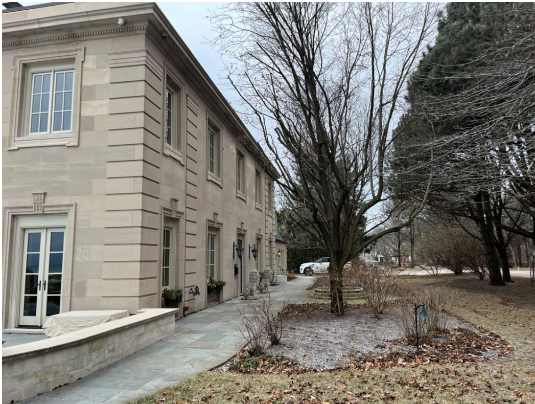
View west, past north façade of house
