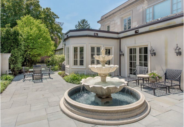
South Façade, view west toward kitchen, atrium addition
