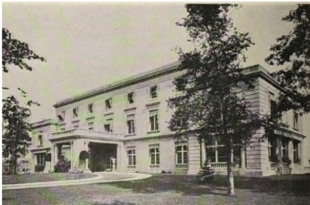
Estate House, 483 Sheridan Road, W. Façade, 1914
