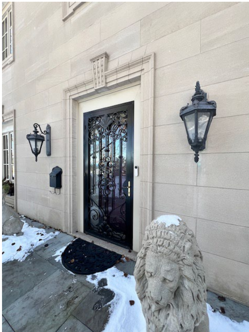
Front Entrance, North Side of House, 2025 photo
