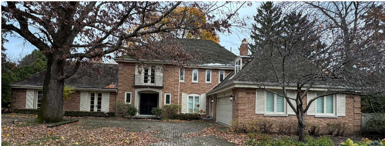
Figure 6 – 499 Sheridan Road (West Elevation)
