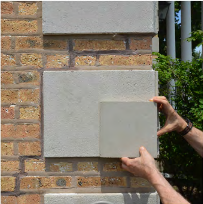
CS-1: CAST STONE TO MATCH EXISTING
