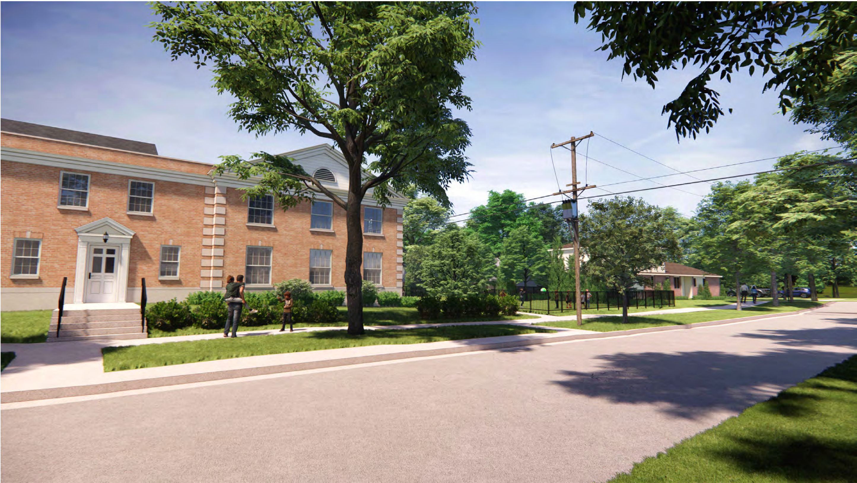
VIEW OF NORTH ADDITION FROM CHERRY STREET
