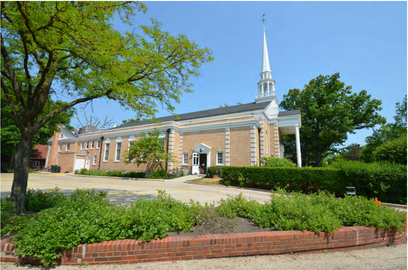
VIEW OF SOUTH FACADE
