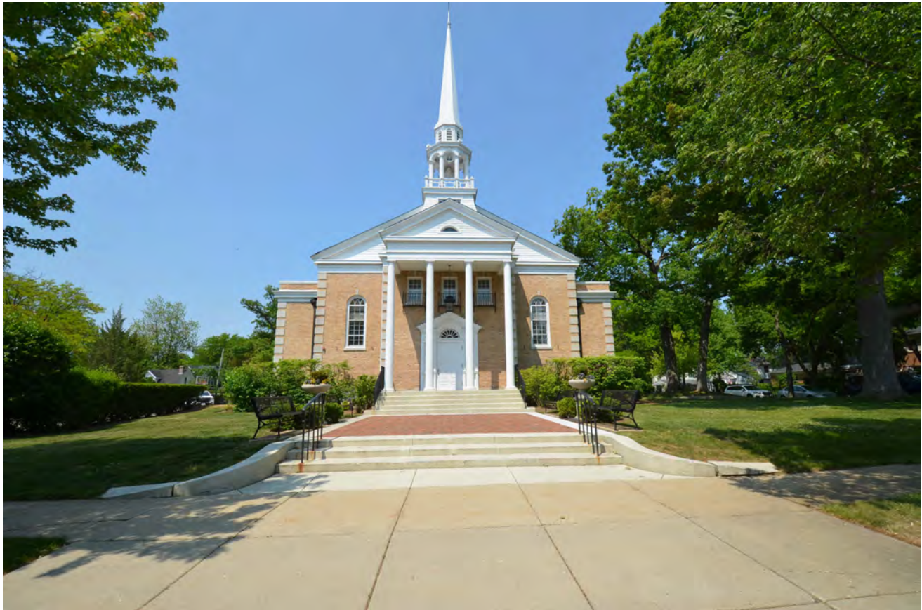
VIEW OF EAST FACADE
