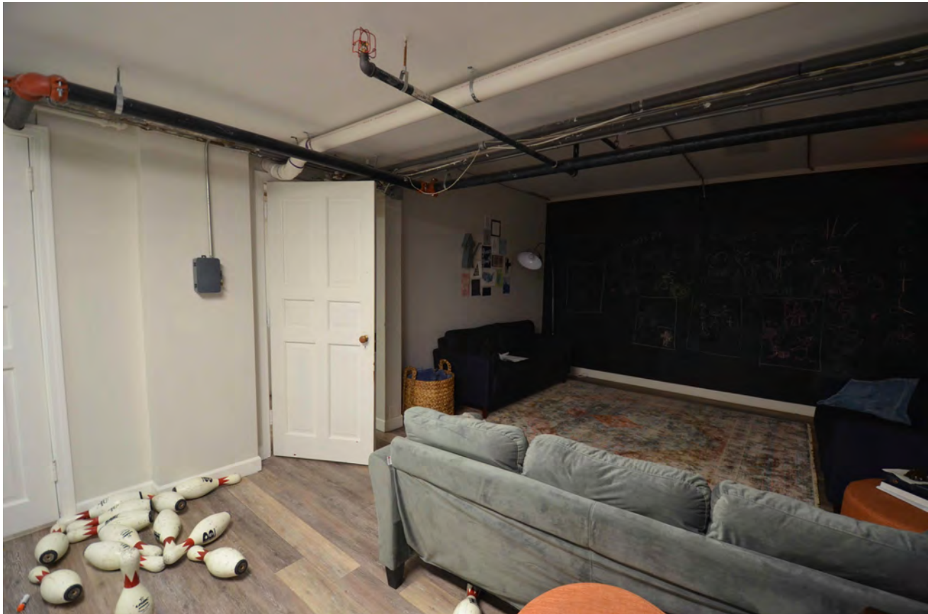
LIMITED HEADROOM IN EXISTING BASEMENT
