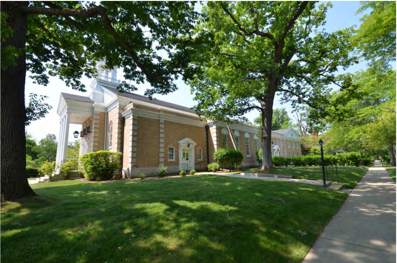
VIEW OF NORTH FACADE
