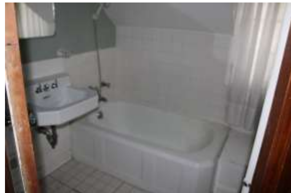
Second floor bathroom.
