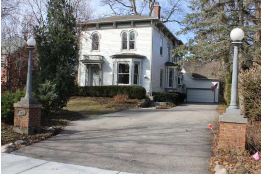
Front façade, view southwest.
