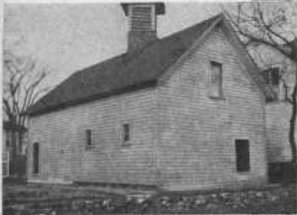
BEFORE The barn before remodeling was a plain rectangular box with a rakish cupola set atop it like a boy's cap on the back of his head
