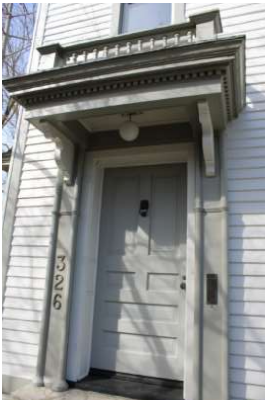
Front façade entrance.
