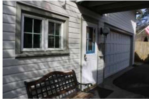
Front façade detail, view northwest.
