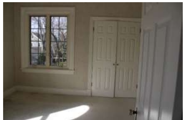
Bedroom 2 at the southwest corner of the house.
