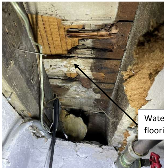
Pictures 11 & 12: Existing First Floor Joist Depth & Water Damaged Sub-floor.
