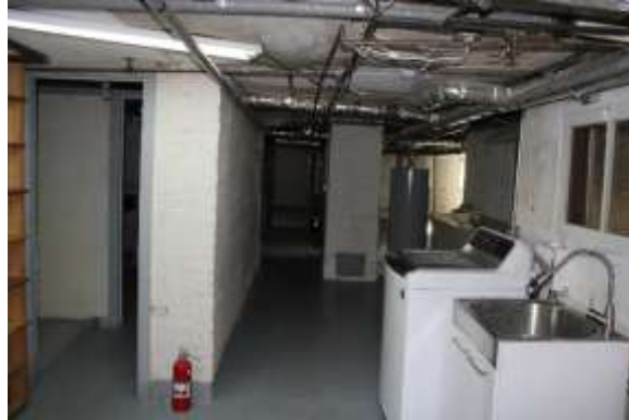
Views of basement.
