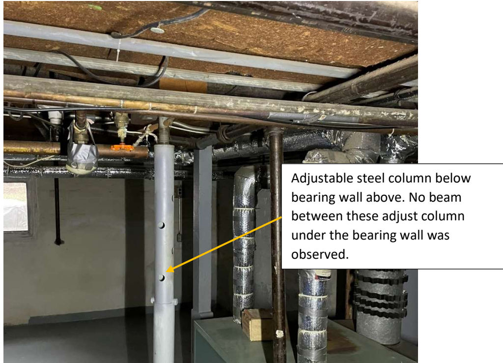
Picture 15: West Temporary Adjustable Column.
