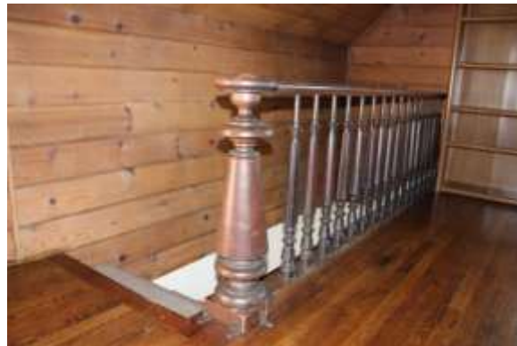
Second floor balustrade.
