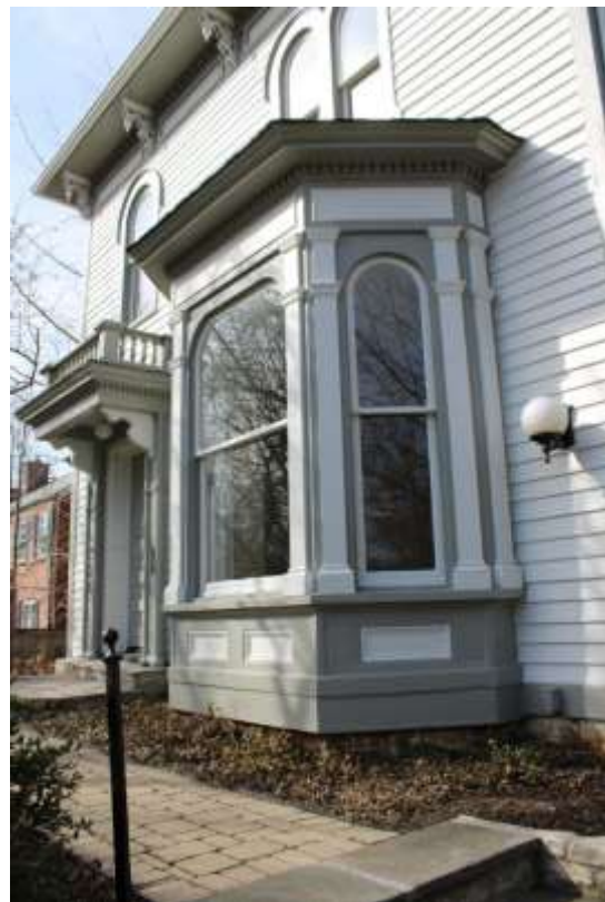
Front façade window bay.
