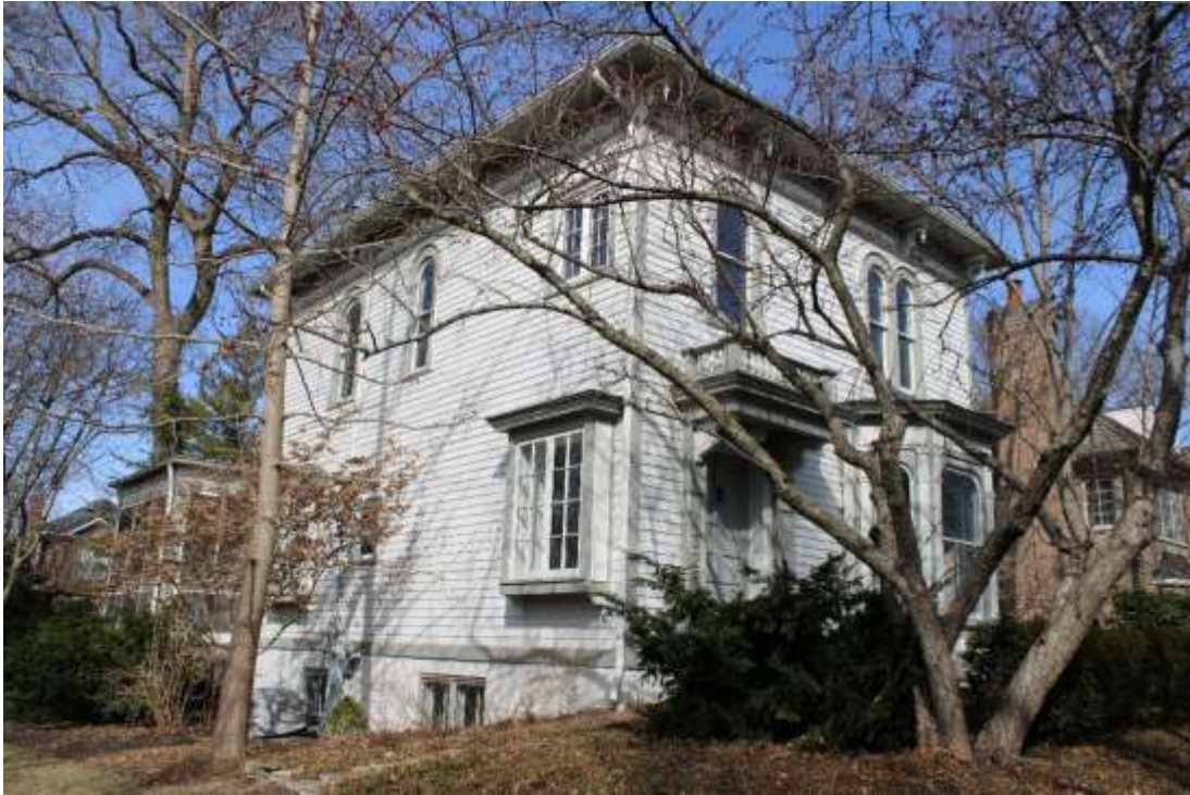
Front and south facades, view northwest.
