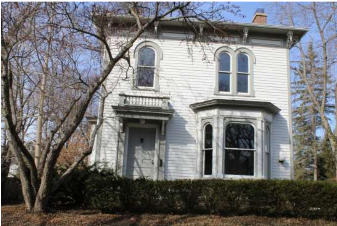
Front façade, view west.
