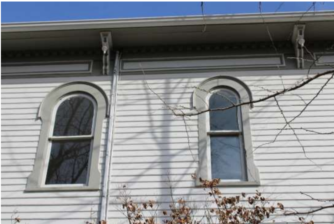
Original round arch windows and decorative brackets on south façade.
