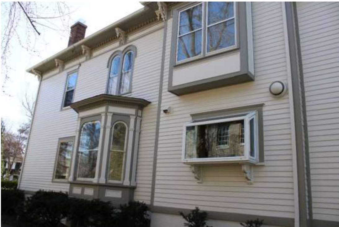
North façade, view southeast.
