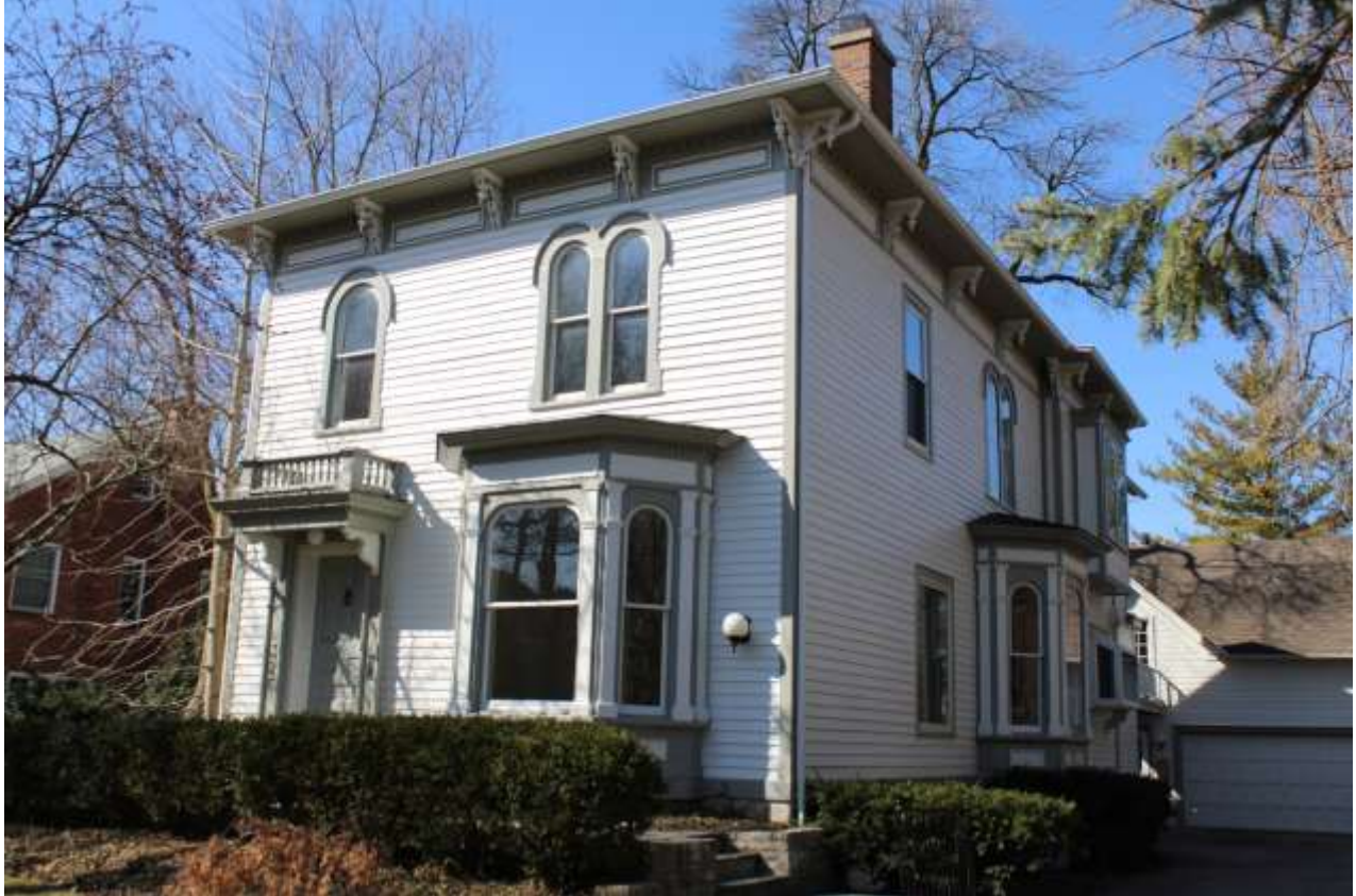
Built c. 1872 Developer: John T. Dale
