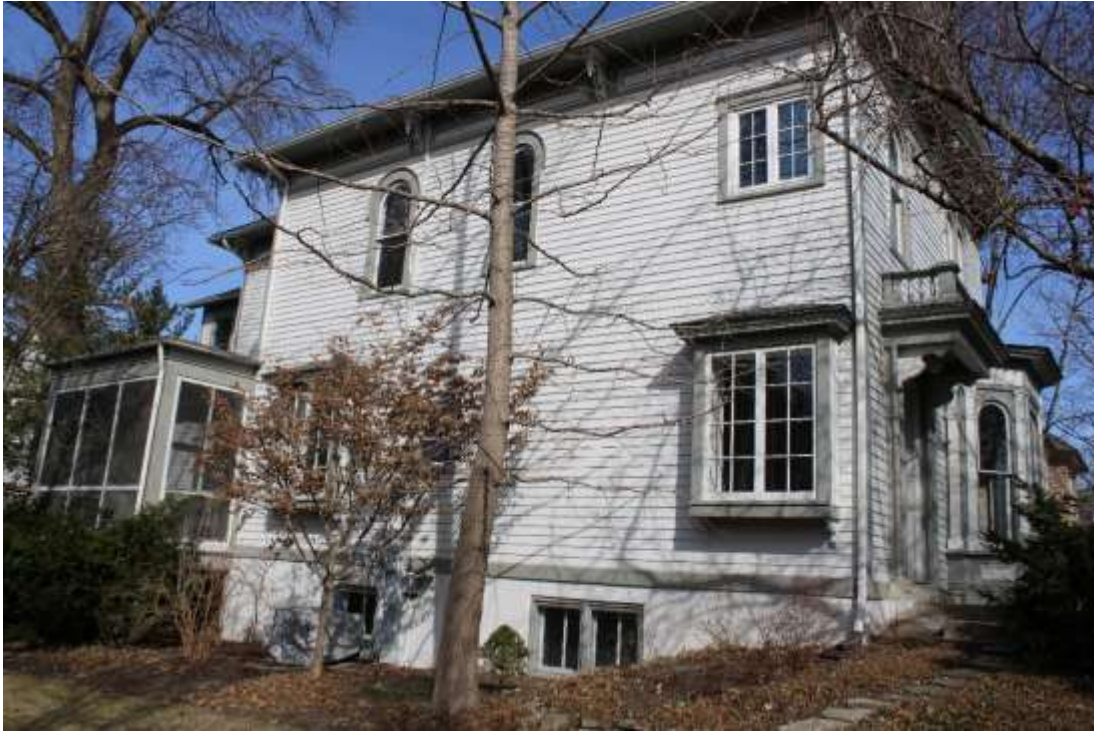
South façade, view northwest.
