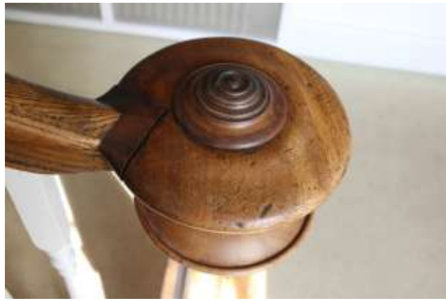
Front hallway and newell post detail.
