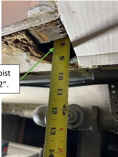
Pictures 11 & 12: Existing First Floor Joist Depth & Water Damaged Sub-floor.
