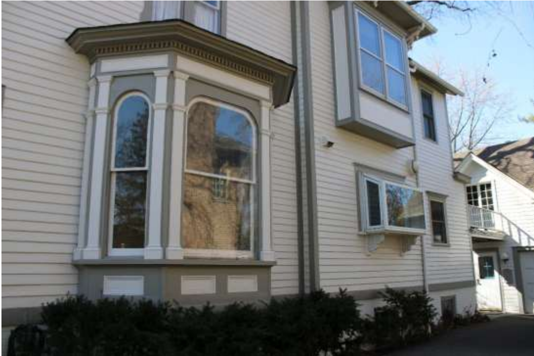
North façade, view southwest.
