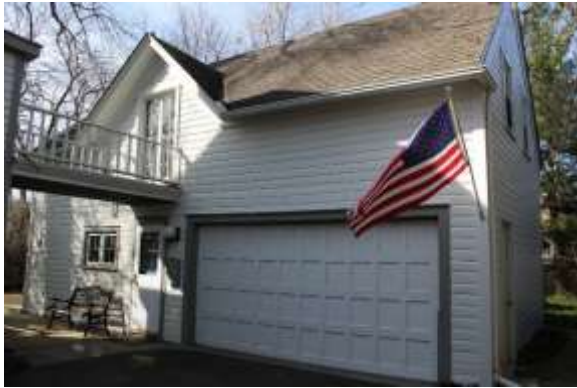
Front façade, view southwest.
