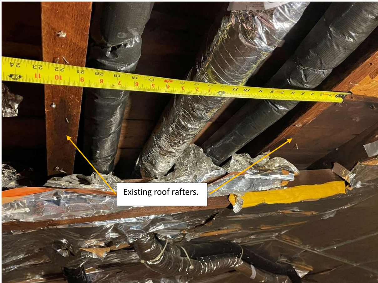
Picture 1: Existing Roof Framing
