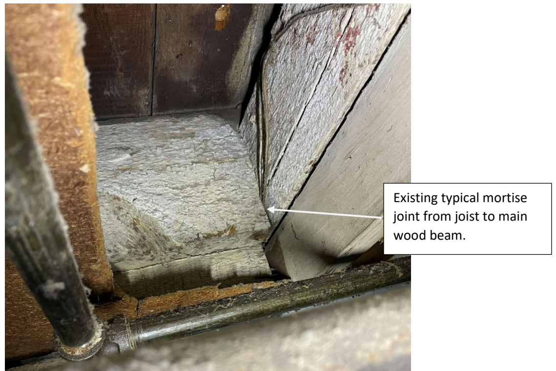
Picture 14: Mortise Joist to Main Wood Beam.
