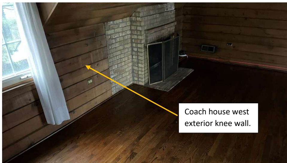
Picture 22: Coach House West Exterior Knee Wall.
