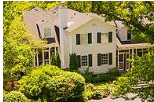
596 Oak Street (c. 1860; Gable-front)
