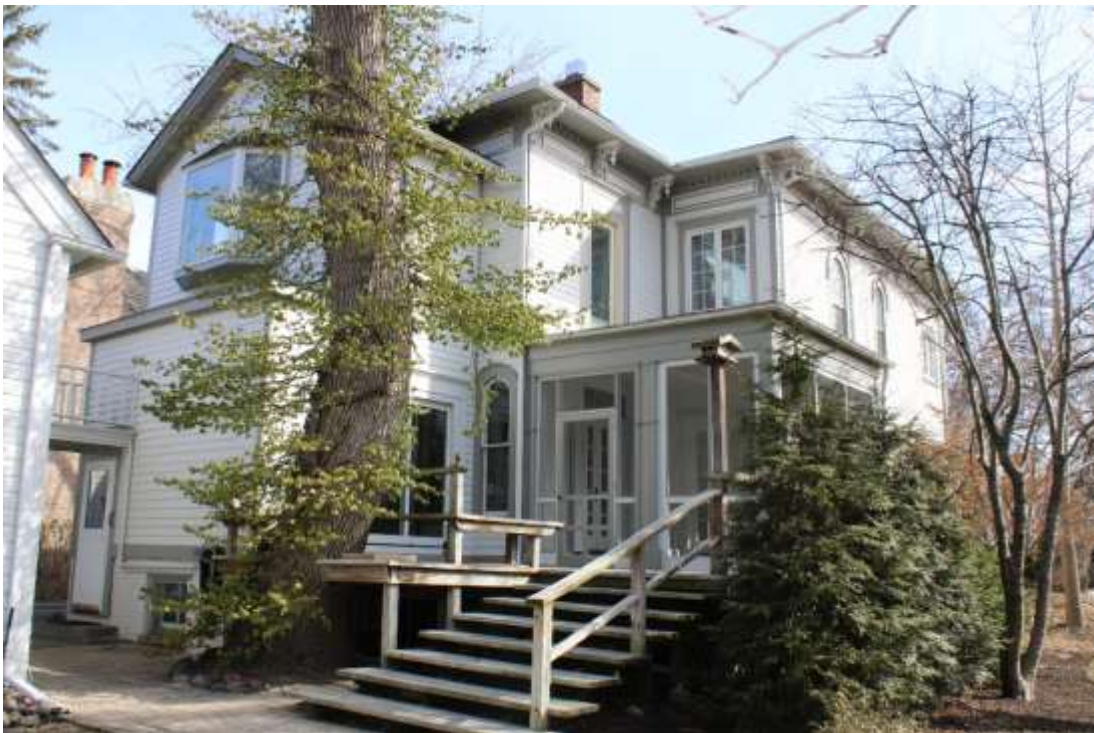
South and rear (west) facades, view northeast.
