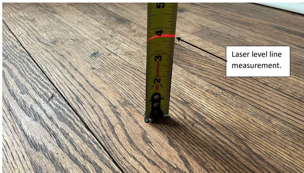
Picture 7: Northeast Bedroom South Measurement.
