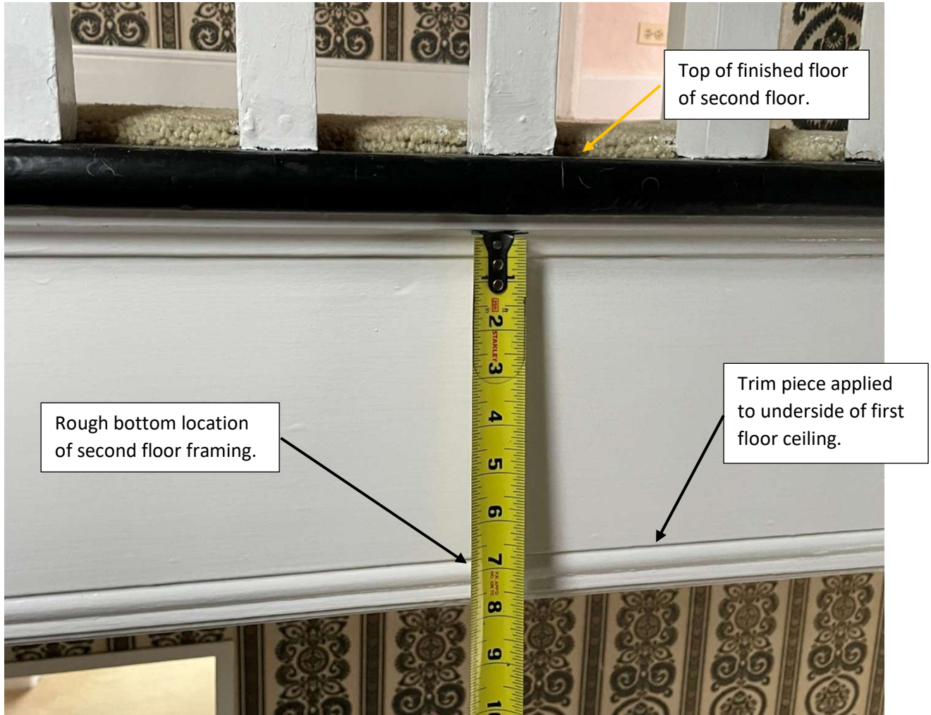
Picture 8: Rough Second Floor Framing Thickness Measurement.
