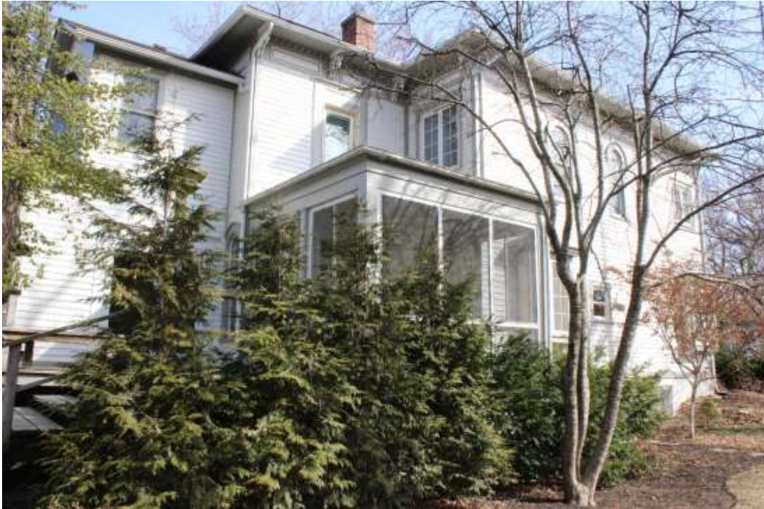
South façade, view northeast.
