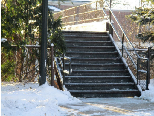
Stairs from Hubbard Place to Pedestrian Bridge, Jan 2017
