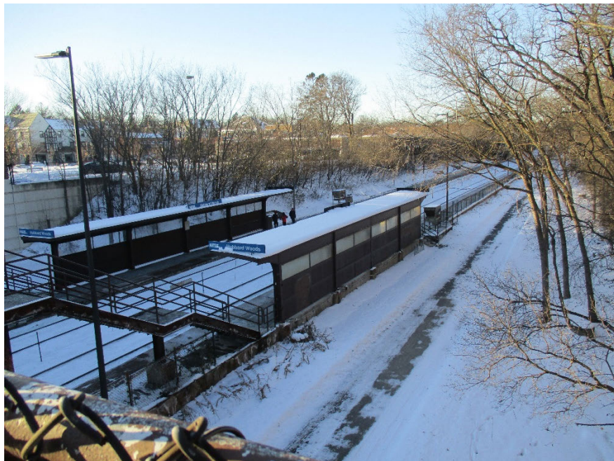
Pedestrian bridge stairs to track level, historic windbreaks, and Green Bay Trail, January 2017
