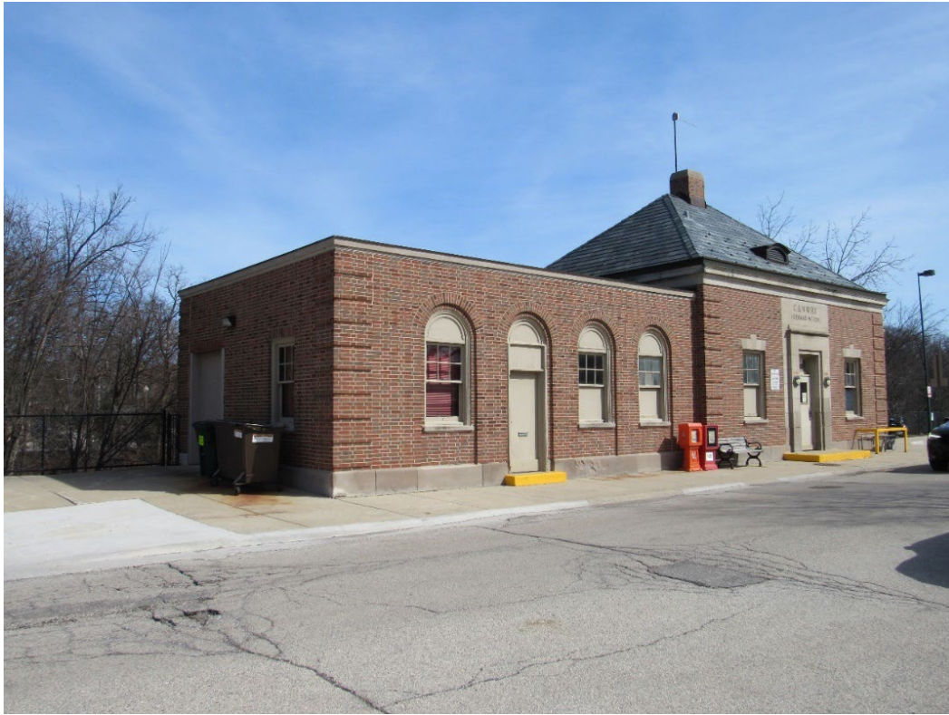
Figure 5 – Hubbard Woods Train Station – West & North Elevations
