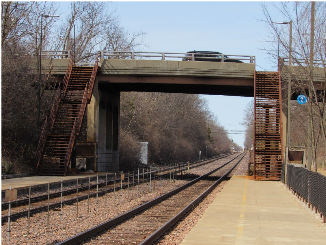
Figure 12 - Stairs from Platform to Scott Avenue
