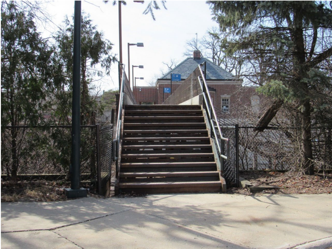
Figure 11 – Stairs from Hubbard Place to Pedestrian Bridge
