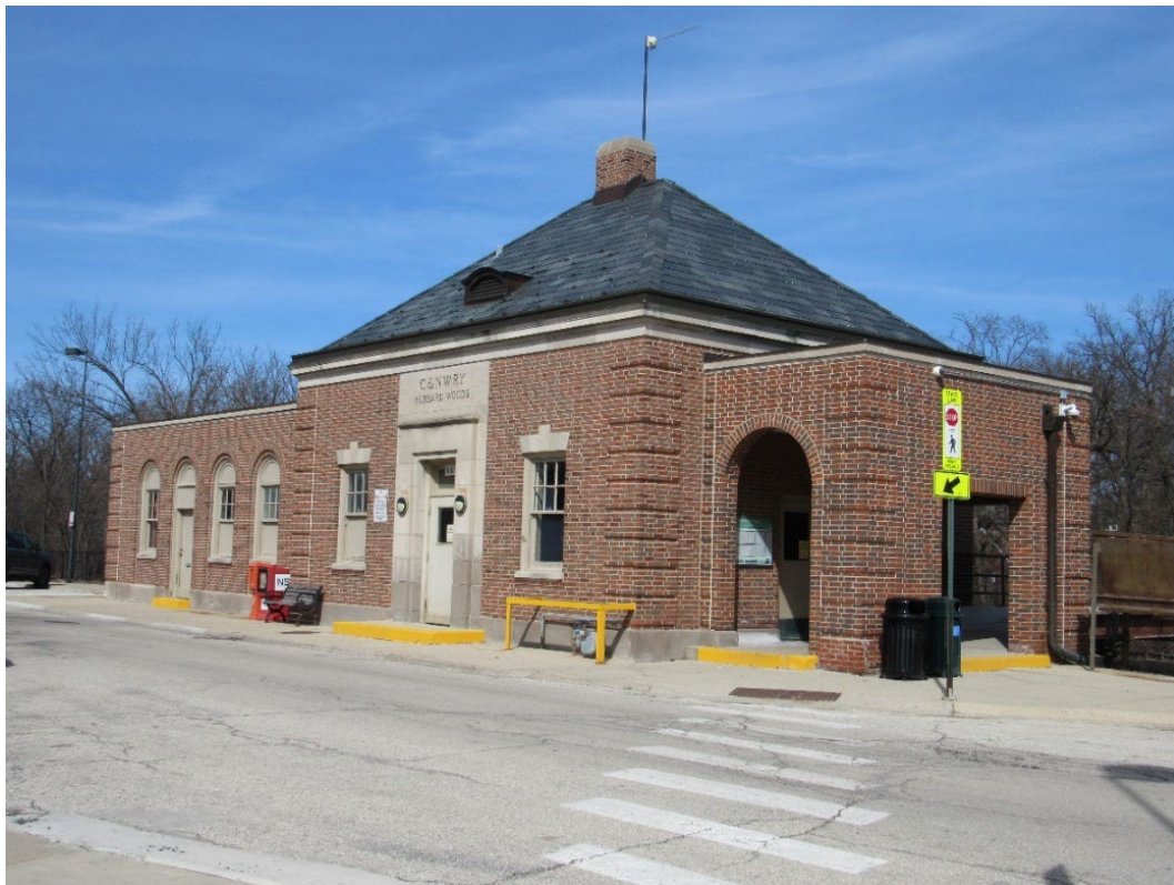
Figure 4 – Hubbard Woods Train Station – West & South Elevations
