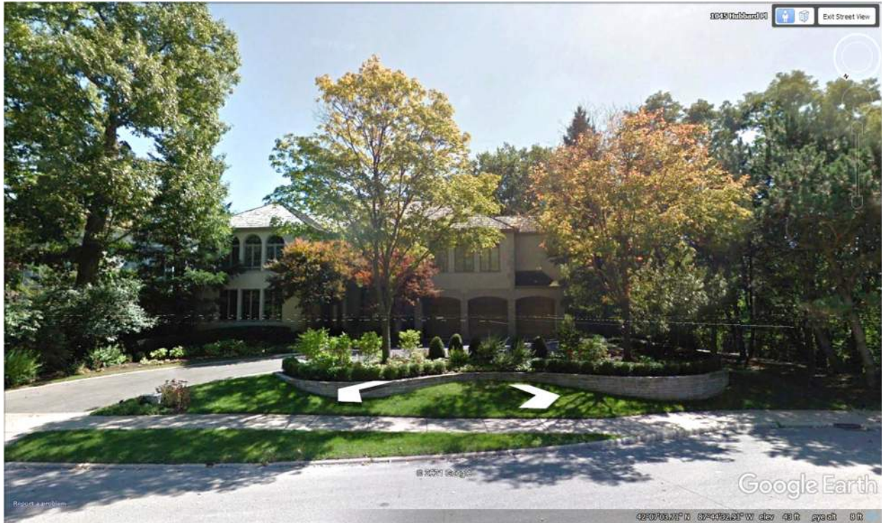
Figure 3 - Residential Dwelling at 1040 Hubbard Place, Structure is approximately 43' from pedestrian bridge and ADA ramp.
