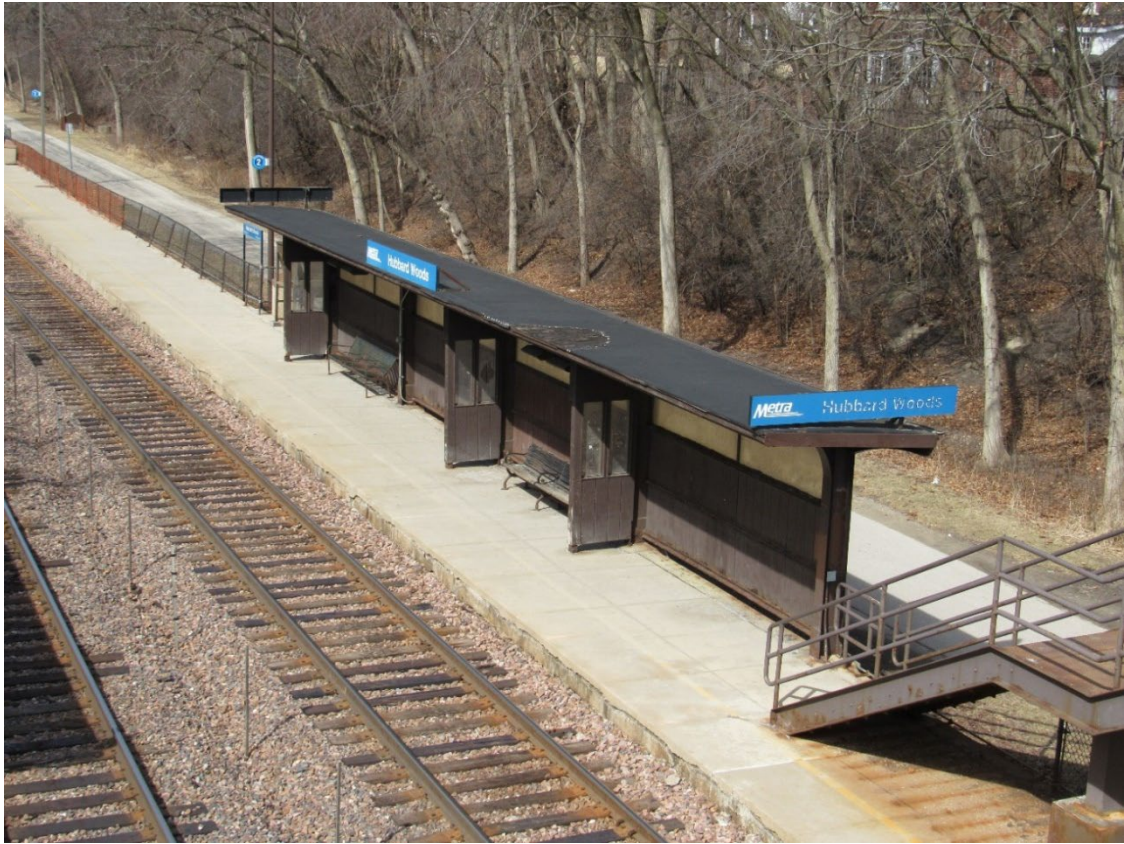
Figure 9 – East Windbreak Shelter
