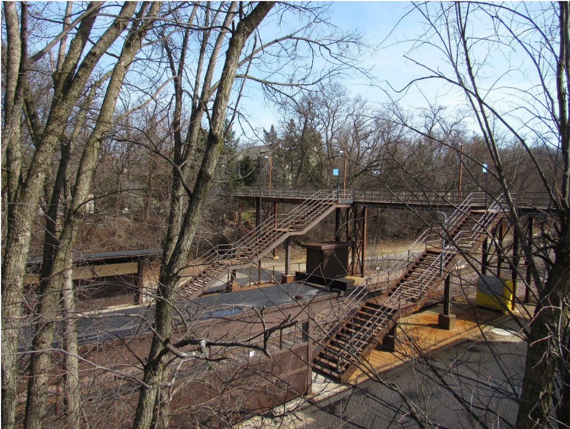
Figure 7 – Pedestrian Bridge, Stairs to Platforms & Windbreak Shelters
