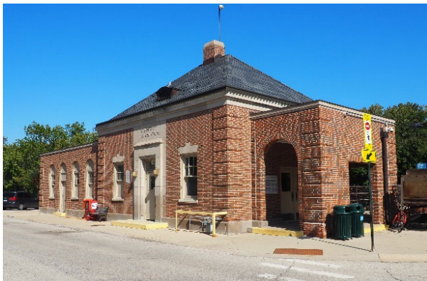
View of 1065 Gage Street, October 2019.
