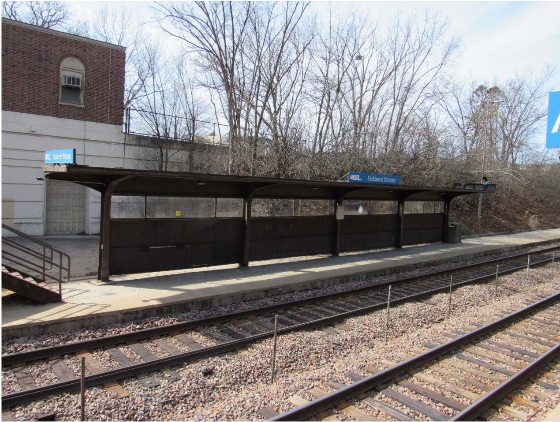
Figure 9 – West Windbreak Shelter
