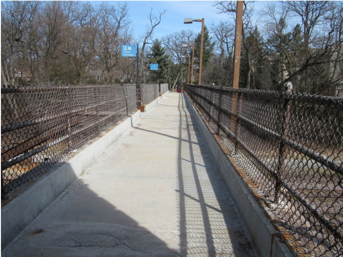
Figure 7 – Pedestrian Bridge Over Tracks
