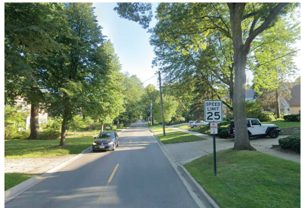
Church Road looking south.
