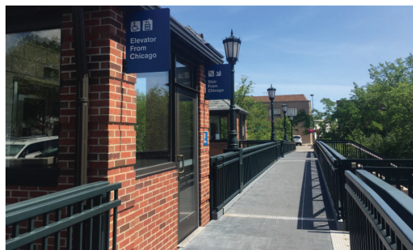
Access to elevators at Winnetka Metra Station.
