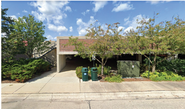
Parking deck at the Hubbard Woods Metra Station.
