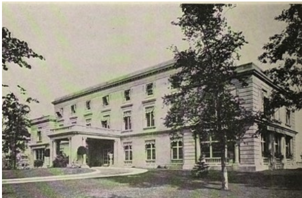
Estate House, 483 Sheridan Road, W. Façade, 1914
