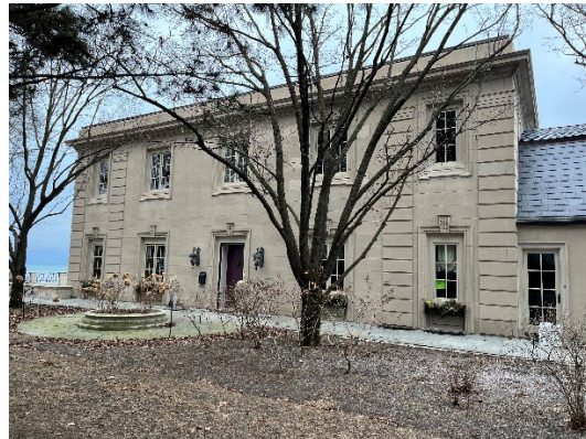
Garage, 480 Oak N. Façade, 2025 photo
