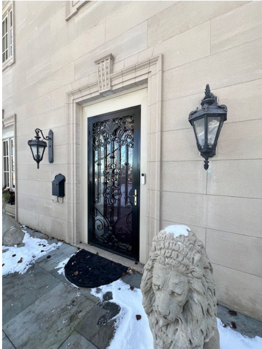
Front Entrance, North Side of House, 2025 photo
