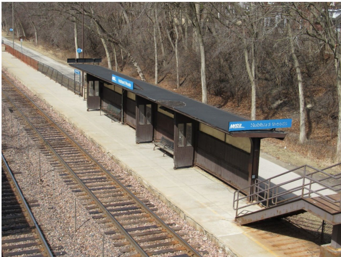
Figure 9 – East Windbreak Shelter
