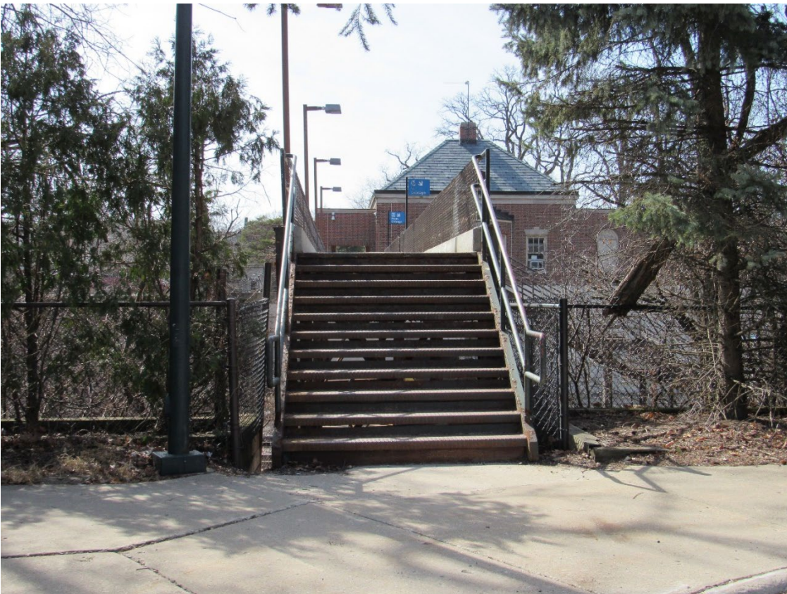
Figure 11 – Stairs from Hubbard Place to Pedestrian Bridge
