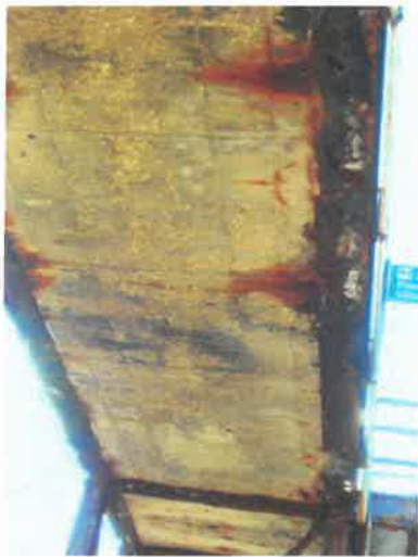
Figure 5 View below on 10/26/2014
