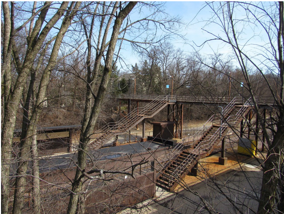
Figure 7 – Pedestrian Bridge, Stairs to Platforms & Windbreak Shelters
