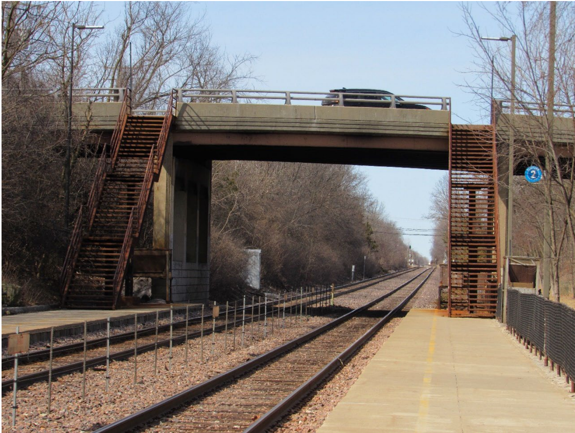
Figure 12 - Stairs from Platform to Scott Avenue
