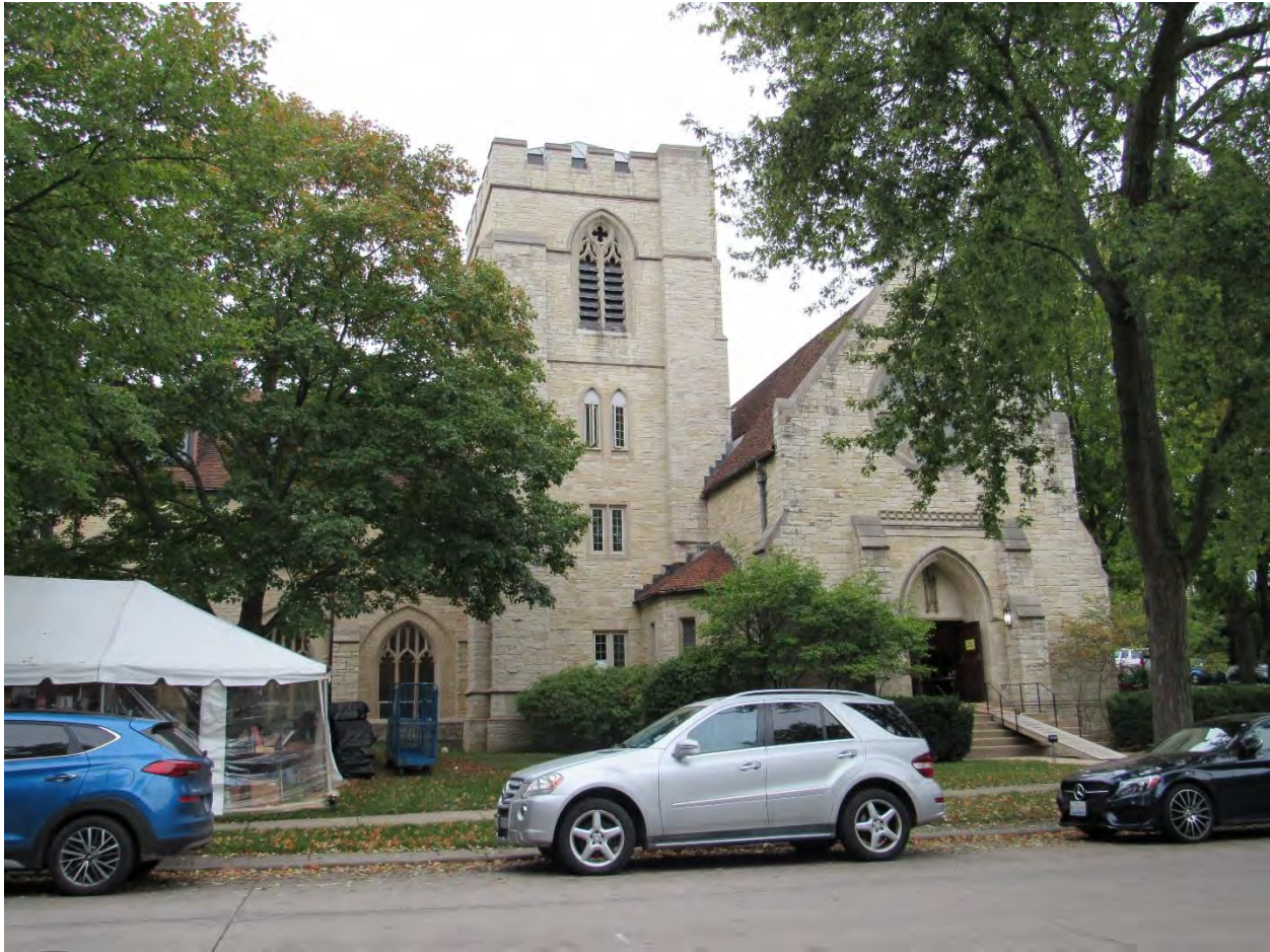
Figure 4 – East Elevation of Christ Church Chapel-Parish House
