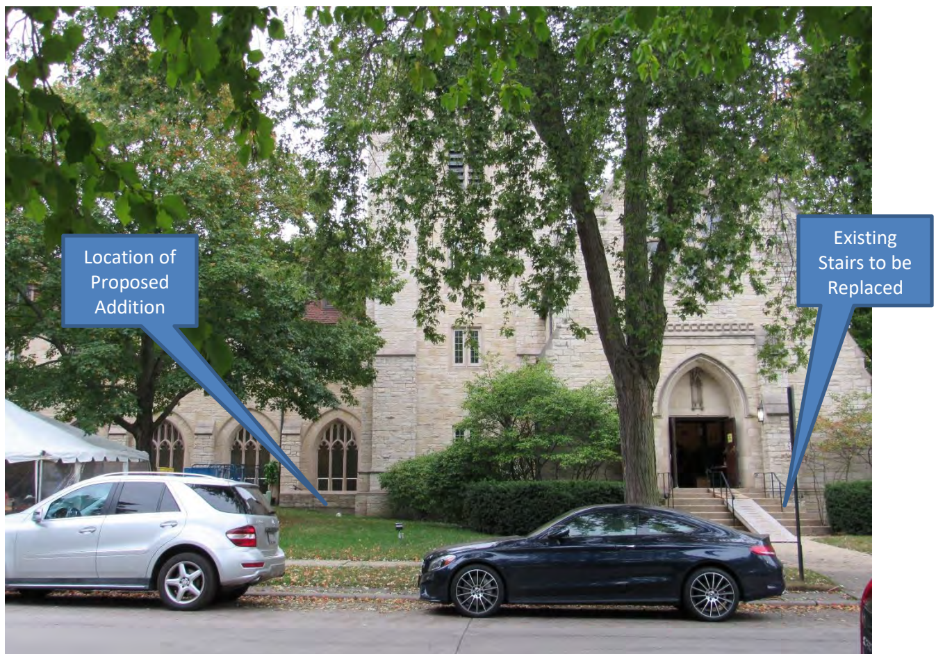
Figure 3 – East Elevation of Christ Church Chapel-Parish House
