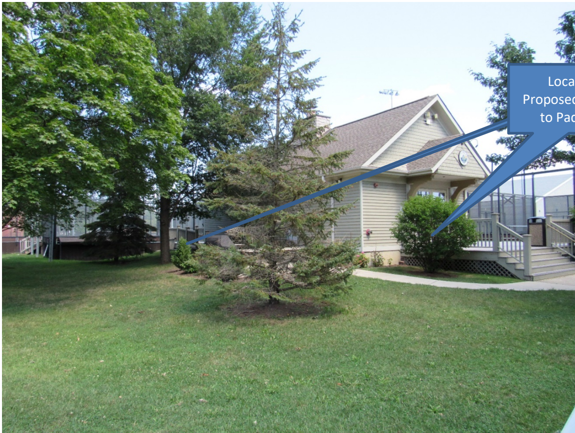
Figure 6 – Existing Paddle Hut (looking northeast)
